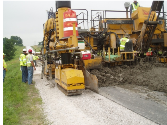
Figure 2. Slipform Paver Utilizing Stringless Paving
