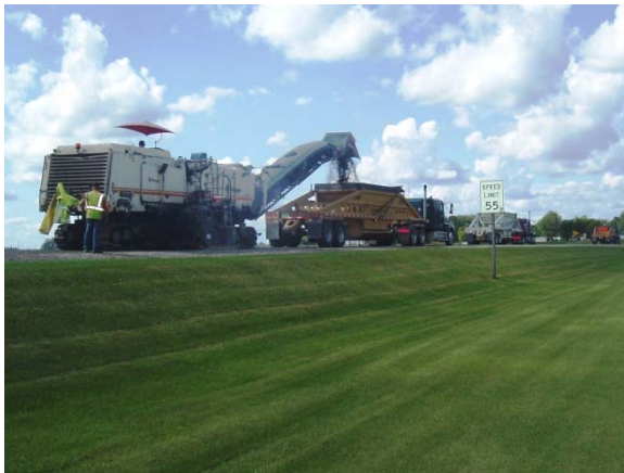
Figure 6. Mainline Pavement Milling
