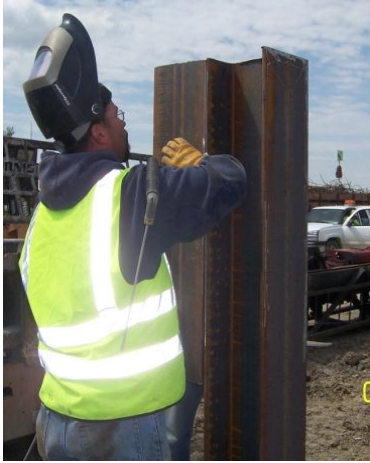
(a) Welded 40 in. short segment onto flanges
