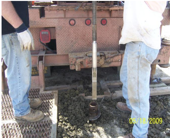
(b) Installing pressure cells
