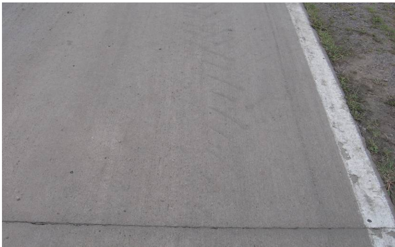
Figure 6.32. New corner break on cell 32 during fall 2010 testing
