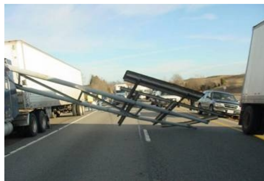
Damage to two highway structures due to high winds.
