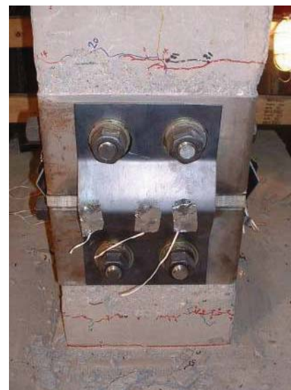
Figure 4. Segment joint after testing
