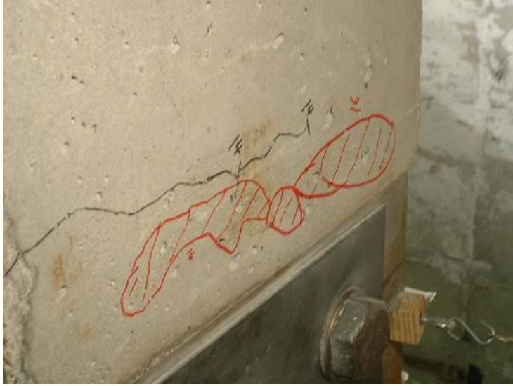
a.) Upper segment compression damage
