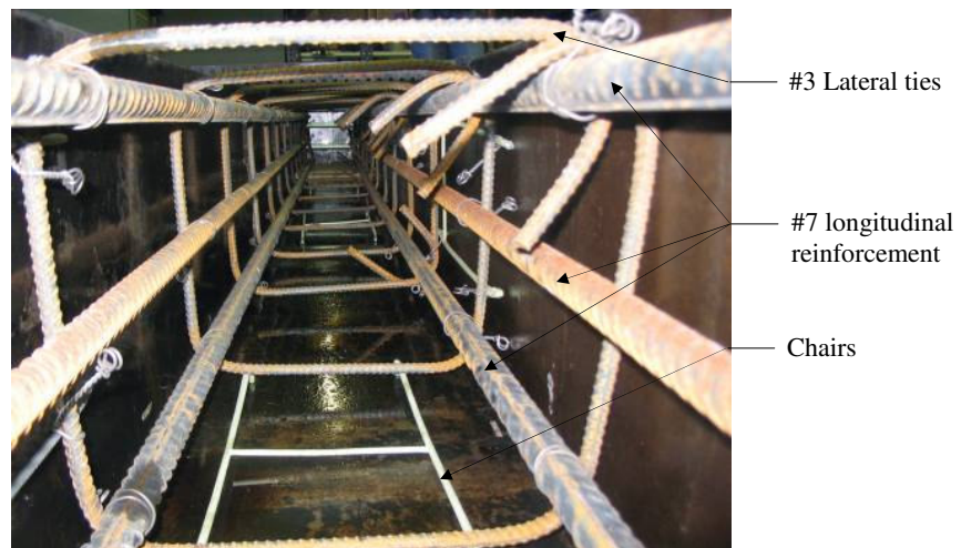
Figure 31. Photograph of chairs and reinforcement in Column 1.
