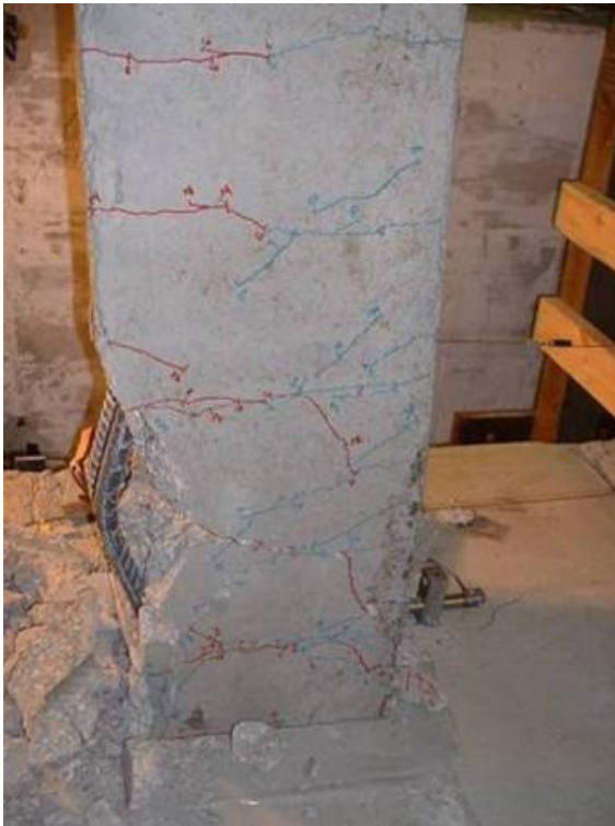
c.) North face cracking/bulging
