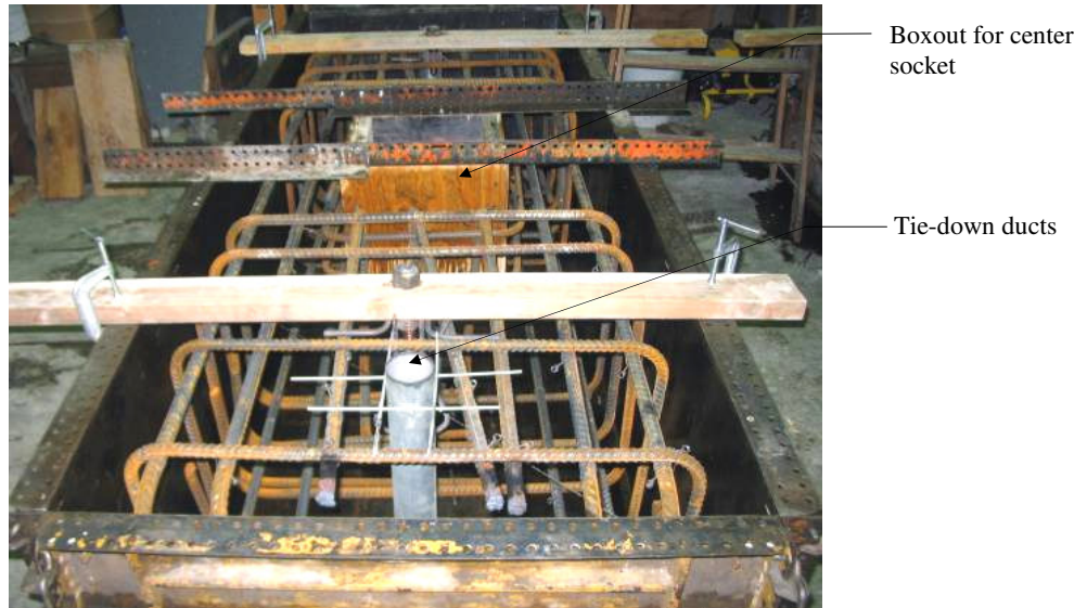
Figure 28. Photograph of foundation reinforcement and tie-down ducts in forms.
