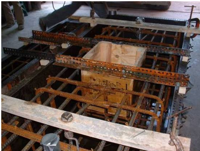
Figure 49. Photograph of Column 3 foundation reinforcement in forms.
