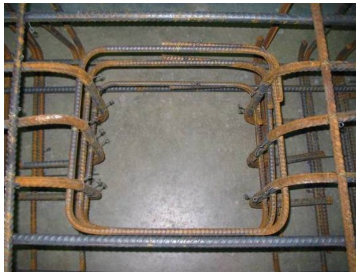
Figure 25. Photograph of center socket reinforcement.
