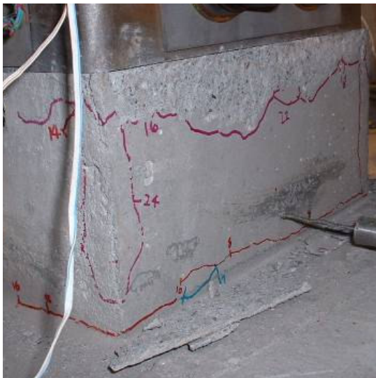
a.) Lower segment east face spalling
