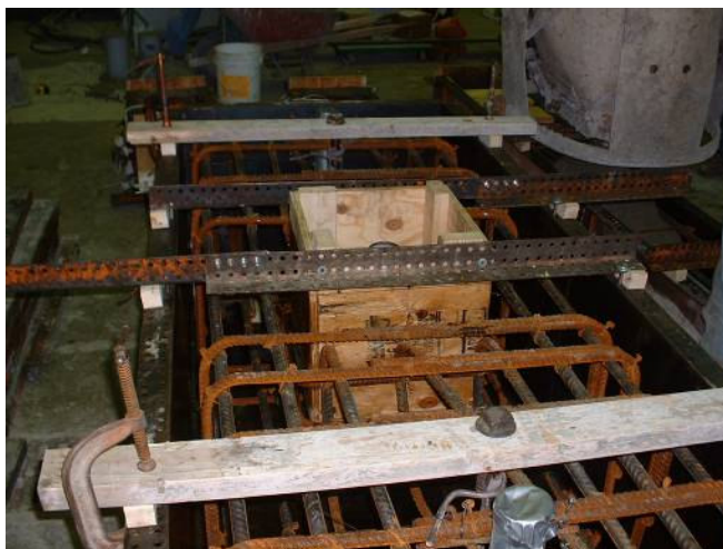
Figure 50. Photograph of Column 4 foundation reinforcement in forms.
