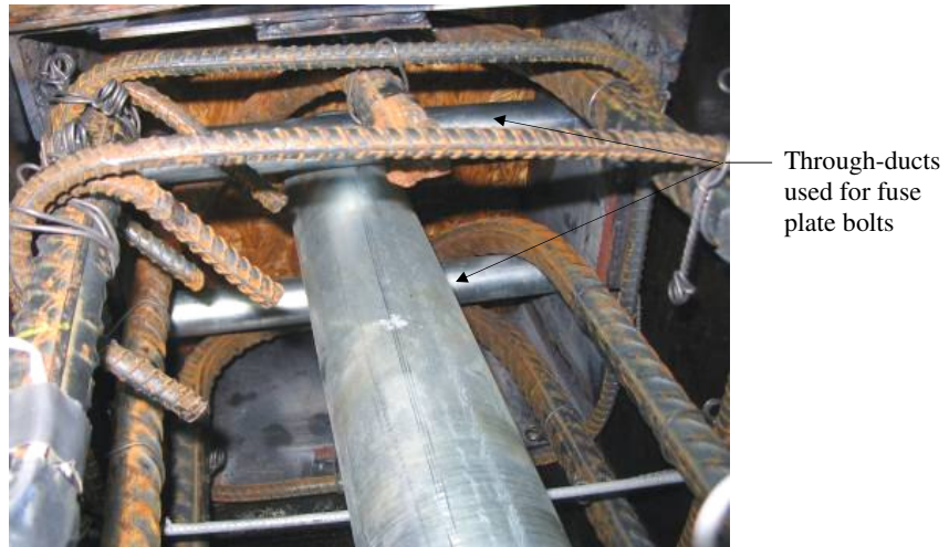
Figure 35. Photograph of Column 2 collar end.
