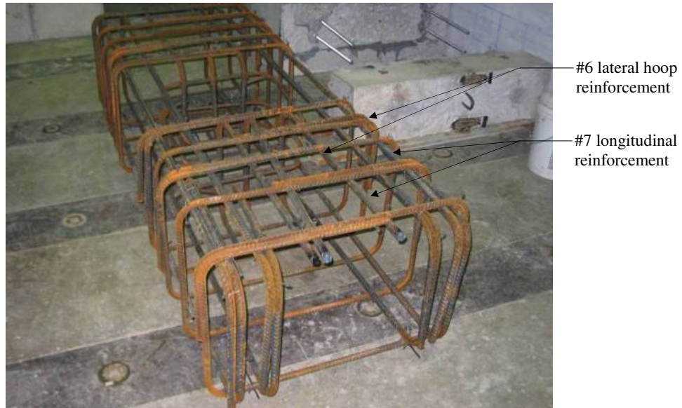
Figure 26. Photograph of foundation reinforcement cage.
