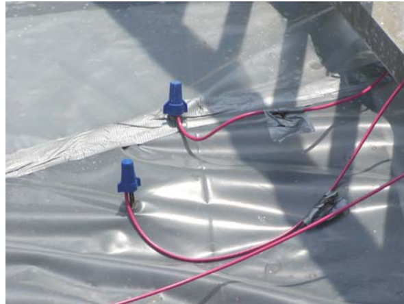
Figure 11 Electrical Connections to the Deck Rebar
