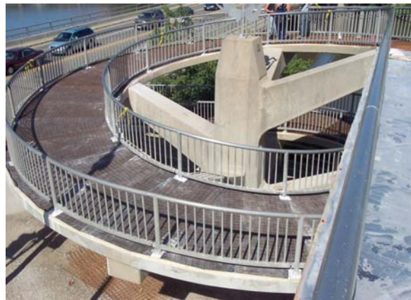
Figure 9 Steel Mats Placed on the Spiral Ramps to the Deck
