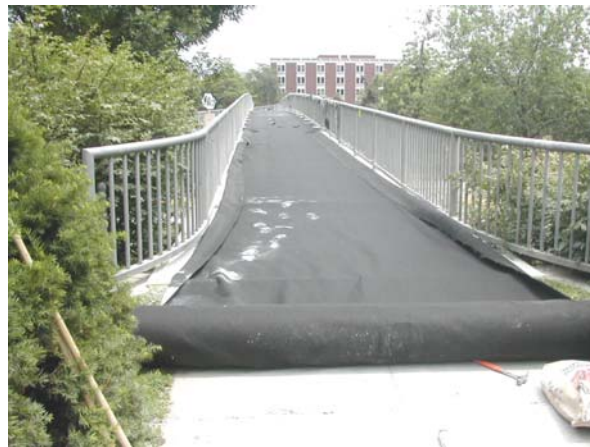
Figure 7 Felt Mat Placed on the Deck
