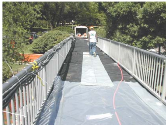
Figure 10 Soaker Hoses & Plastic Sheets Placed on the Felt
