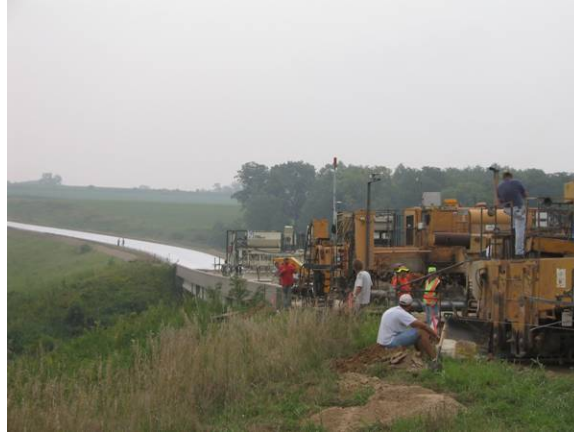
Figure 3. Slip-form Paving Machine Being Reconfigured to Cross Narrow Bridge
