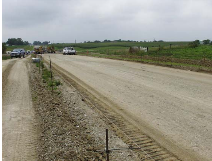
Figure 1. Stakes and String Line for Concrete Road Paving
