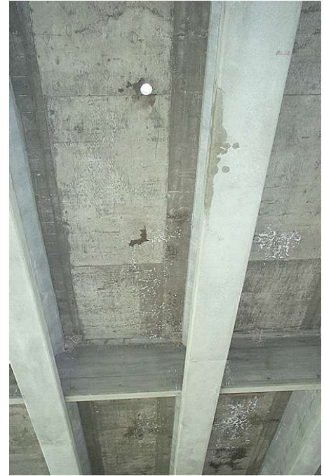
Figure 7. Photographs of core site (left) and from beneath bridge deck (right) after coring operation.
