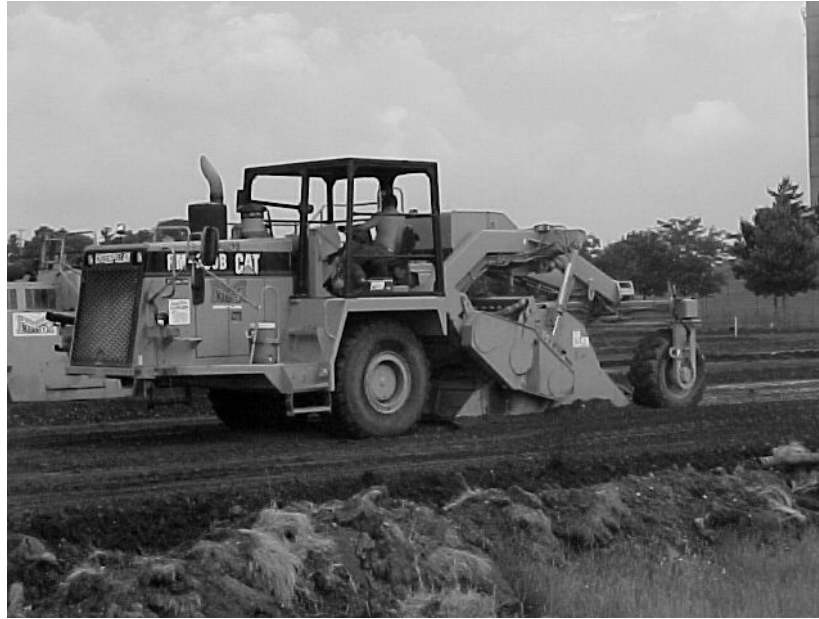
Figure 1. Pulvamixer used for on-site mixing
