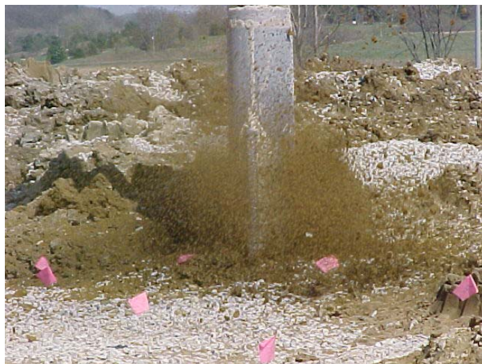
Figure 17. Stone Column Construction Operations
