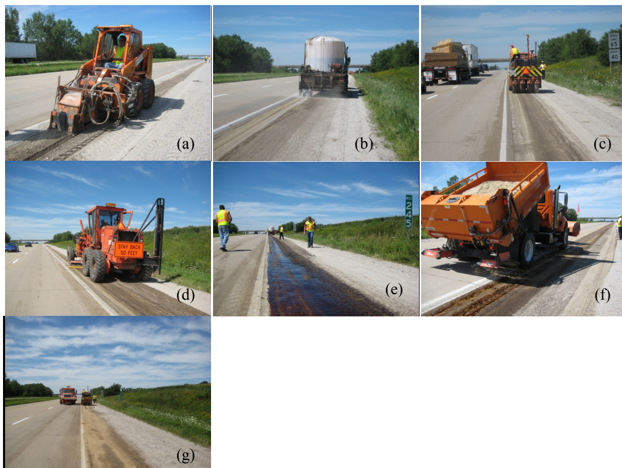
Figure 83. Section III: a) shoulder scarification, b) moisturizing, c) roller compaction, d) surface grading, e) DUSTLOCK application, f) sand spraying, and g) roller compaction August 18, 2009
