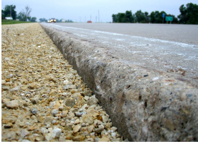
Figure 2. Shoulder drop-off Highway 63 milepost 172.5 northbound June 4, 2008
