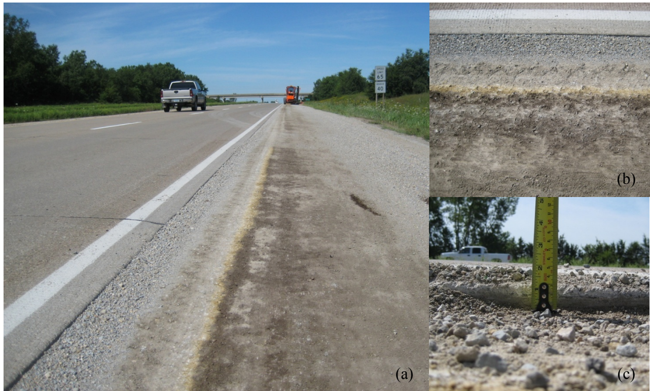
Figure 82. Section III: a) graded surface, b) side view of graded surface, and c) pavement edge drop off August 18, 2009
