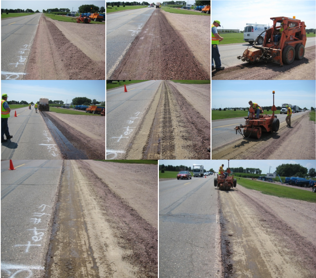
Figure 54. Stabilization procedure of Test Area I Section II on southbound shoulder of US 75 near Sioux Center, Iowa July 29, 2009
