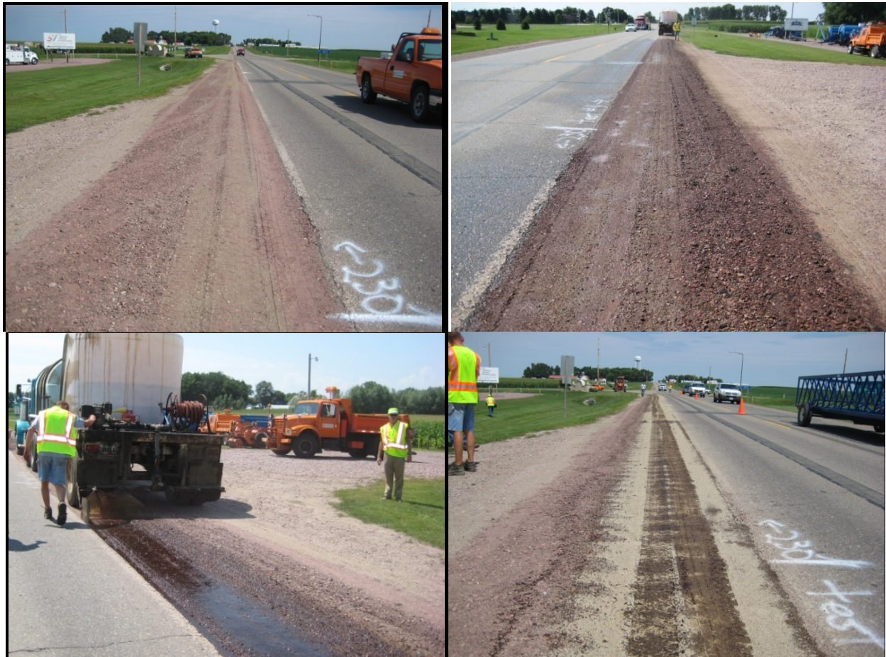
Figure 53. Stabilization procedure of Test Area I Section I on southbound shoulder of US 75 near Sioux Center, Iowa July 29, 2009
