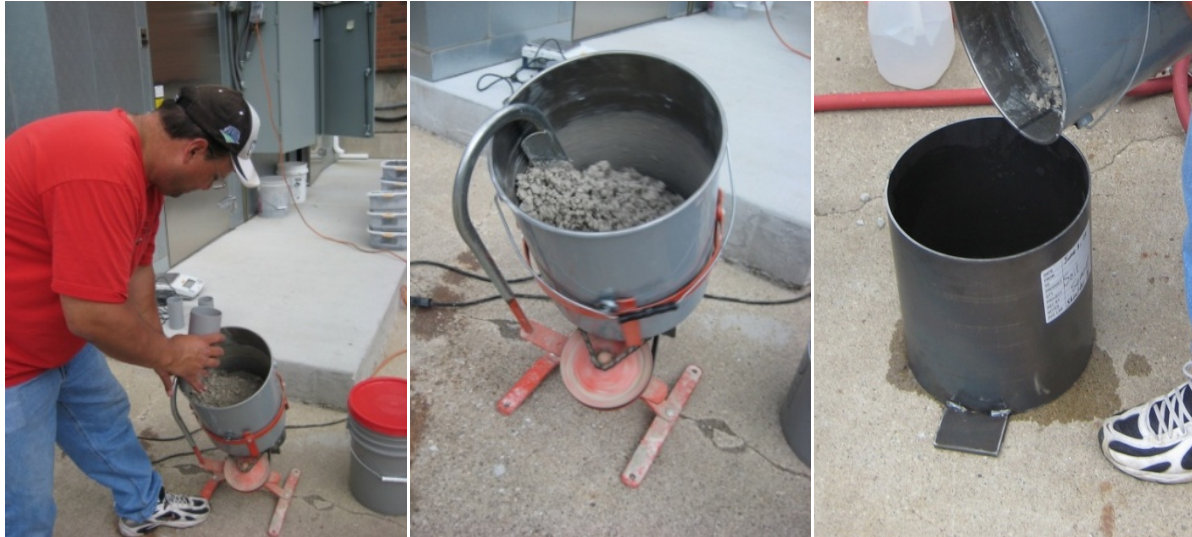
Figure 33. Preparation of one batch of aggregate/stabilizing agent mixture
