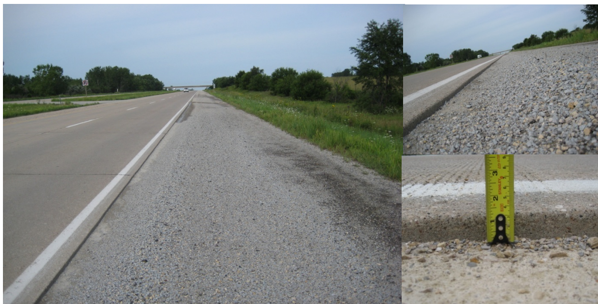
Figure 72. Shoulder conditions and edge ruts along the pavement slabs August 17, 2009
