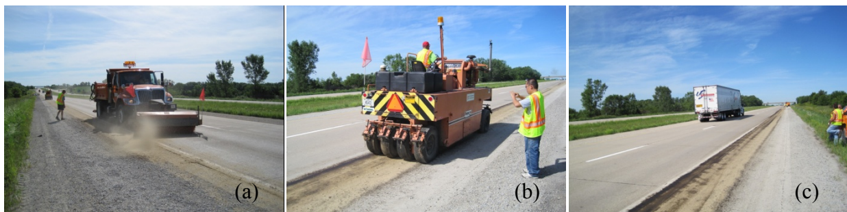
Figure 80. Section II: a) pavement cleaning, b) compaction, and c) finished surface August 18, 2009
