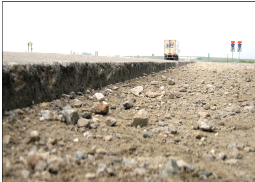
Figure 1. Shoulder drop-off near pavement edge Highway 18 milepost 195.95-196.2 westbound June 4, 2008
