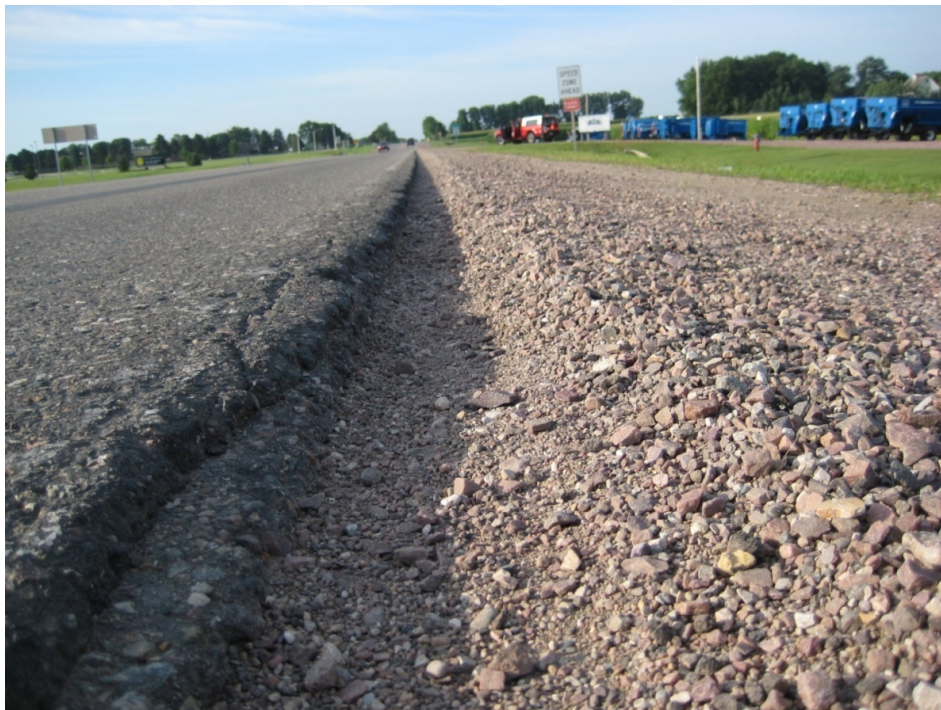
Figure 50. Shoulder rutting at Test Area I before stabilization July 28, 2009
