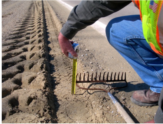
Figure 16. Pickup truck tire rut that indicated the typically soft conditions one day after full-depth reclaiming
