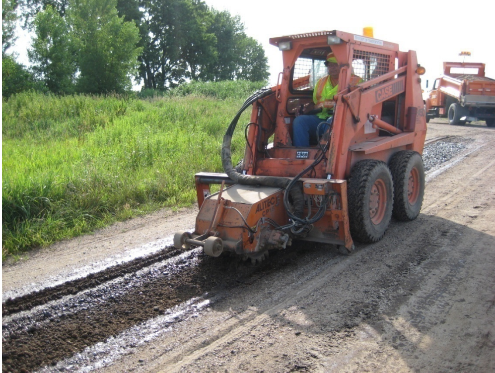
Figure 45. Mixing aggregate material with the stabilizing agent
