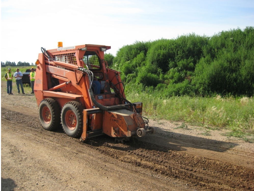
Figure 43. Scarifying ground surface using a milling machine
