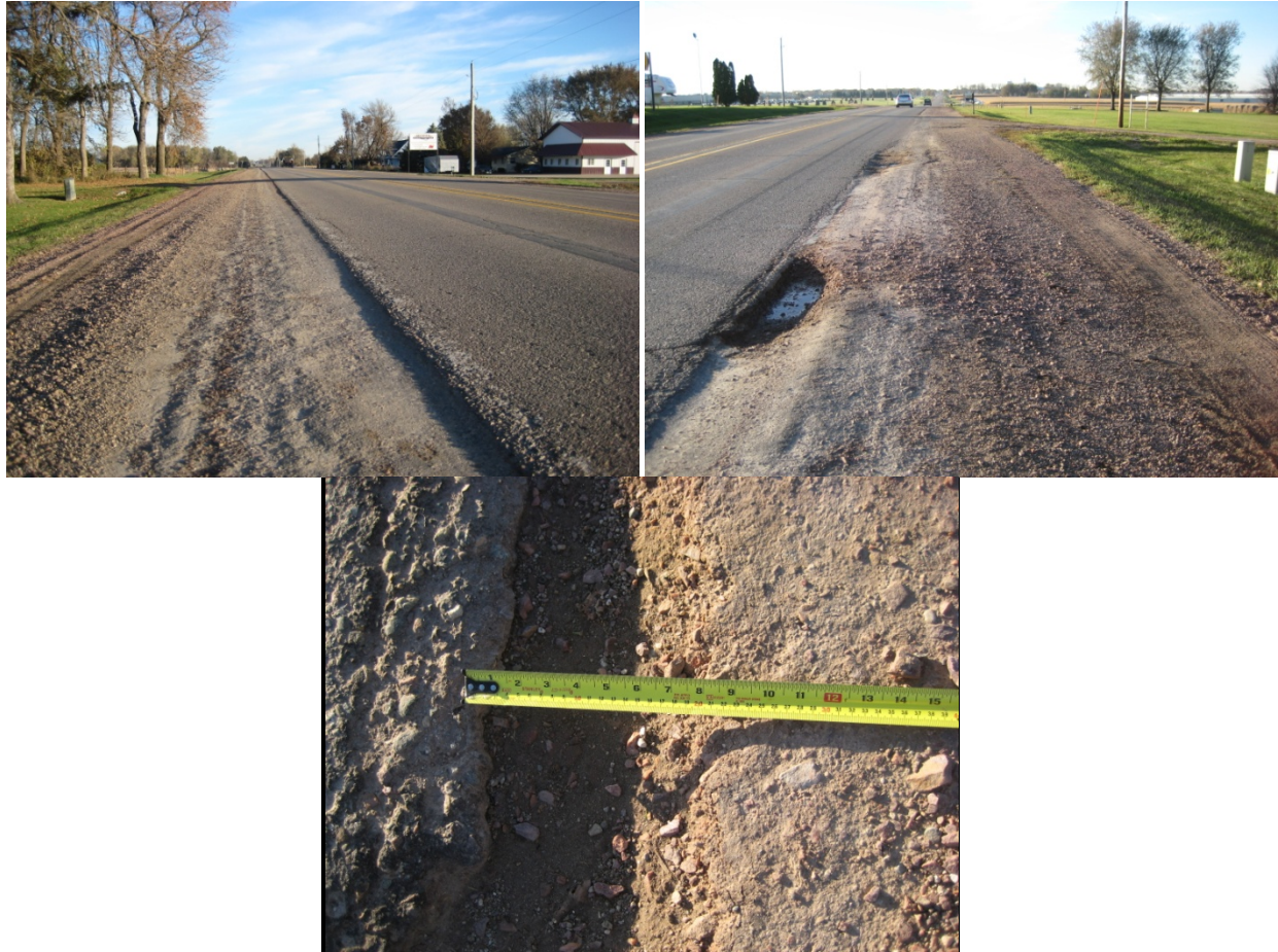
Figure 68. Shoulder condition of the Test Area III on the southbound shoulder of US 75 near Sioux Center, Iowa October 27, 2009
