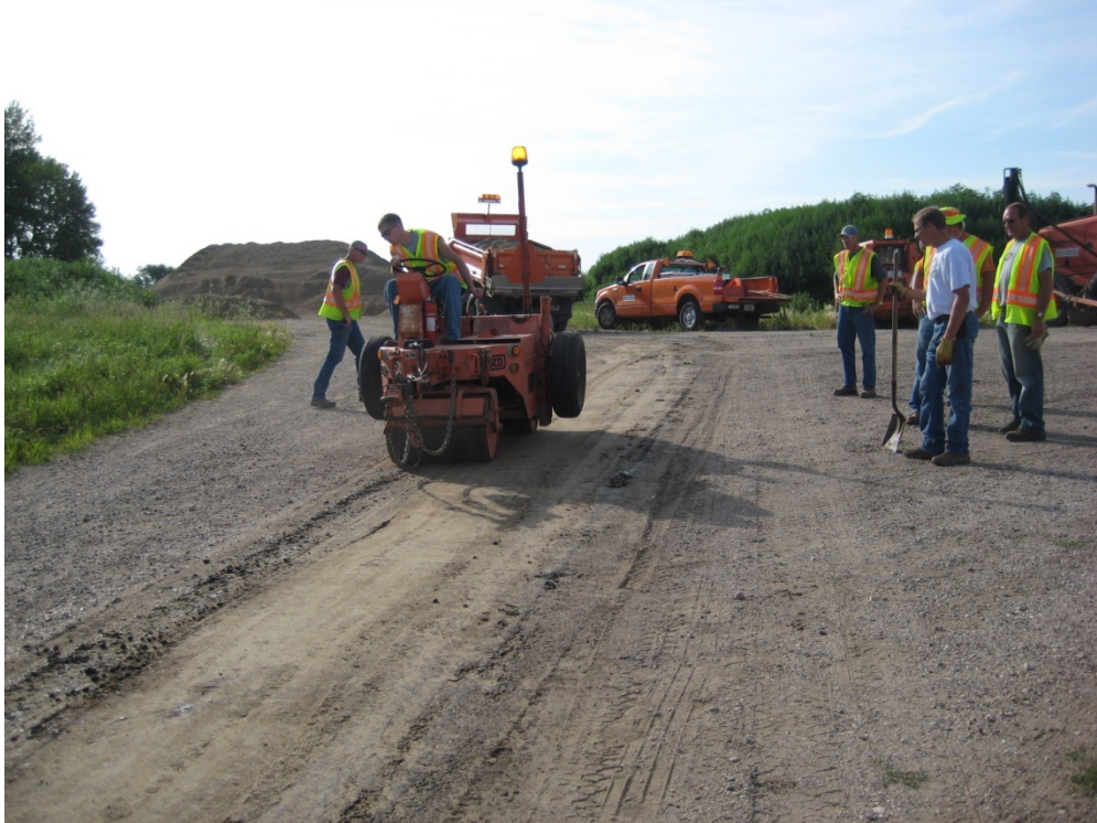
Figure 47. Compaction using a smooth roller
