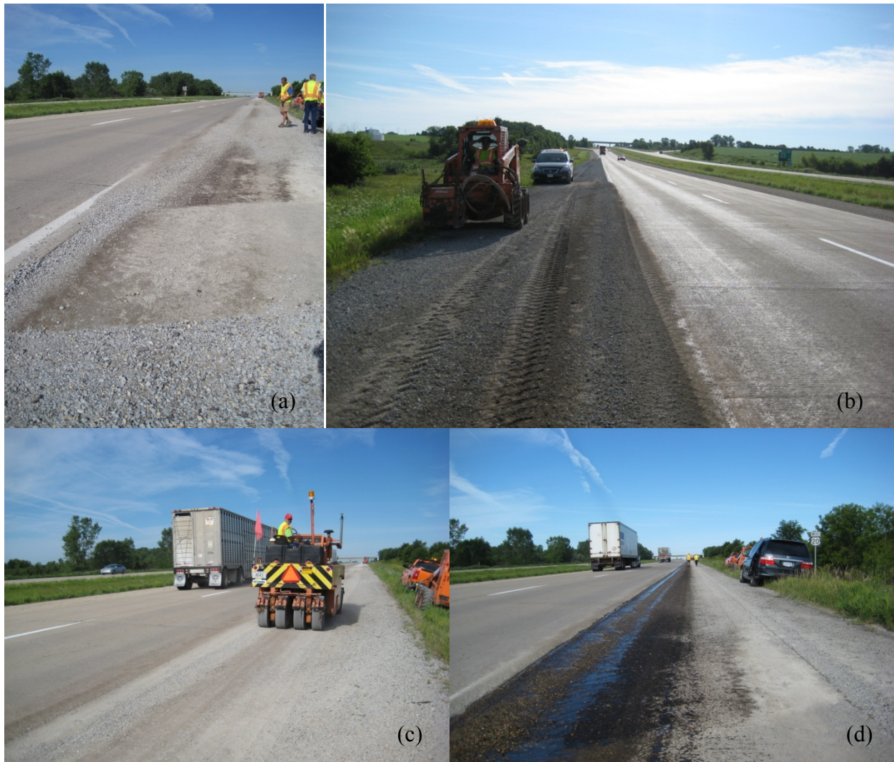
Figure 79. Section II: a) grading, b) filling and leveling, c) compaction, and d) application of DUSTLOCK August 18, 2009
