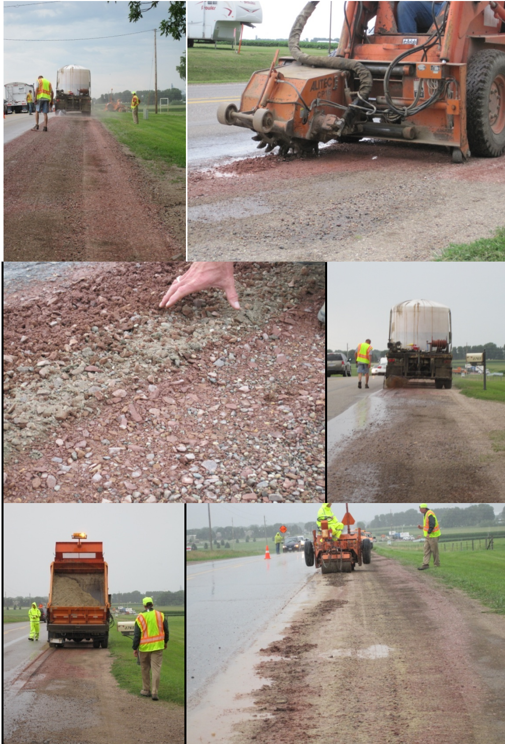
Figure 65. Stabilization procedure of Test Area III on southbound shoulder of US 75 near Sioux Center, Iowa July 29, 2009
