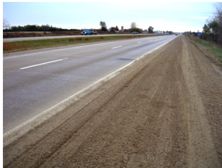
Figure 17. Magnesium chloride full-depth after one week
