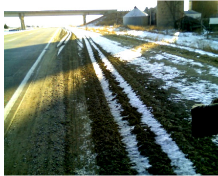
Figure 20. Rutting on Control Section 1 in February
