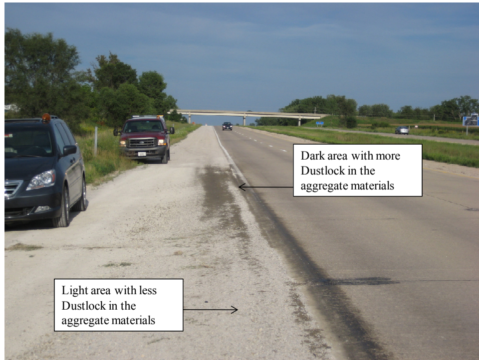
Figure 86. Uneven mixed of DUSTLOCK due to grading process in Section V August 18, 2009
