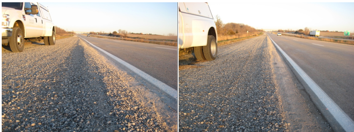
Figure 89. Stabilized shoulder using DUSTLOCK on US 20 westbound covered with course aggregate beyond edge-rut area November 7, 2009
