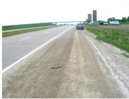
Figure 21. Mostly good calcium chloride full-depth 8 ft wide June 2009
