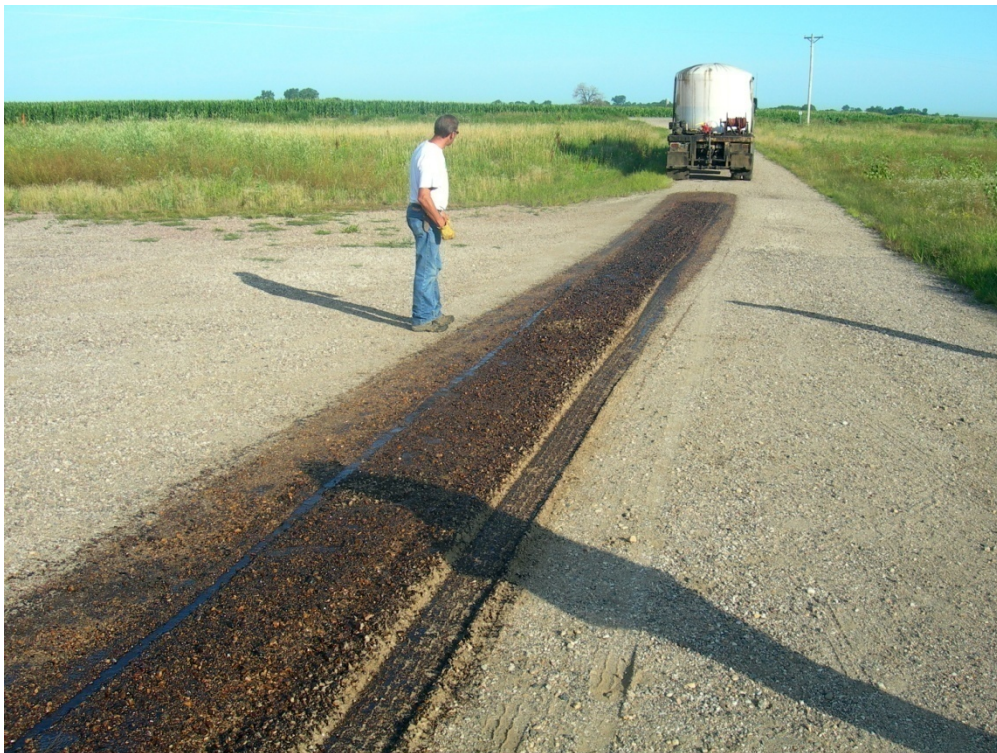
Figure 44. Spraying of the stabilizing agent on the scarified surface
