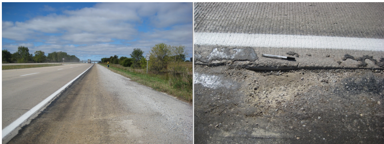
Figure 87. Stabilized shoulder using DUSTLOCK on US 20 westbound September 29, 2009
