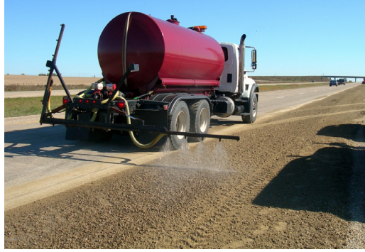
Figure 9. Distributor truck spraying calcium chloride on shoulder surface
