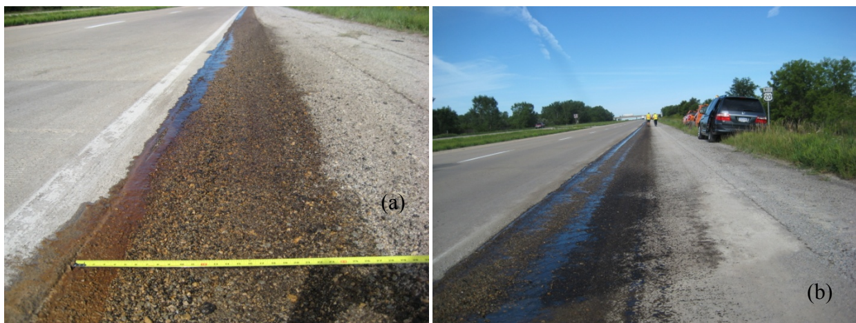
Figure 76. Topical application of DUSTLOCK: a) 2 ft (0.6 m) strip (sprayed with one tip) and b) 4 ft (1.2 m) strip (sprayed with two tips) August 18, 2009
