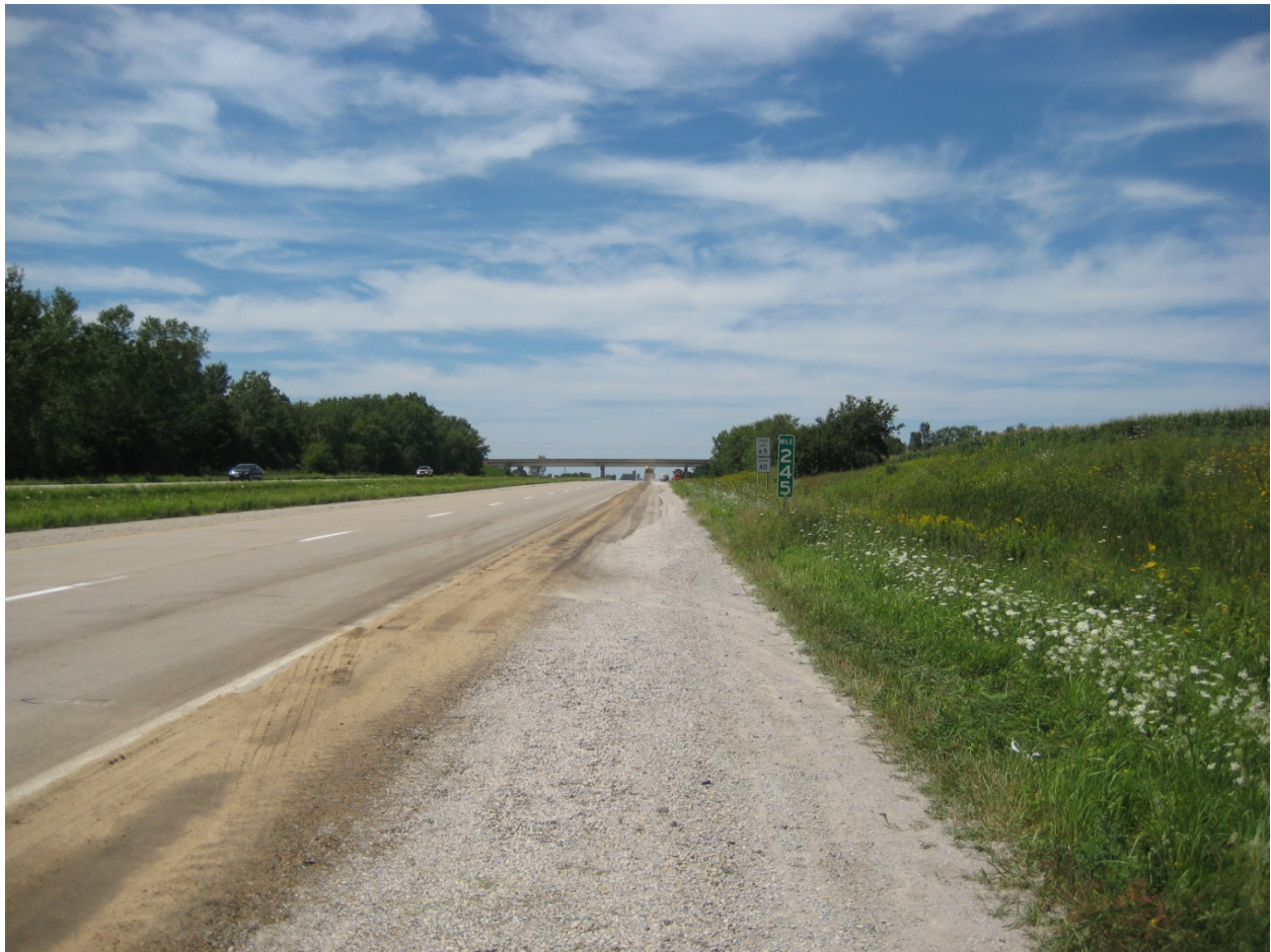
Figure 84. Stabilized shoulder surface of Sections II to IV (a) August 18, 2009
