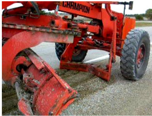
Figure 10. Road grader scarifying shoulder material
