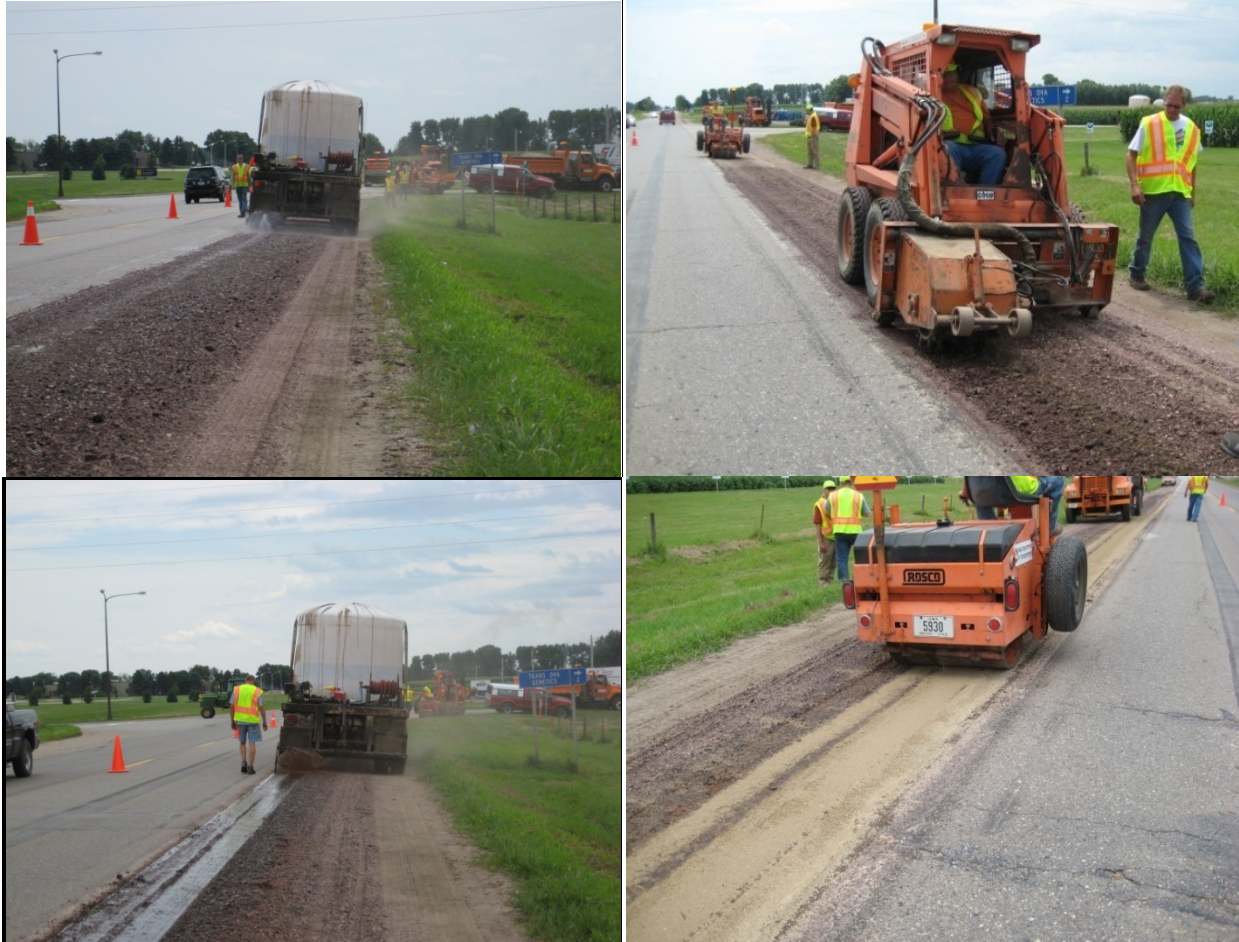
Figure 60. Stabilization procedure of Test Area II on southbound shoulder of US 75 near Sioux Center, Iowa July 29, 2009
