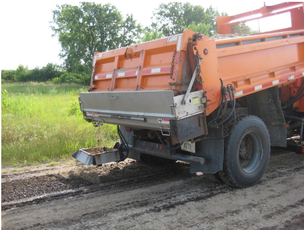
Figure 46. Sand broadcasting
