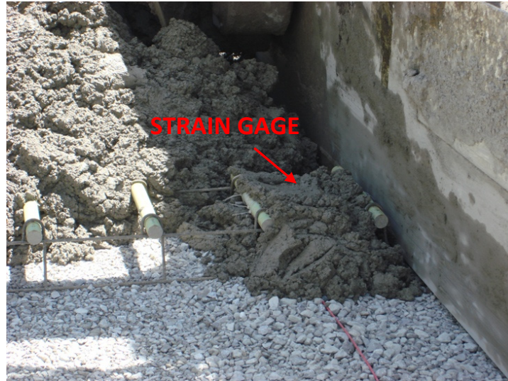
Figure 12. Strain gages during paving
