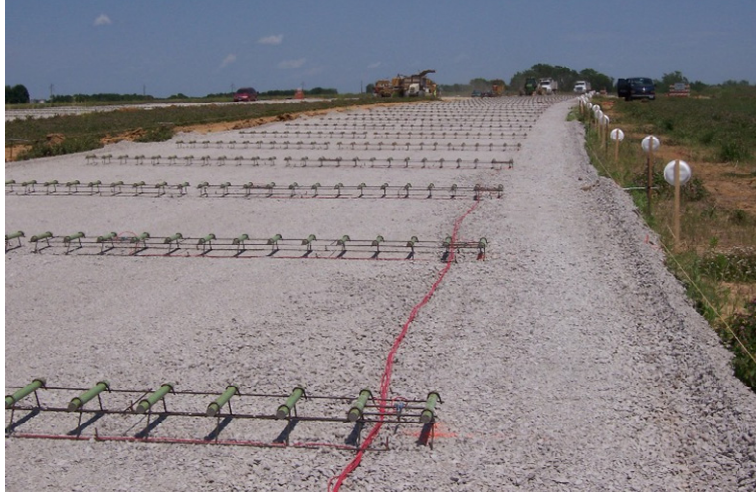
(a) Arrangement of strain gages and cables
