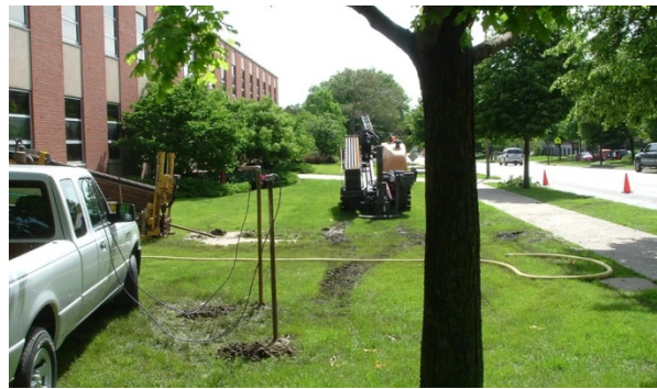
Figure 4.104. Bore seen approaching the two pressure cells (left)
