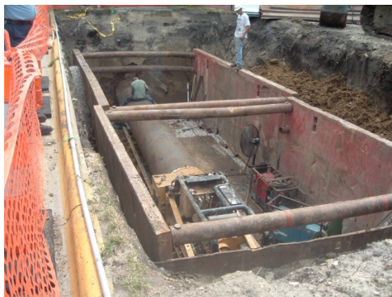
Figure D.15. First casing being bored from the launching pit
