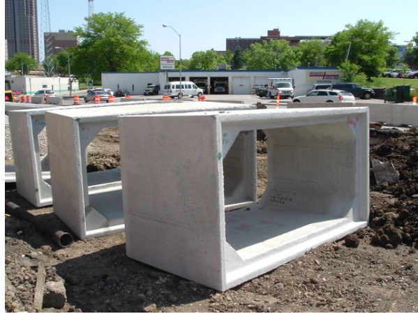
Figure 4.14. Segments of 10-foot by 5-foot RCBCs
