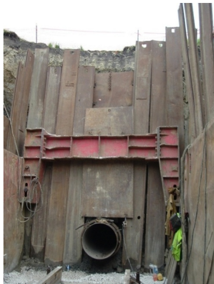
Figure 4.31. Protruding casing after boring is finished
