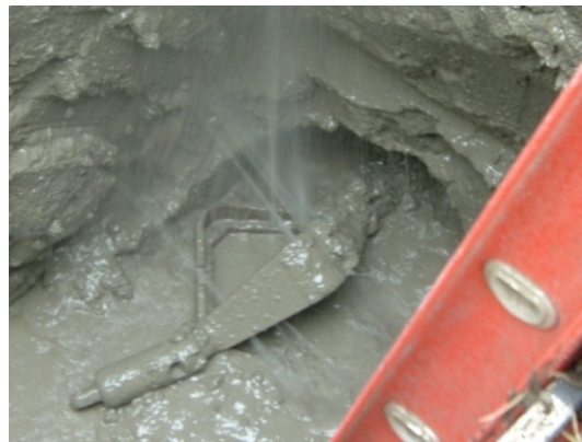
Figure 4.41. Reamer shown jetting drilling fluid in point D exit pit just before pullback
