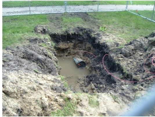
Figure 4.98. HDPE pipe (8-inch diameter) capped at point C after installation from points C to D; locate wire visible
