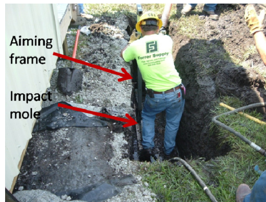
Figure 4.110. Launching the mole and adjusting line and grade using telescopic aiming frame
