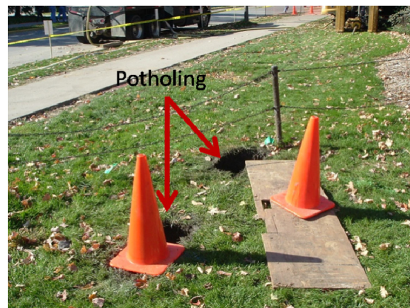
Figure 4.59. Potholing to verify position of nearby utilities
