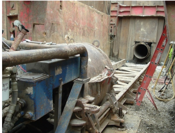
Figure 4.30. Launching pit before a new 20-foot pipe section is lowered into place
