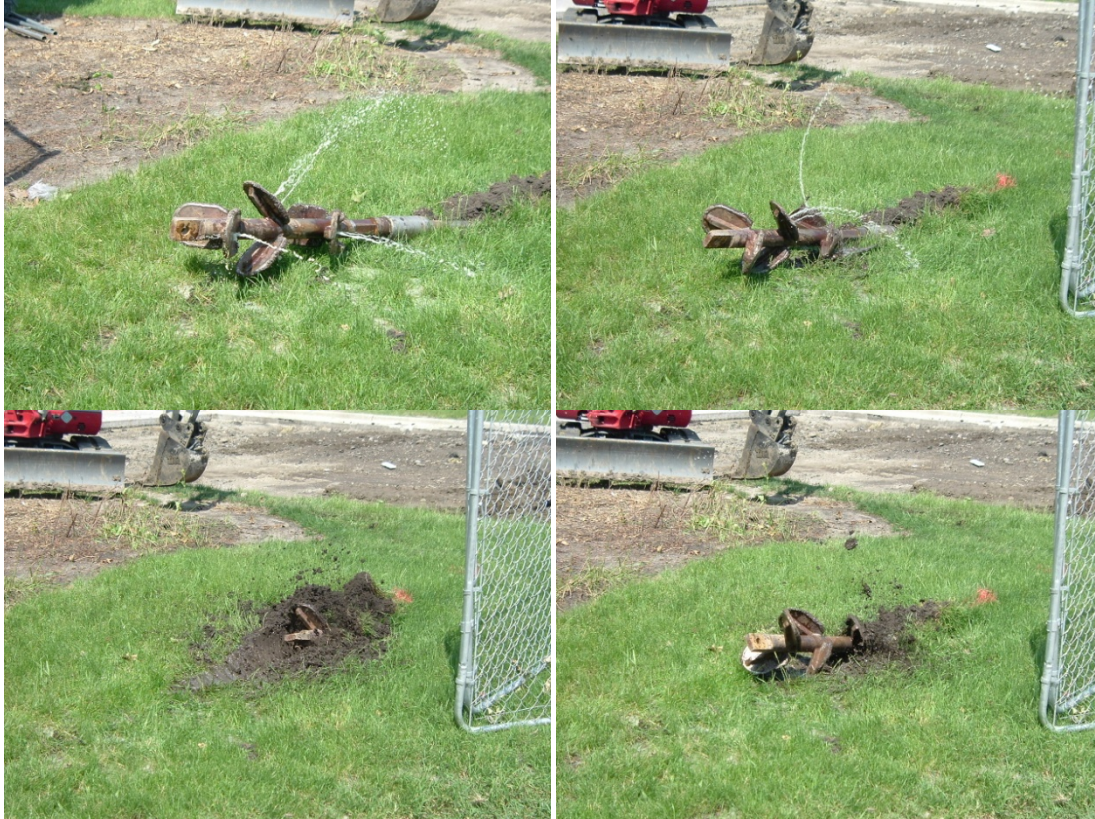
Figure 4.101. Reamer (14-inch diameter) pulled into borehole at point A (clockwise from upper left)
