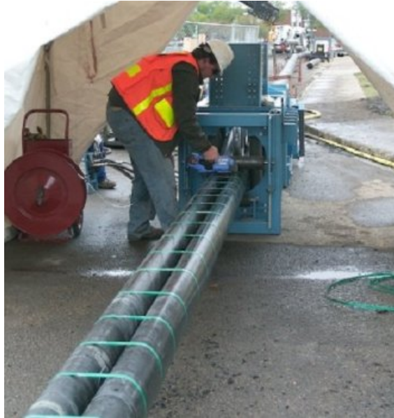
Figure 2.26. Close-fit pipe (Insituform Technologies Inc.)
