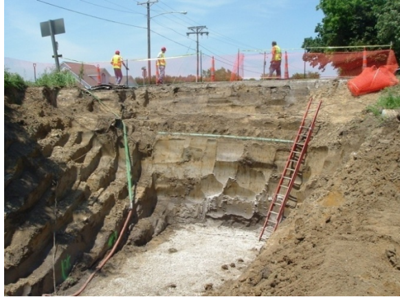
Figure D.3. Launching pit with terraced sides and a gravel base
