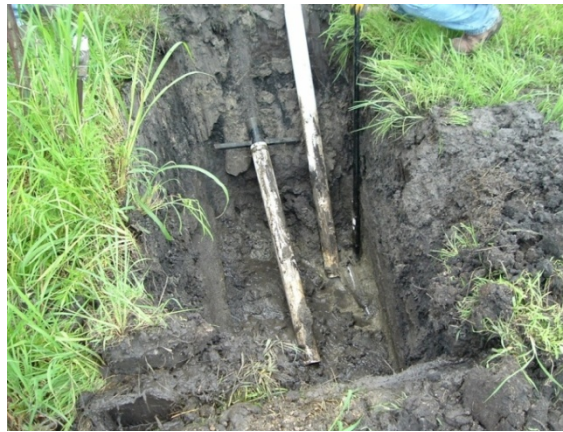
Figure 4.112. Exit pit at point C dewatered to allow retrieval of the mole
