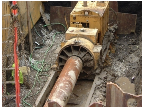
Figure D.11. Pipe and auger boring machine as a new pipe segment is being fitted to the machine and welded to the pipeline
