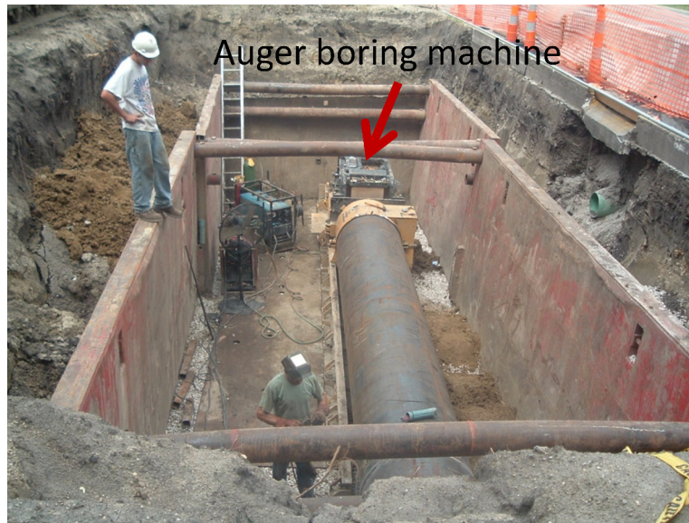
Figure 2.2. Launching pit with auger boring machine installing pipe
