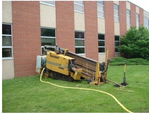
Figure 4.96. Directional drilling machine drilling from point C to D
