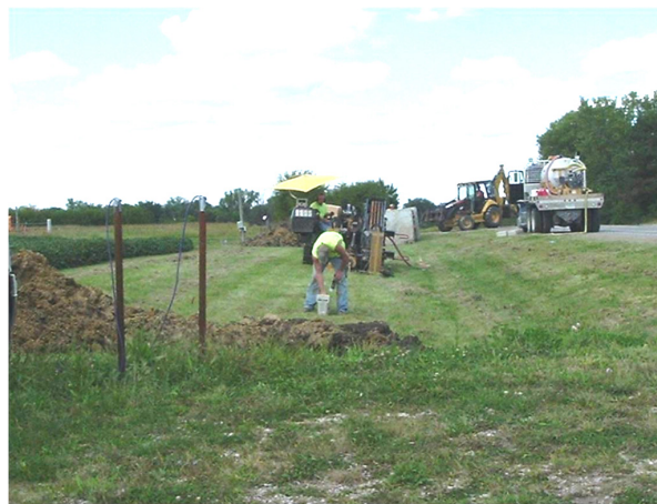
Figure 4.128. Bore approaching two pressure cells
