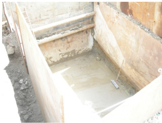
Figure 4.13. Trench box before installation began
