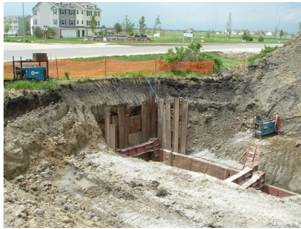
Figure 4.28. Launching pit with Delaware Avenue in background
