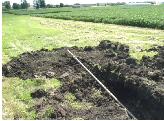
Figure 4.122. Pilot bore emerging from exit pit at point D
