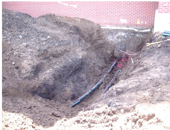
Figure D.33. The 4 inch diameter HDPE pipes connected to the building near point B
