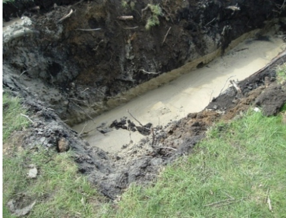
Figure D.44. Drilling fluid at the bottom of the exit pit at B
