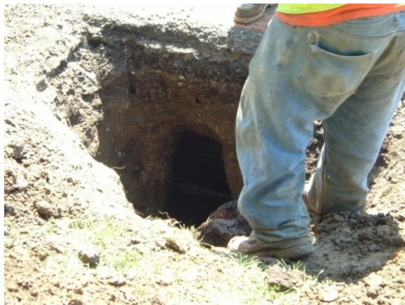
Figure D.2. Potholing by edge of pavement
