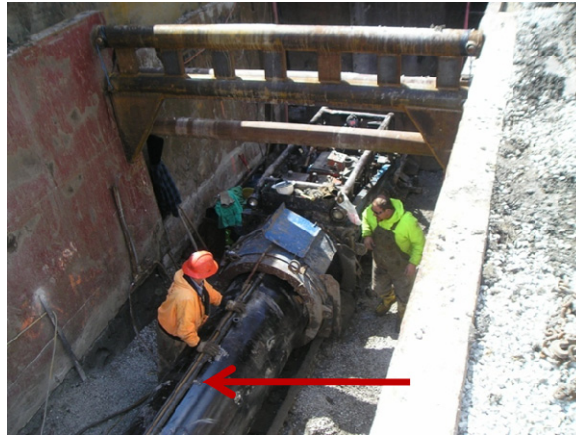
Figure 4.5. Pipe and auger boring machine operation, with fluid supply line, water line, and steering rod running along top of pipe
