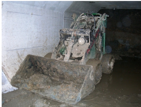
Figure 4.17. Skid loader used to move spoil from pipe to trench box to be removed by backhoe
