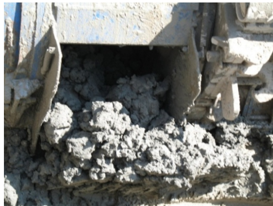
Figure 4.8. Weathered shale deposited out of auger boring machine
