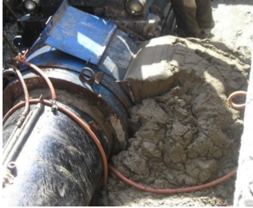
Figure 4.6. Sandy soil deposited out of auger boring machine
