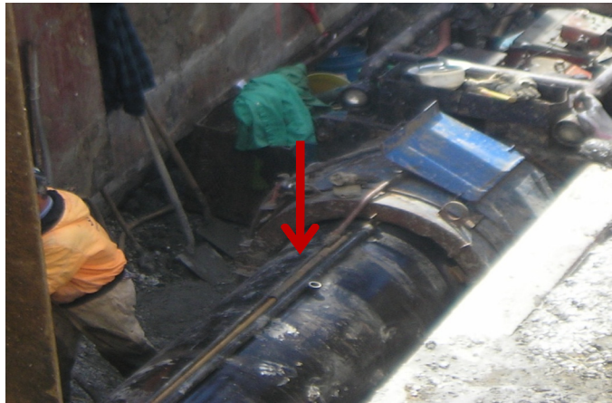
Figure 2.4. Waterline grade measurement pipe, steering rod, and fluid supply pipe attached to top of casing
