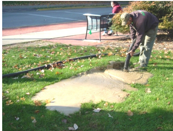
Figure 4.64. Drilling fluid at ground surface resulting from frac-out
