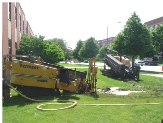
Figure 4.99. HDD rigs set up for 80-foot bore from points C to D (left machine) and 400-foot-bore from points C to A (right machine)
