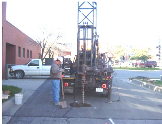
Figure 4.80. Drilling a borehole through asphalt
