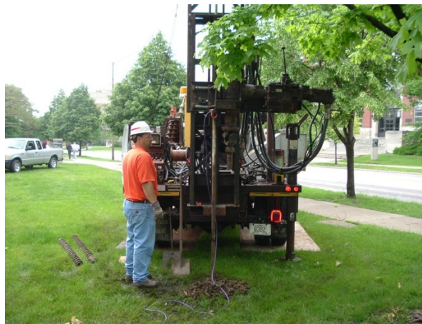
Figure 4.103. Installing push-in pressure cell
