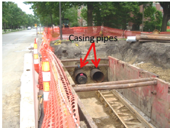
Figure D.17. Both casing pipes after boring are seen from the launching pit, and the carrier pipe can be seen in the casing pipe on the left
