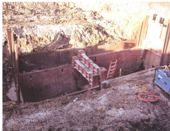
Figure 4.29. Launching pit with shoring and gravel base
