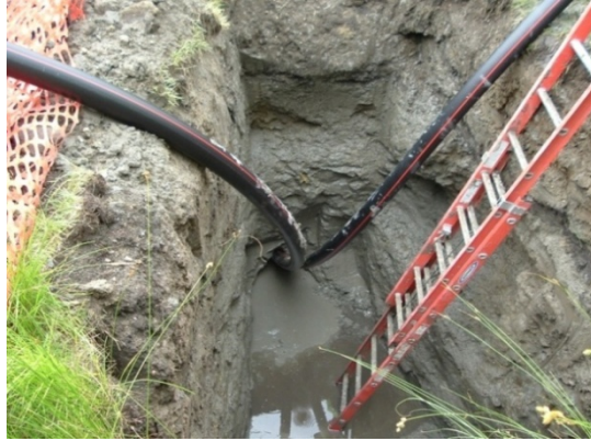
Figure 4.42. Installation of two conduits connected behind 18-inch reamer at point D
