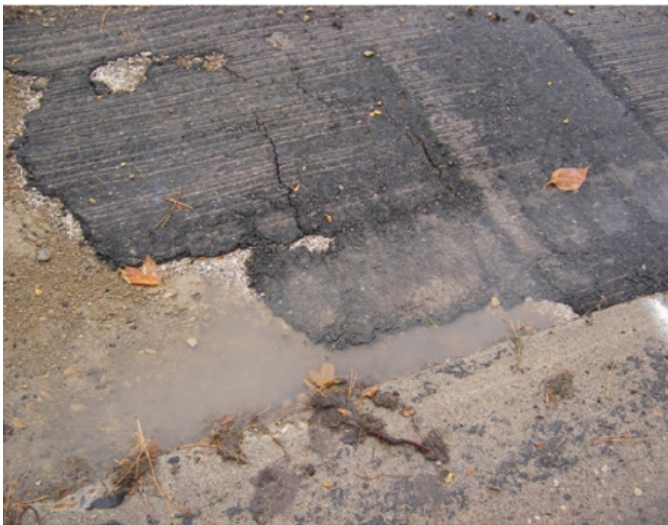
Cracks on temporary patch covering city practice trench indicating settlement (collapse) due to rain
