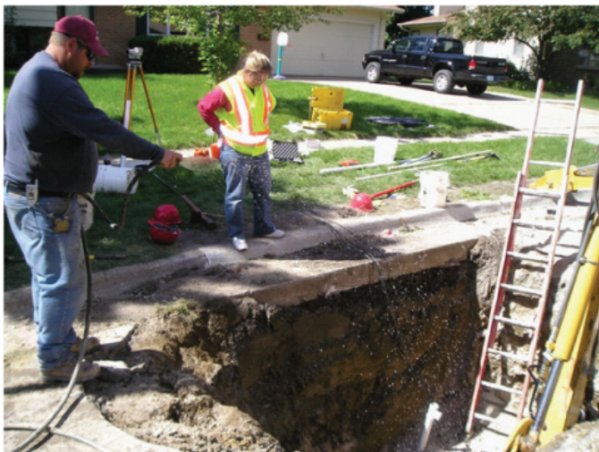
Watering backfill material to increase the moisture content beyond the bulking moisture content
