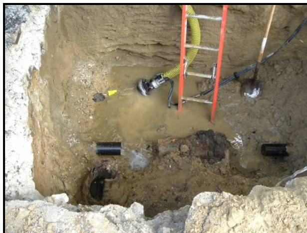
Figure 4.22. Water being pumped out of Trench F
