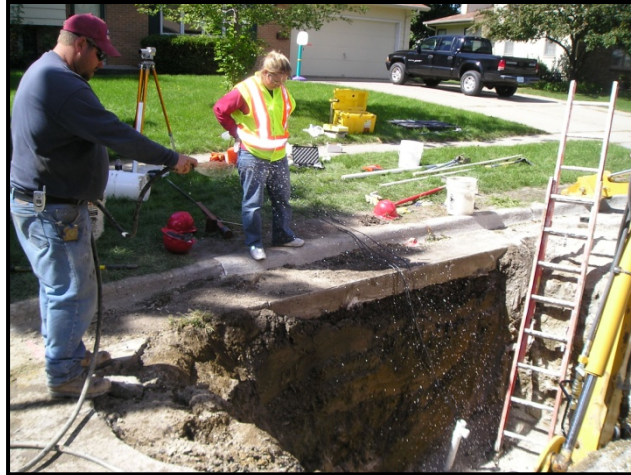
Figure 5.23. Adding water to the 3/8-inch minus backfill from above in Trench CI
