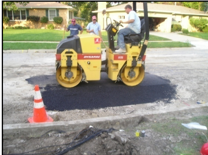
Figure 5.20. The placement of the temporary patch on Trench BI
