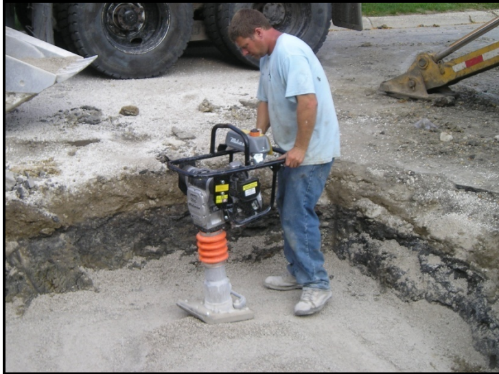
Figure 5.17. Impact rammer used to compact the backfill in Trench BI
