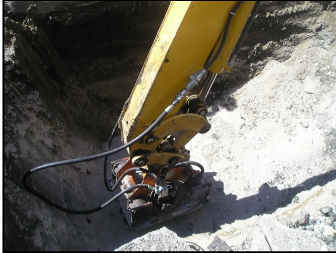
Figure 5.15. Vibratory plate compactor attached to the backhoe used to compact the backfill in Trench AI
