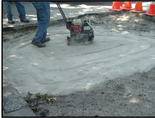
Figure 4.9. Small vibratory compactor used to compact the backfill in Trench B
