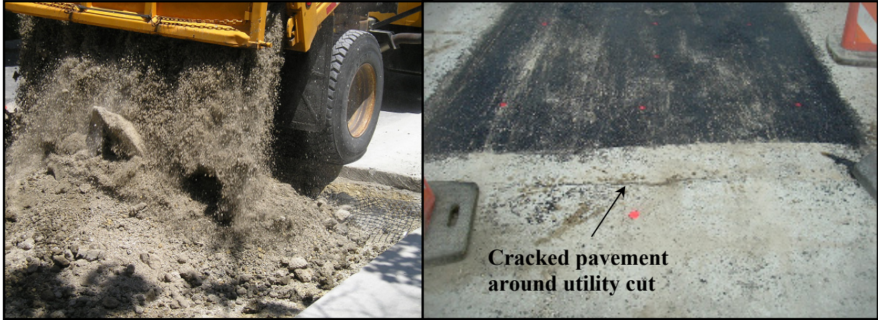
Figure 2.1. Cracking pavement surrounding the utility cut area because of construction equipment getting too close to the edge of open cut
