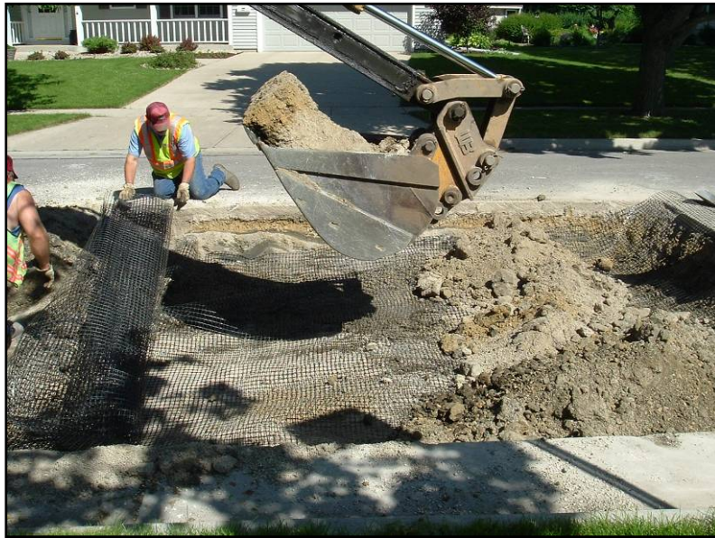
Figure 4.13. Geogrid being placed in Trench C
