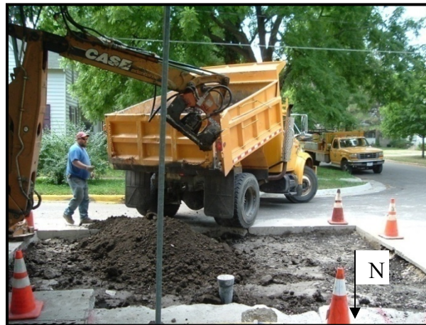
Figure 4.18. Soil previously removed being placed back in Trench E by a truck to the south, while a backhoe operates on the east edge of the pavement
