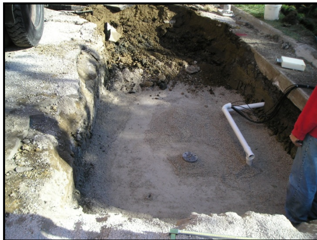
Figure 5.24. The excavation of the T-section being constructed for Trench CI
