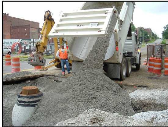
Figure 2.2. Large lift thickness used in utility cut trench backfilling
