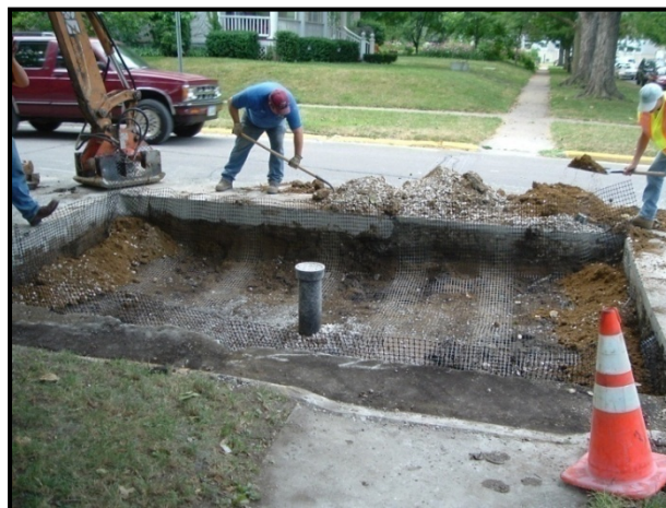
Figure 4.25. Geogrid being placed in Trench F after the fourth lift and T-section were excavated
