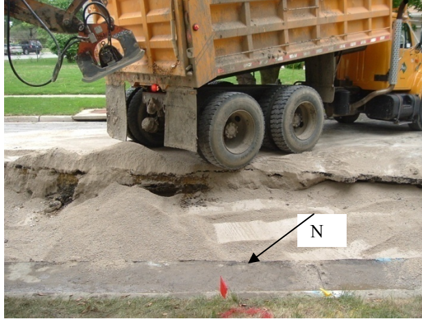
Figure 4.4. Truck backing into Trench A from the east while a backhoe with an attached vibratory plate compactor operates on the northwest side of the trench
