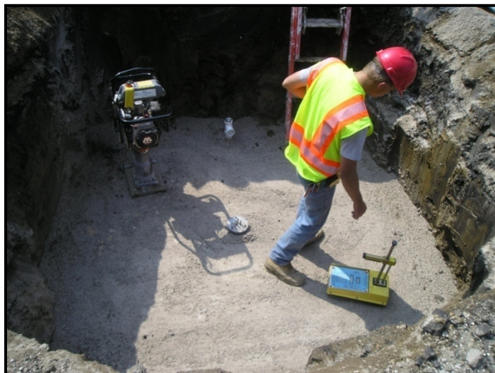
Figure 5.18. Nuclear density gauge used in Trench BI
