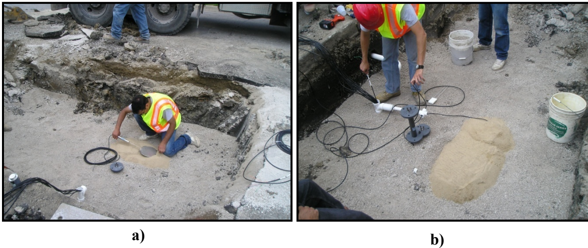
Figure 5.7. Pressure cell being placed within a lens of sand: (a) sand lens below the pressure cell, and (b) sand lens covering the pressure cells
