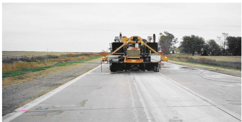
Surface grinder used in pavement rehabilitation
