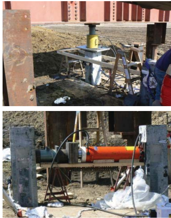
Figure 5. Vertical load test on UHPC pile P1 (top) and lateral load test on UHPC pile P2 (bottom).
