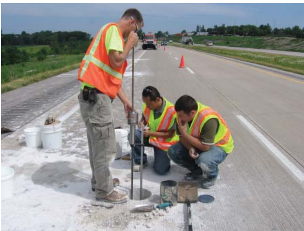
Dynamic cone penetrometer (DCP) test
