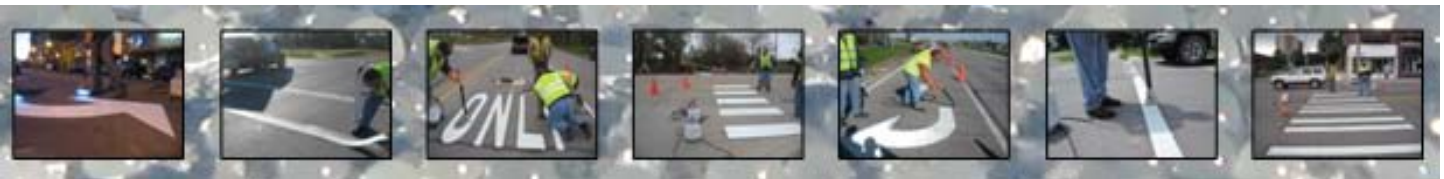
Transverse marking installation and performance demonstrations
