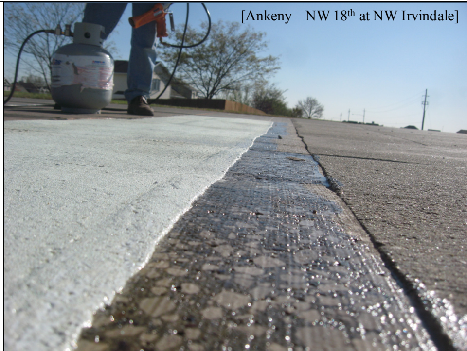
October 2008 – Urban Stop Bar Installation ( R_L=530 ), on concrete and within a groove of variable depth.
