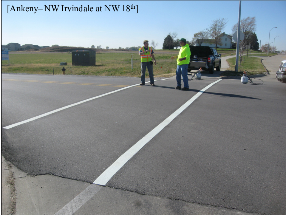
October 2008 – Urban 6" Crosswalk Installation ( R_L=487 ), on asphalt.
