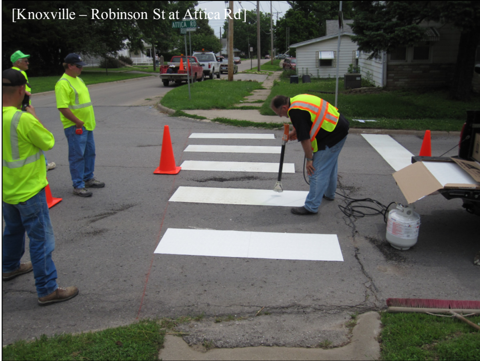
July 2009 – Urban 24" Stop Bar and Crosswalk on asphalt.
