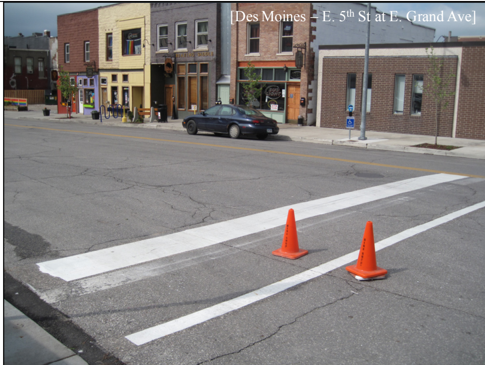
June 2009 – Epoxy Urban Stop Bar and Crosswalk on asphalt. Marking material is Poly Carb M-55.3
