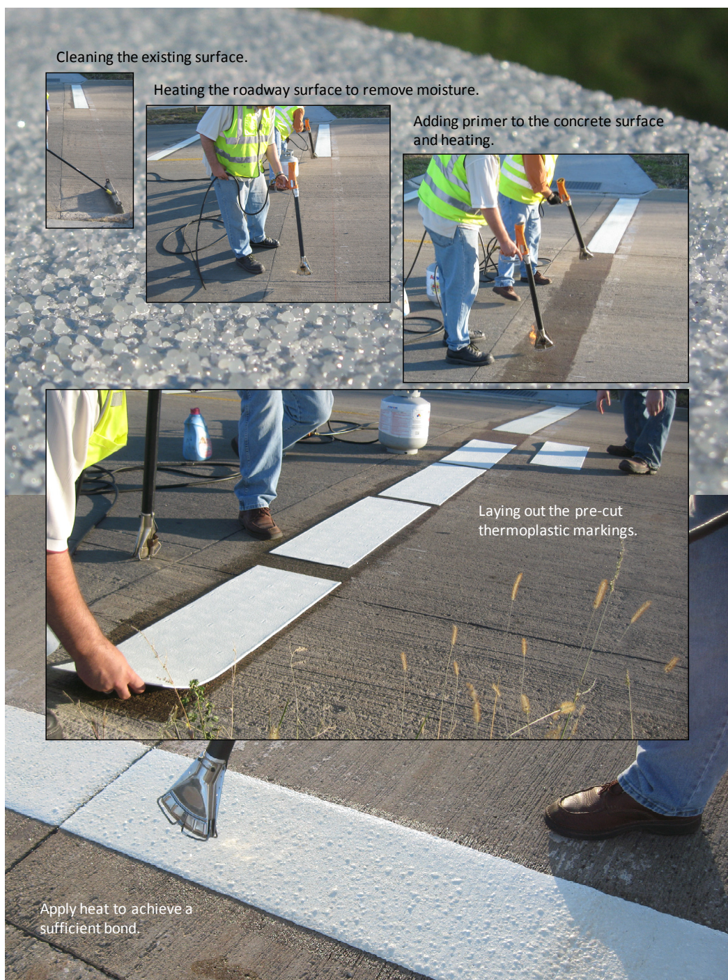
Figure 34. Installing preformed thermoplastic pavement markings
