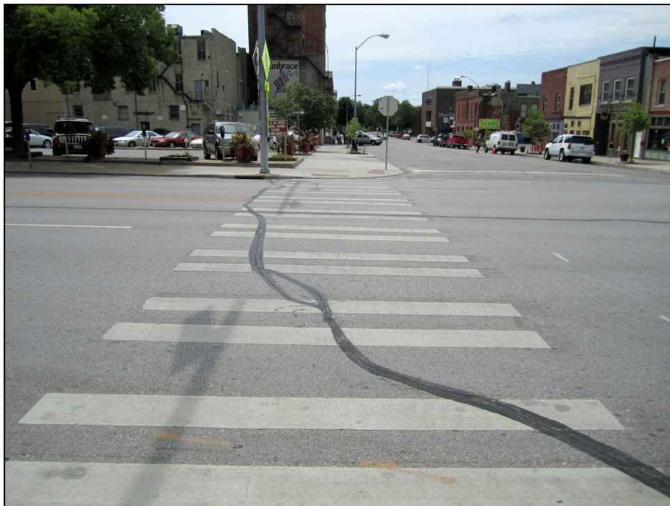
July 2010 – Same location as above, after 12 months. ( R_L=102 , Presence=Pass). The dark line is pavement joint sealant.
