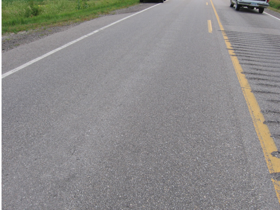
Figure C.7. Pavement Condition on A (Start) of V43 in Black Hawk County, IA (I.D. No. 13): Rubblization
