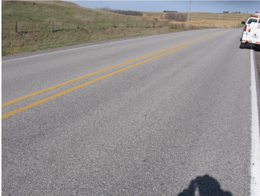
Figure C.25. Pavement Condition on C (End) of L55 in Mills County, IA (I.D. No. 32): Rubblization
