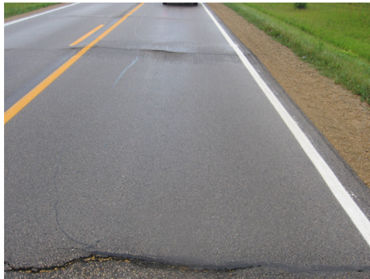
Figure 14. Picture of reflection cracking on HMA-overlaid PCC pavement (I.D. No. 47: IA139 in Winneshiek County)
