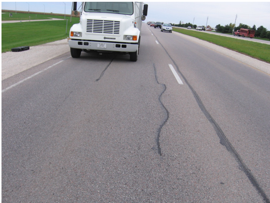
Figure C.32. Pavement Condition on A (Start) of IA141 in Polk County, IA (I.D. No. 33-2): Rubblelization
