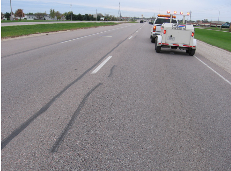
Figure C.28. Pavement Condition on A (Start) of IA141 in Polk County, IA (I.D. No. 33-1): Rubbblization
