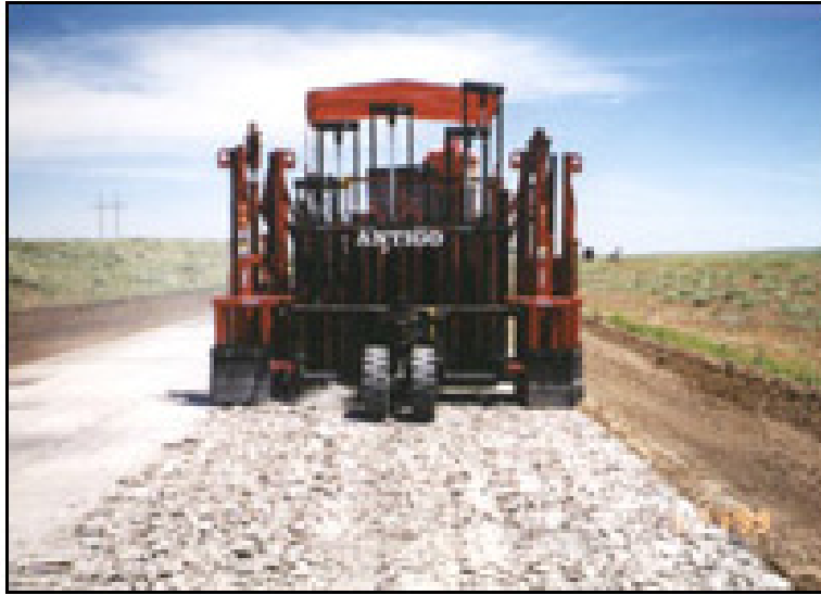
Figure 2. Multi-Head Breaker (Antigo Construction, Inc.)
