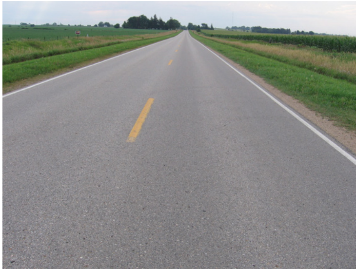
Figure 11. Picture of distress-free HMA surface on rubblized PCC (I.D. No. 12: C23 in Franklin County)
