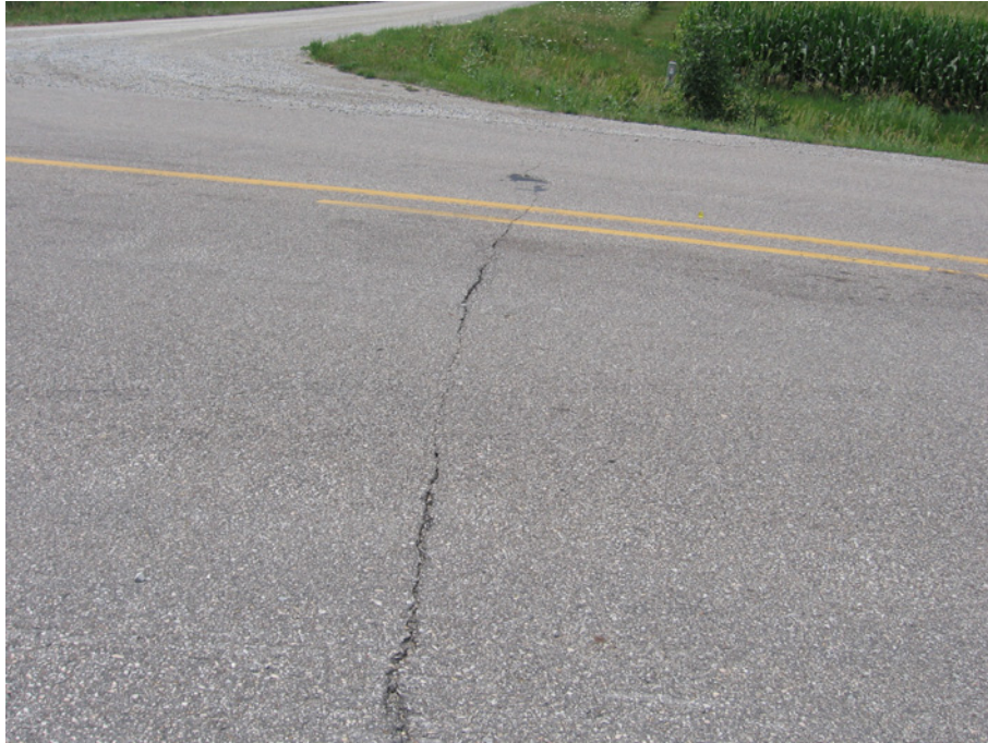
Figure C.11. Low Temperature Crack on V43 in Black Hawk County, IA (I.D. No. 13): Rubblelization
