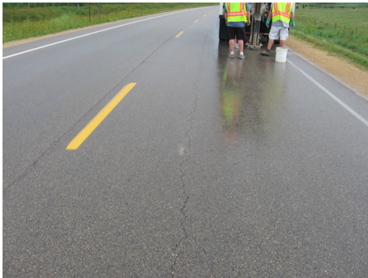
Figure 12. Picture of longitudinal cracking on HMA-overlaid rubblized PCC (I.D. No. 21: IA3 in Delaware County)
