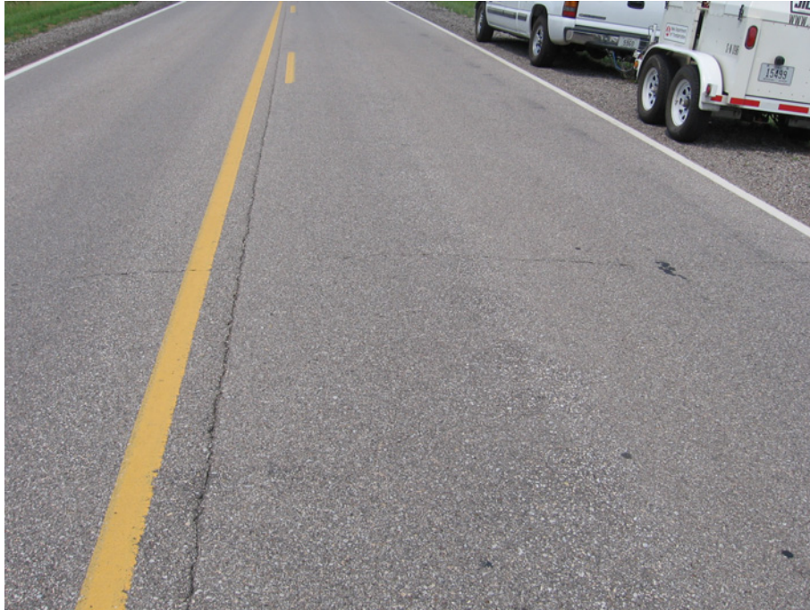
Figure C.9. Pavement Condition on C (End) of V43 in Black Hawk County, IA (I.D. No. 13): Rubblization
