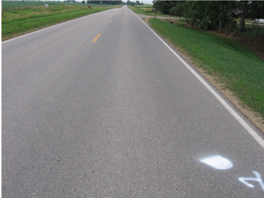
Figure C.19. Pavement Condition on A (Start) of C23 in Franklin County, IA (I.D. No. 26): Rubblization
