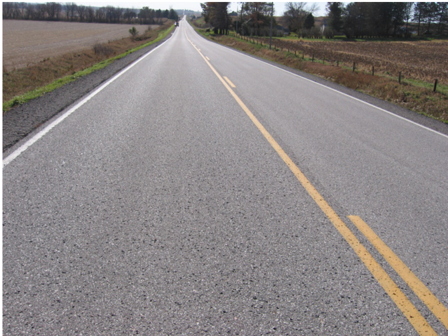
Figure C.22. Overall Pavement Condition on L55 in Mills County, IA (I.D. No. 32): Rubblelization
