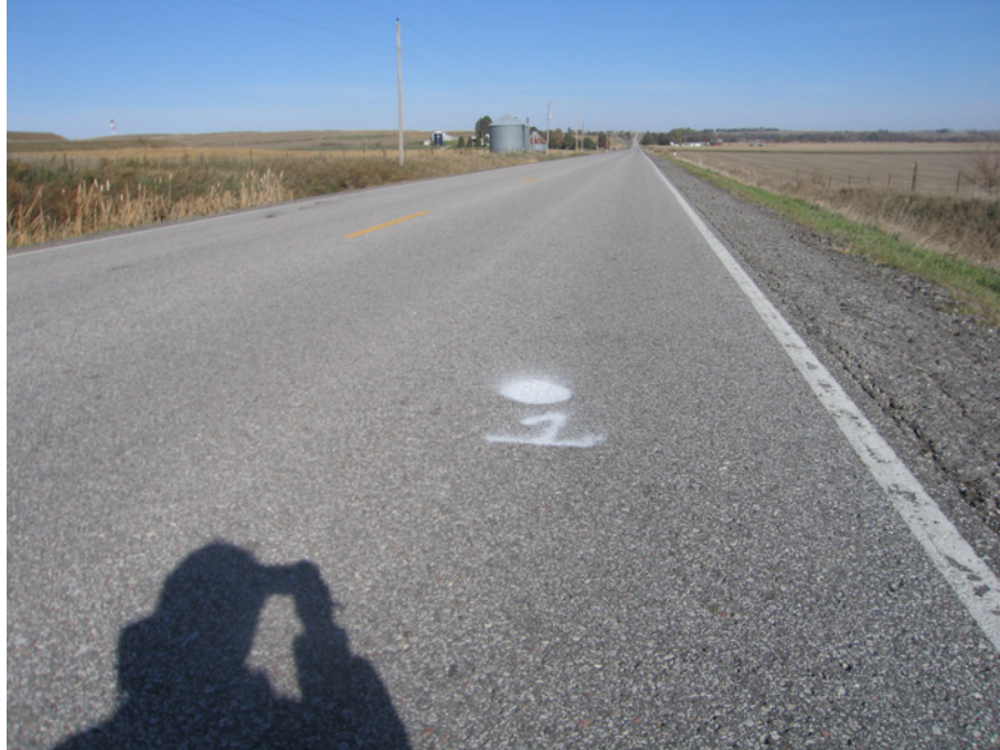
Figure C.23. Pavement Condition on A (Start) of L55 in Mills County, IA (I.D. No. 32): Rubblization
