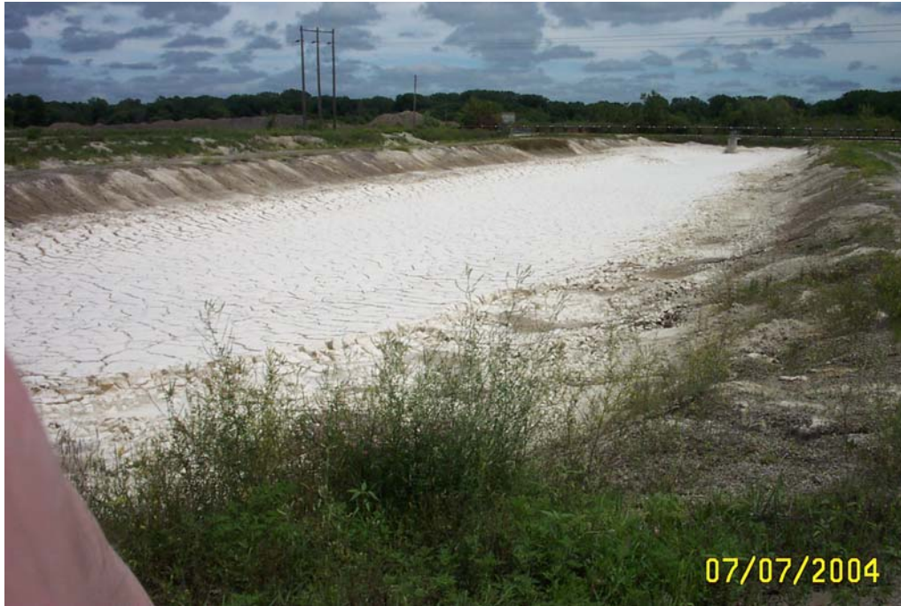
Figure 3: Dewatering Lagoon after 10 Months Settling
