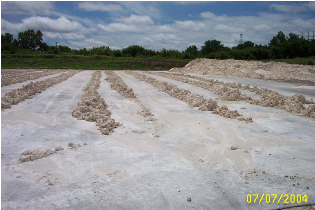
Figure 4: Solar Drying of Sludge in Windrows
