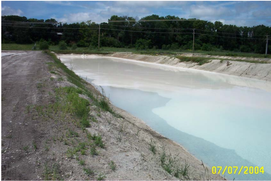
Figure 1: Dewatering Lagoon While Filling
