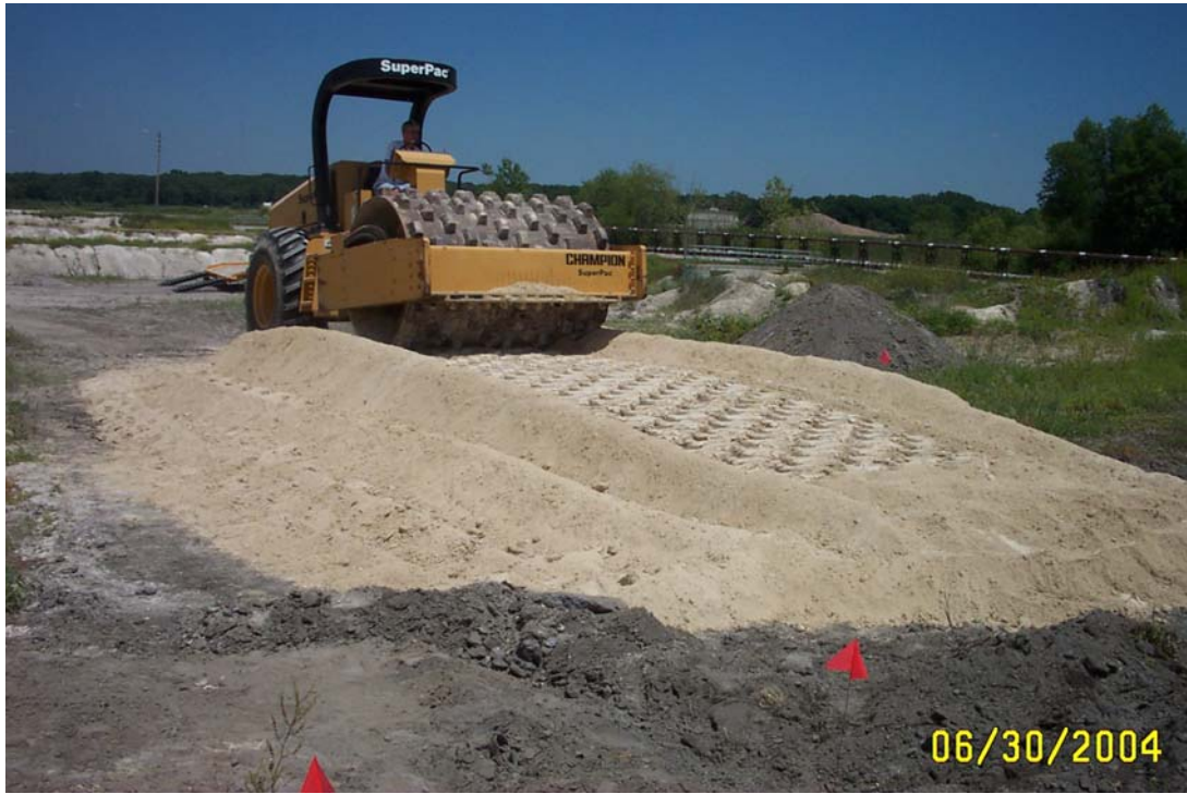
Figure 60: Compacting the test embankment
