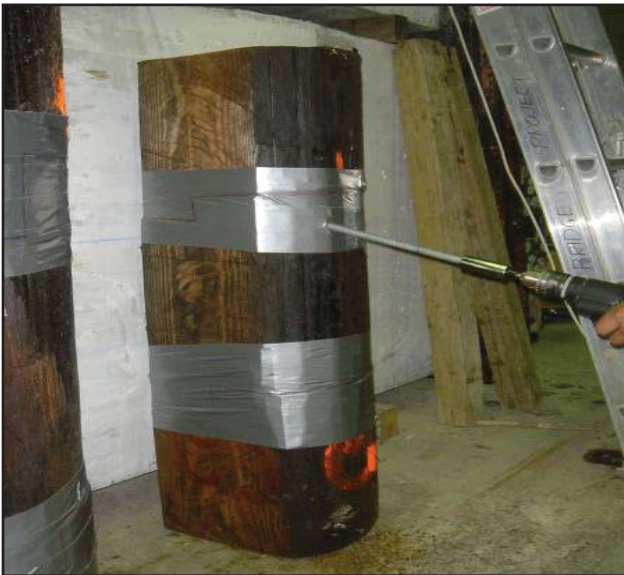
Timber pile repair using mechanical splicing
