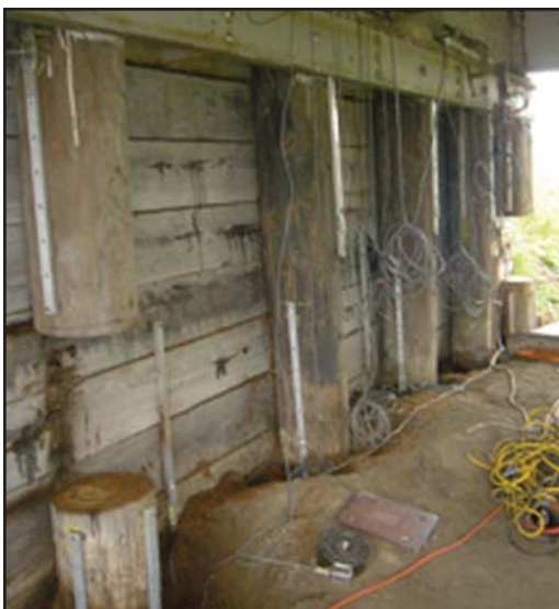
Humboldt County bridge with sections removed from three piles
