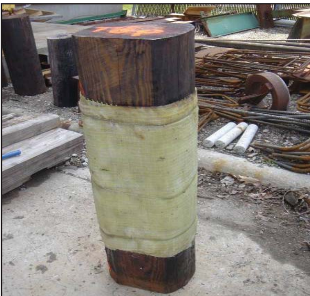
Timber pile repair using fiber reinforced polymer (FRP) wrap
