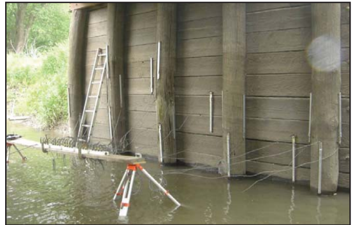
Bridge abutment instrumented with strain gauges
