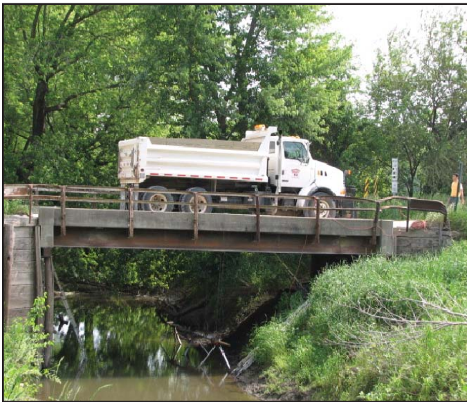
Testing of the Mahaska County bridge
