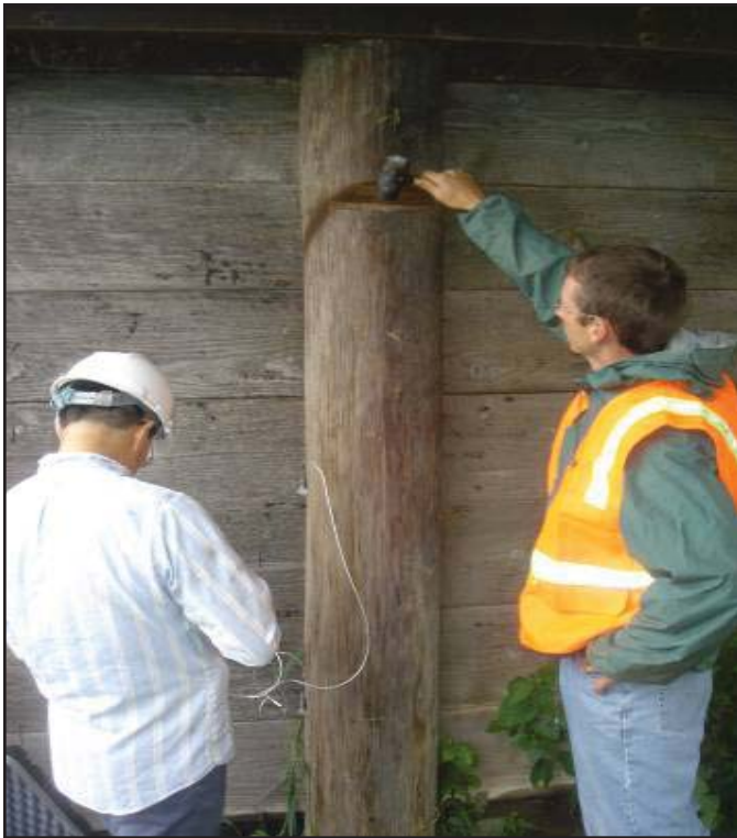
Pile integrity test: impacting the pile to generate a compression wave
