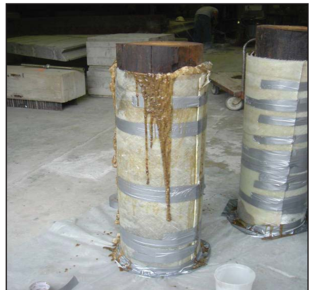
Timber pile repair using epoxy filler with FRP shell
