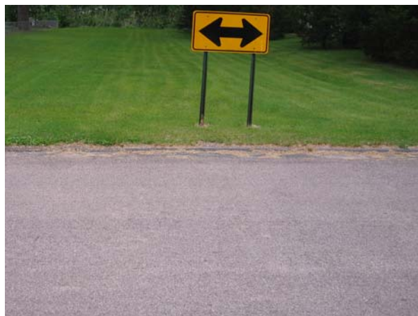
Figure 24. No reflected alligator cracking (chipmat)
