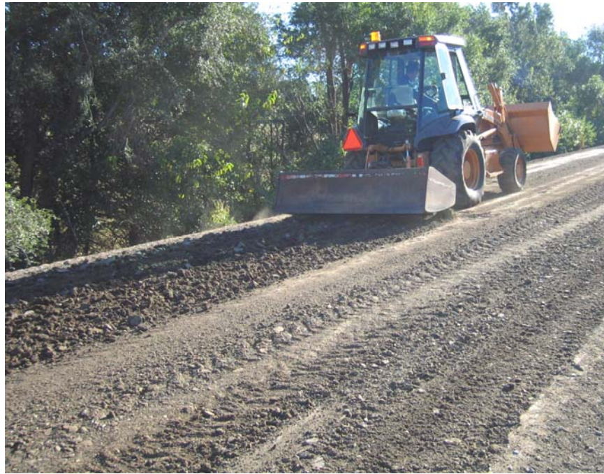
Figure 14. Stabilization of College Road
