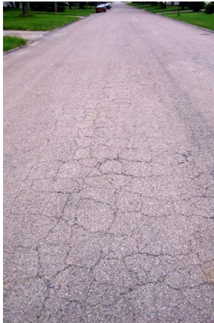
Figure 25. Reflected alligator cracking (no chipmat)
