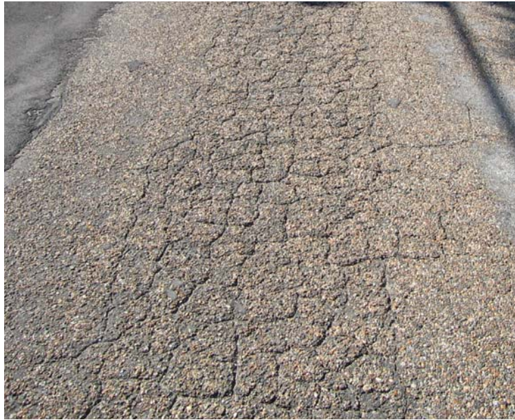
Figure 4. Alligator cracking on Vermont Avenue
