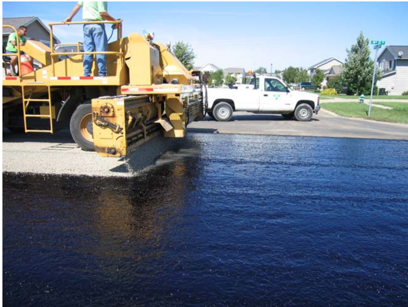
Figure 10. Seal coat construction on 74th Street
