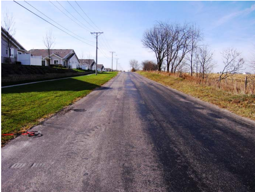
Figure F.5. Typical view of washed limestone on 74th Street (digitally enhanced photo)
