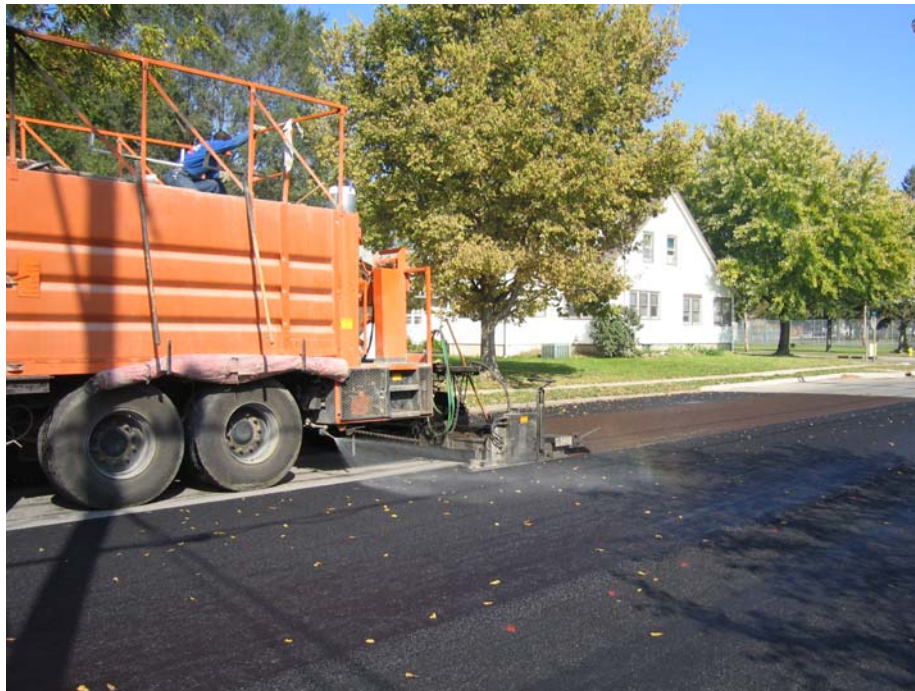
Figure 23. Micro-surfacing construction
