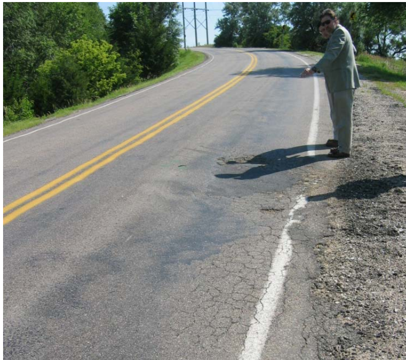
Figure 13. College Road alligator cracking, potholes, and bleeding
