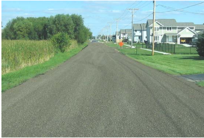
Figure 28. 74th Street pre-coated chips
