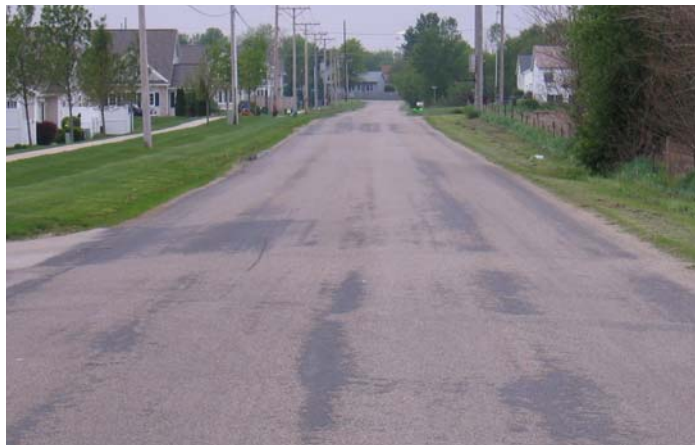
Figure 29. 74th Street washed limestone chip
