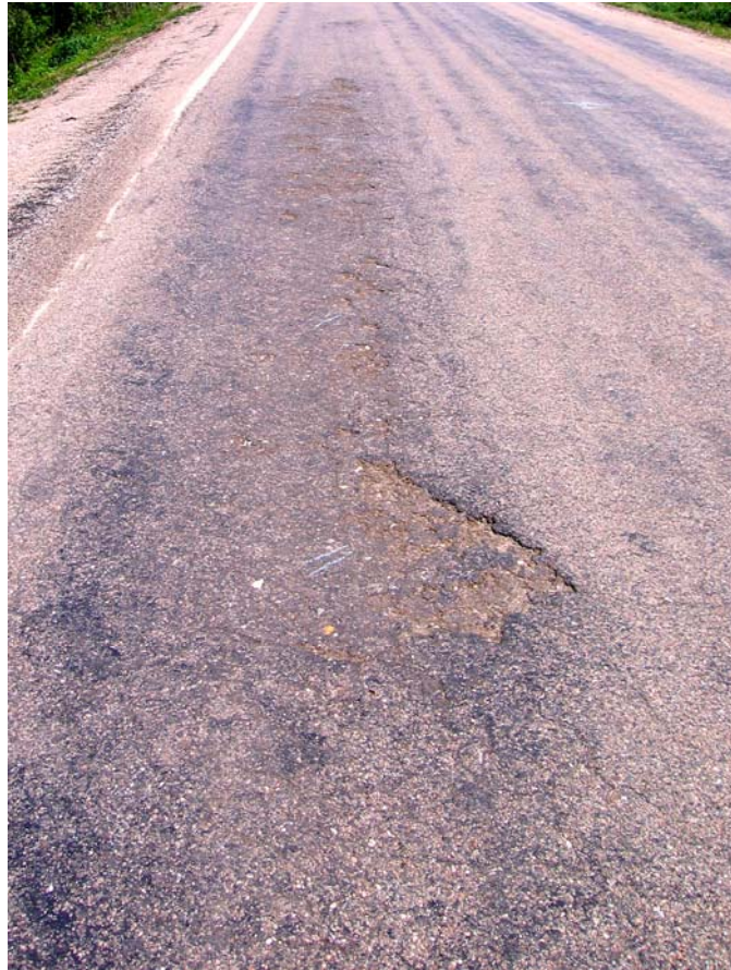
Figure 34. College Road alligator cracking
