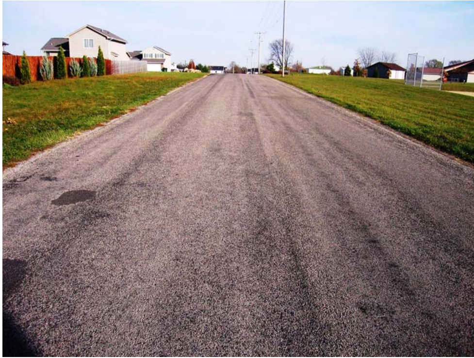
Figure F.7. Typical view of double seal coat on 74th Street (digitally enhanced photo)
