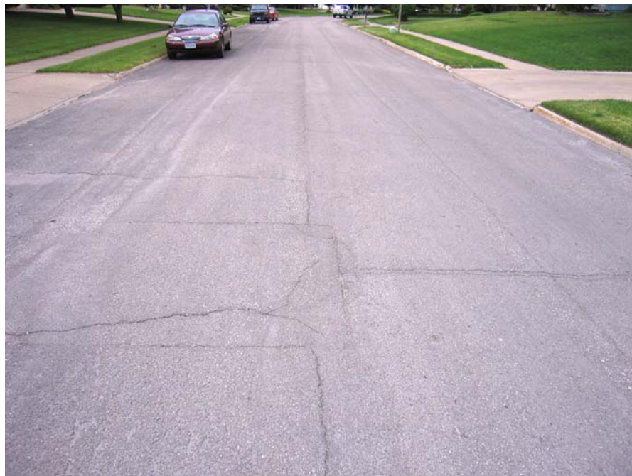
Figure 38. Reflective cracking on Aspen Drive
