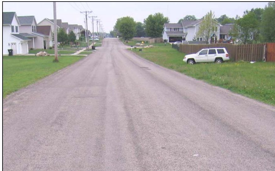
Figure 32. 74th Street double seal coat
