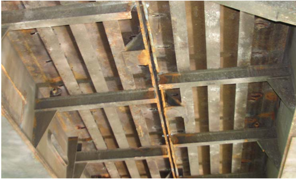
b. LFC gap between adjacent girder webs
