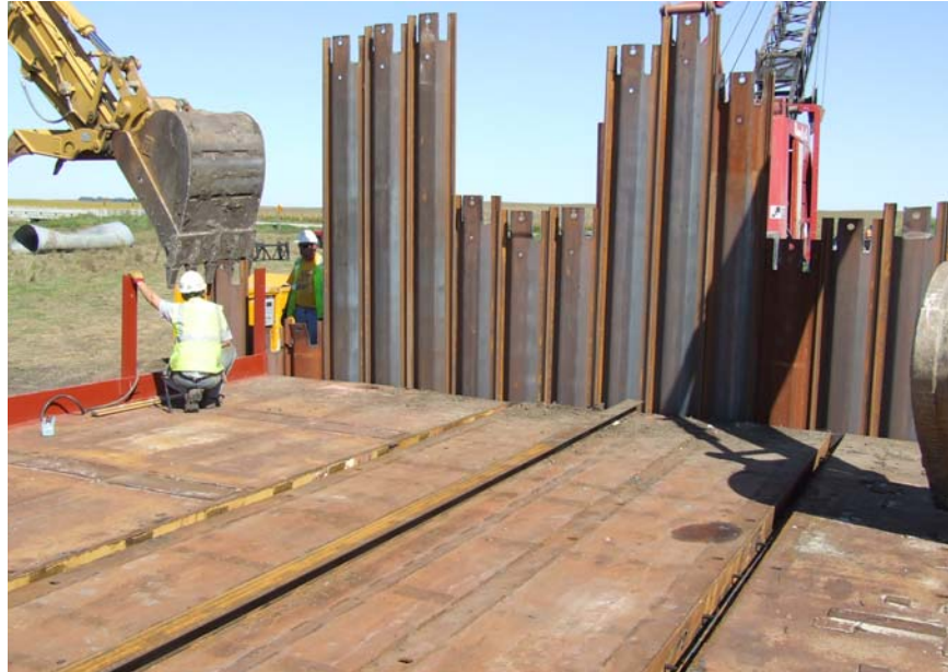
Figure B.6. East abutment after driving
