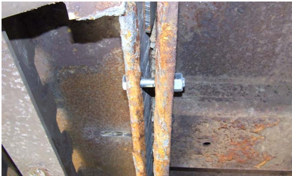
c. LFC bolted connection
