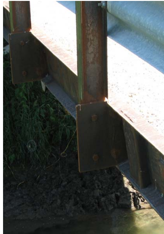
b. Guardrail connection to RRFC
