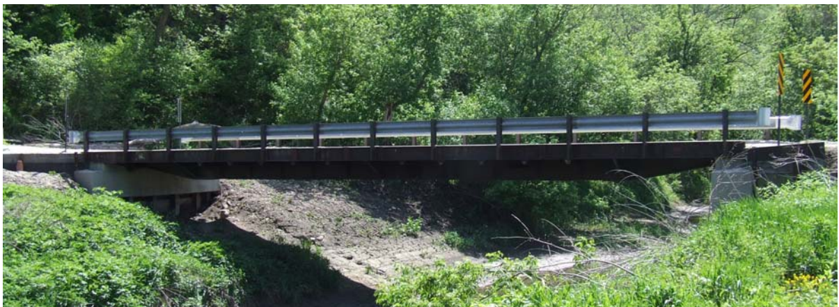
Figure D.5. Completed Winneshiek RRFC bridge
