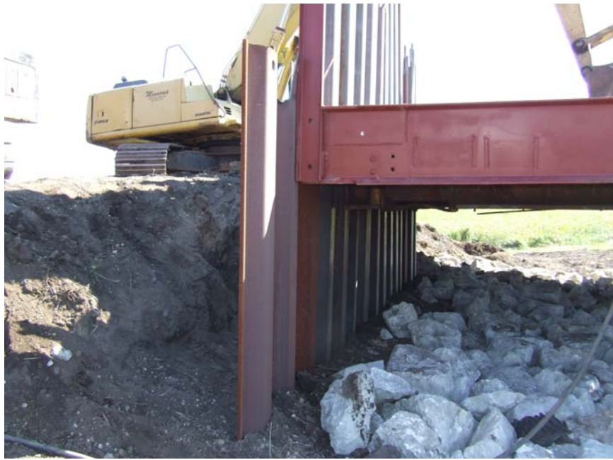
Figure B.4. Sheet pile abutment construction with no expansion joint provided
