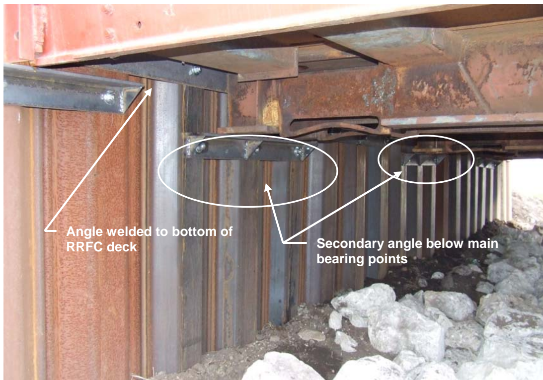
Figure B.8. Secondary angle attached below main bearing points
