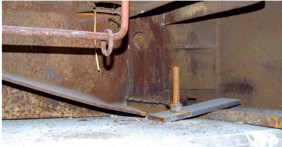
Figure 3.3. Clip angle to attach RRFC to abutment
