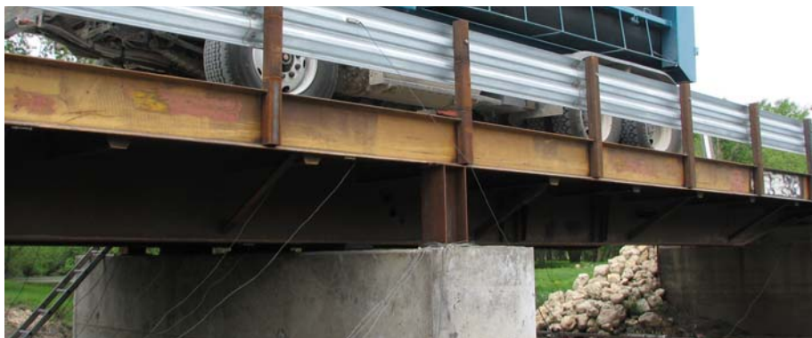
b. I-shaped Support at Exterior Girder
