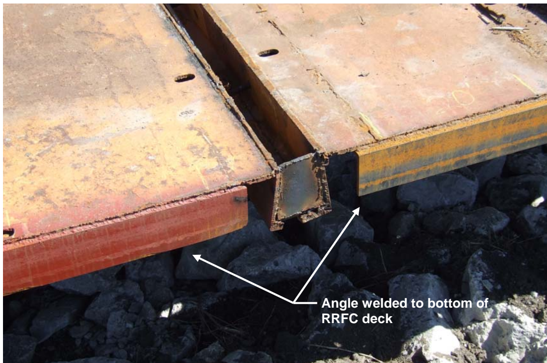
Figure B.7. Angle welded to bottom of RRFC deck
