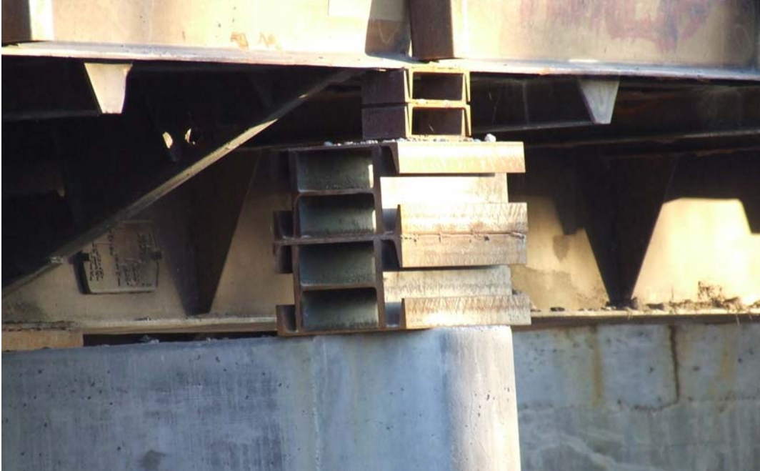
Figure 2.3. Miscellaneous I-shapes used as exterior girder support
