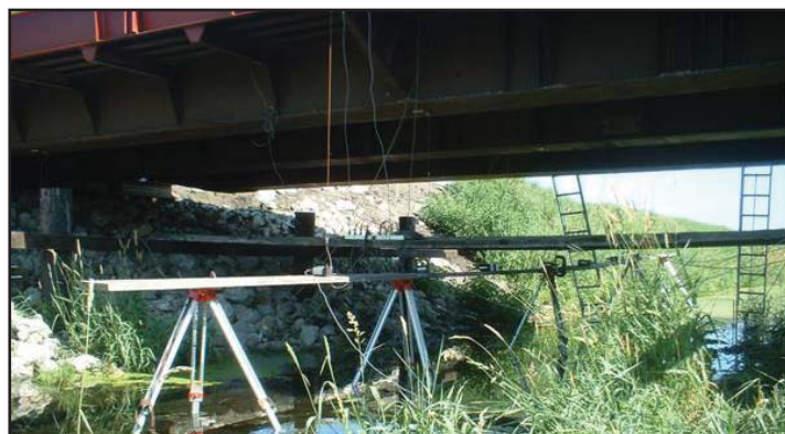
Deflection instrumentation installed below RRFC bridge
