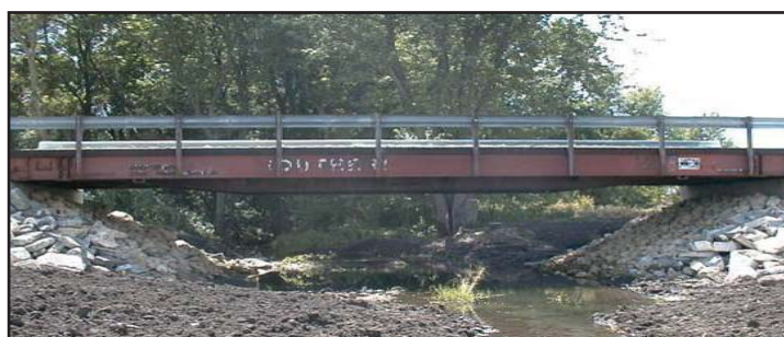
Single span RRFC bridge constructed using 56-foot railroad flatcars
