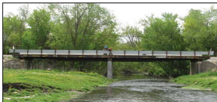
Multiple span RRFC bridge constructed using 89-foot railroad flatcars
