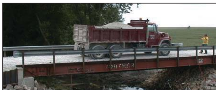
Test truck driving across single span RRFC bridge
