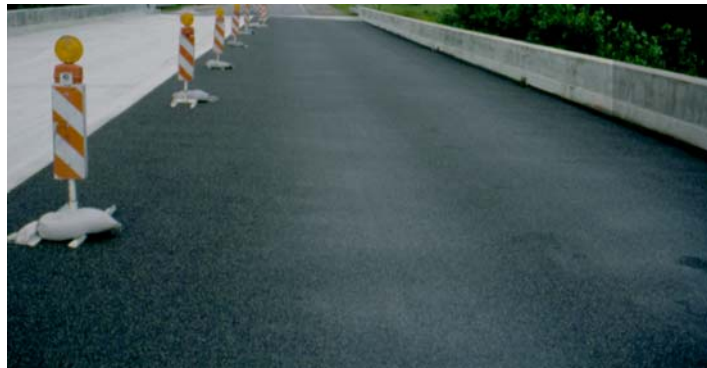
Photograph showing completed lane.
