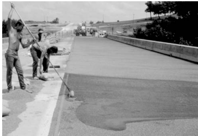
Photograph showing the spreading of Flexogrid.
