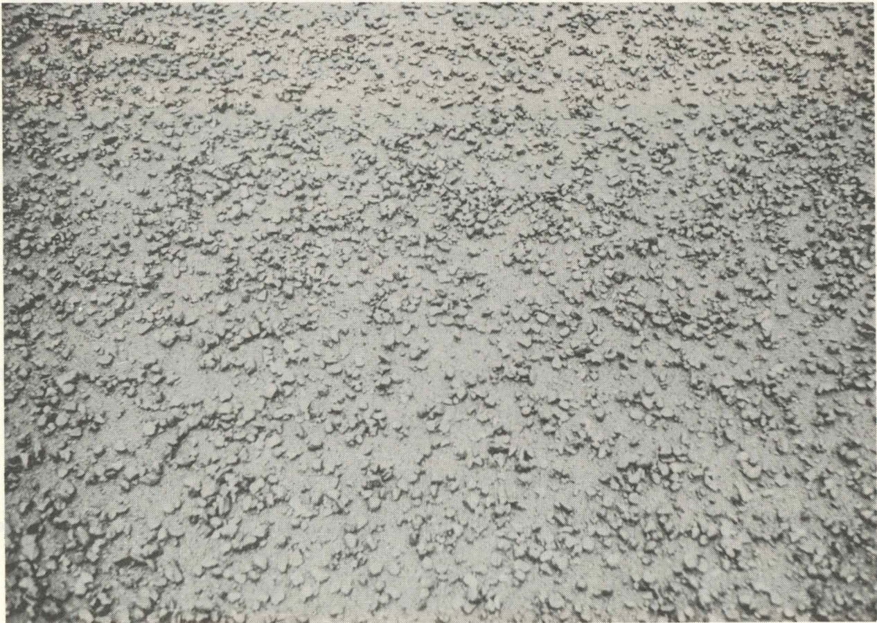
Figure 7: Sprinkled Aggregate Before Rolling
