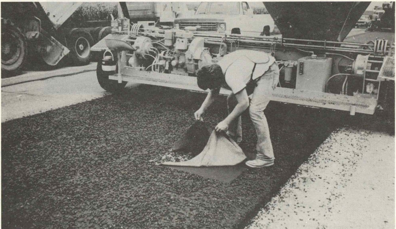
Figure 9: Collecting Sample for Application Rate Check
