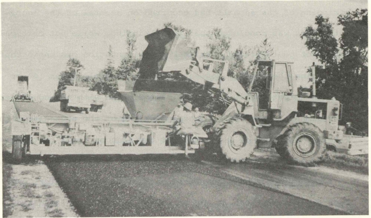
Figure 5: Charging the Bristowes Spreader
