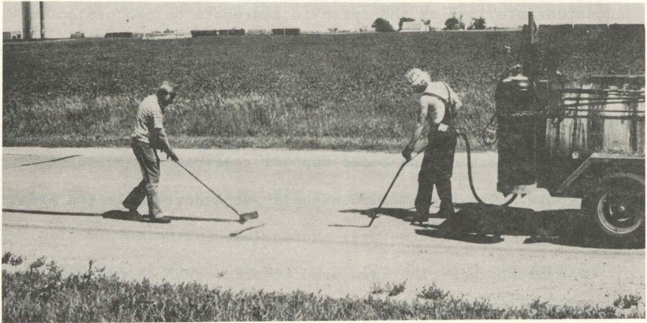
Figure 4: Filling Cracks with Overflex MS
