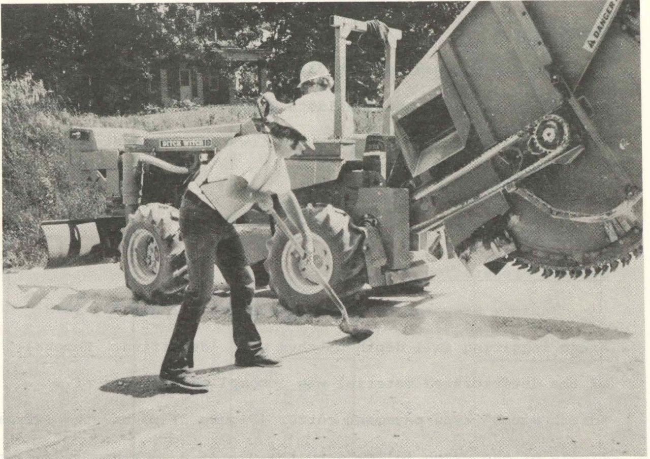
Figure 3: Preparing Patch Area
