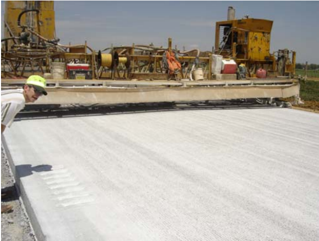
Figure 4. Application of Curing Compound
