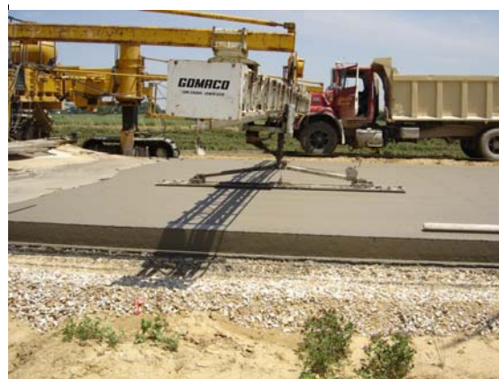
Figure 3. Slab behind paver
