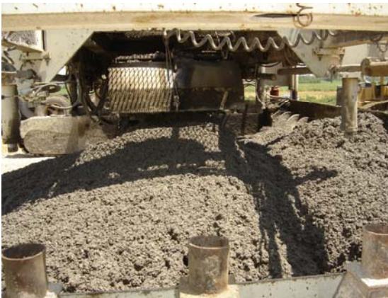
Figure 2. Mix at Belt Placer
