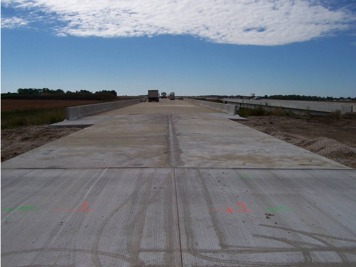
Figure 43. Finished north approach slab prior to opening to traffic.
