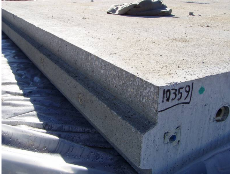
Figure 23. Keyway after completion of grinding.
