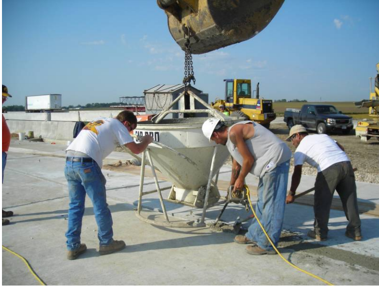
Figure 33. Filling of the longitudinal joint (photo by Iowa State University).
