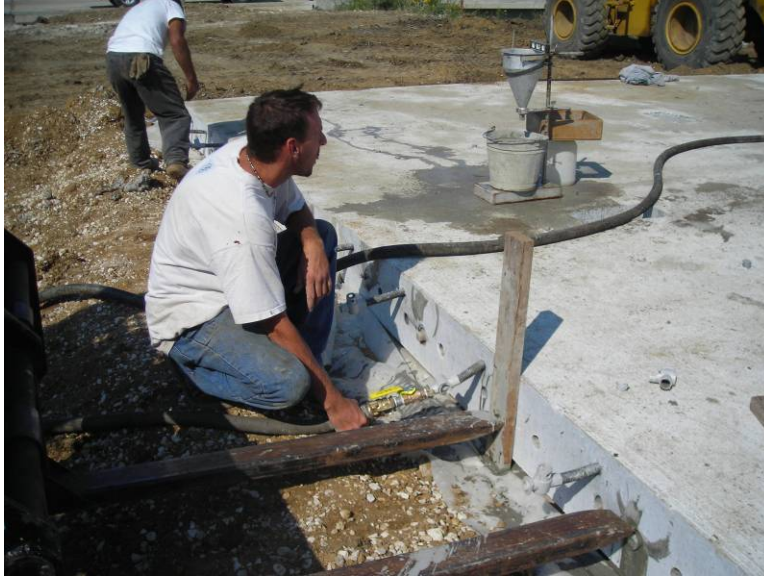
Figure 31. Grouting of the post-tensioning tendons (photo by Iowa State University).
