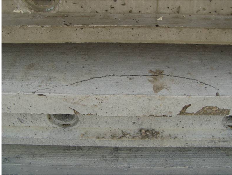
Figure 21. Damaged keyway after trial assembly.
