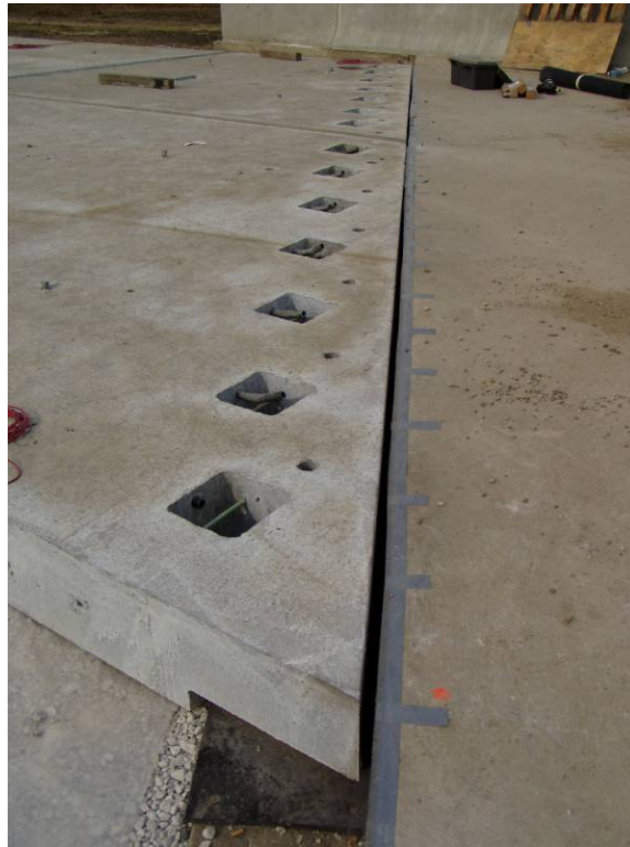
Figure 37. Joint between south approach slab and bridge abutment.
