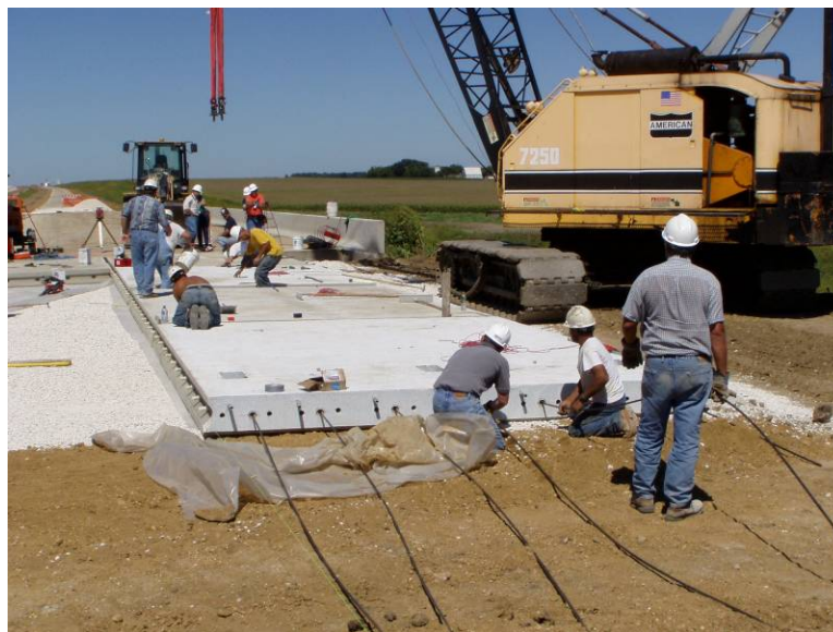
Figure 29. Inserting the longitudinal strands into the approach slab.
