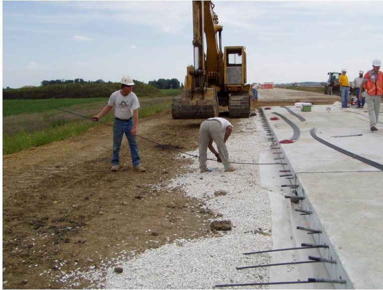
Figure 30. Inserting the transverse strands into the approach slab.
