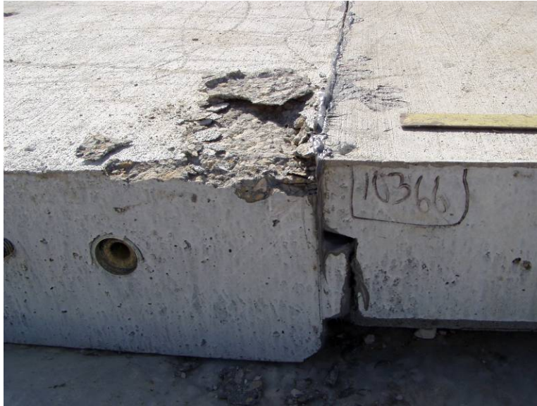
Figure 38. Minor joint spall which occurred during panel installation.
