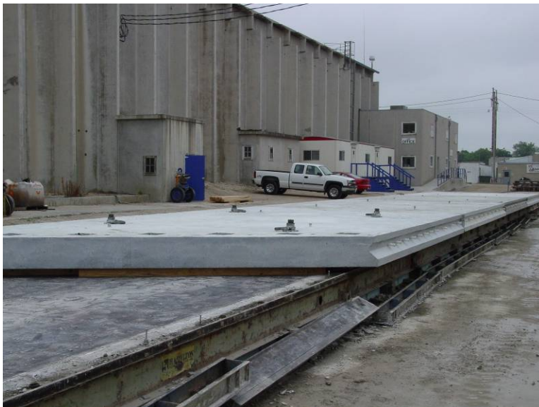
Figure 19. Trial assembly of precast panels at the fabrication plant (photo by Iowa DOT).
