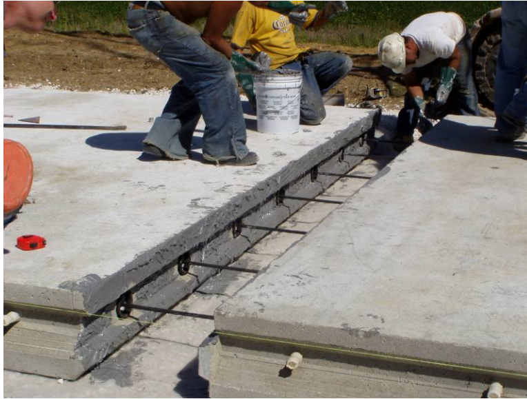
Figure 27. Application of joint epoxy during panel installation.
