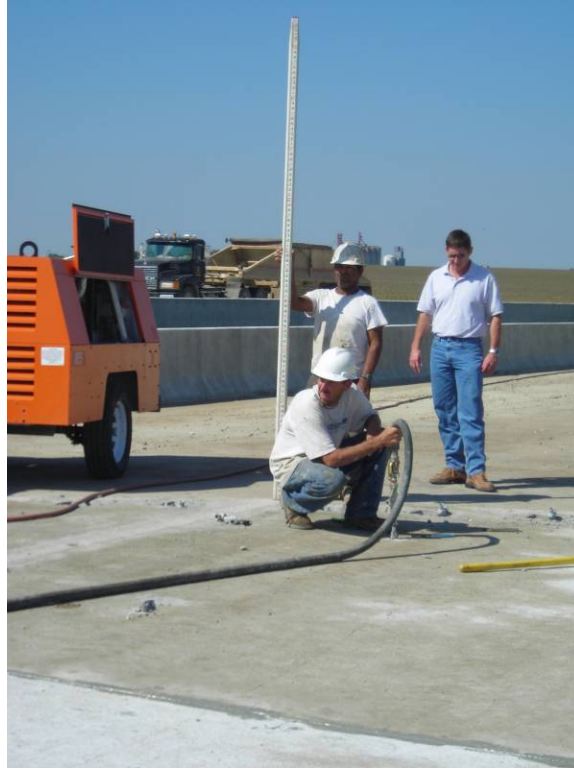
Figure 32. Rod and level were used to check for slab lifting during the underslab grouting operation. (photo by Iowa State University).
