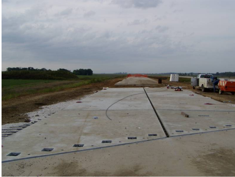
Figure 26. Finished approach slab prior to final post-tensioning.
