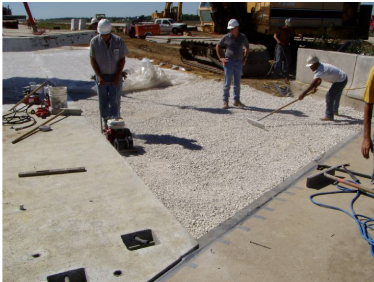
Figure 24. Grading and compaction of the aggregate base material.
