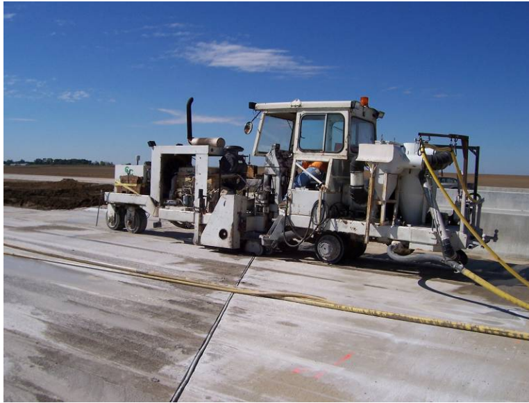
Figure 36. Diamond grinding the south approach slab.
