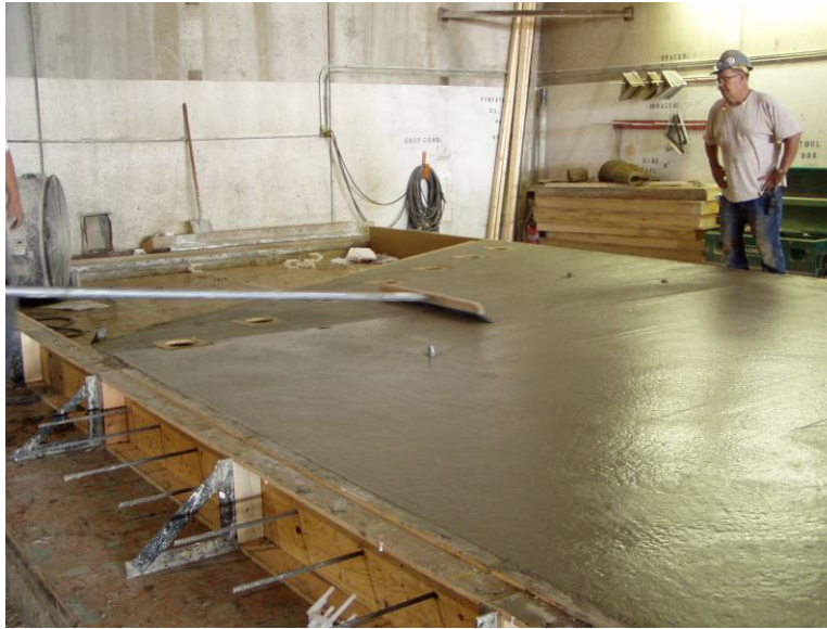
Figure 16. Application of the light broom texture to the panel surface.
