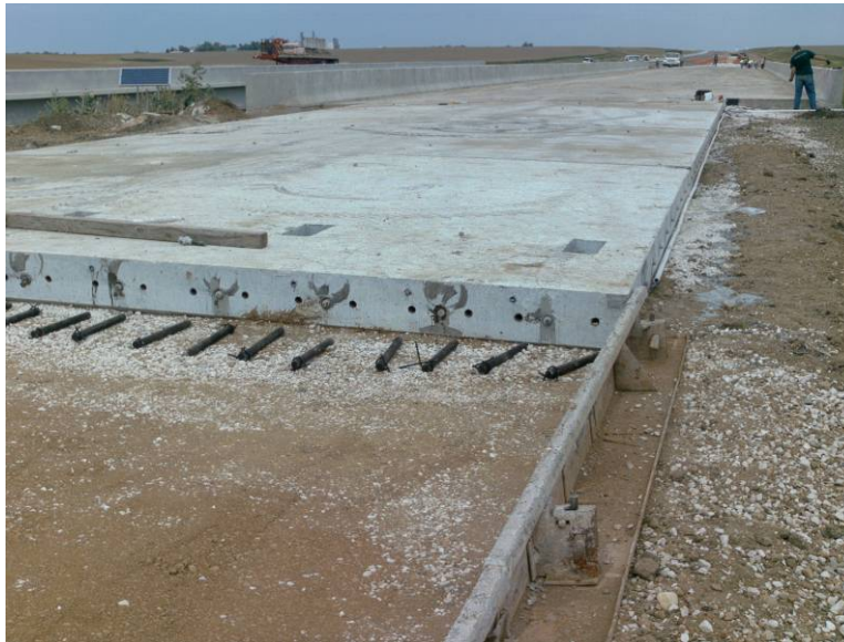
Figure 35. Dowels for the EF expansion joint prior to installing them in the precast panels (photo by Iowa State University).
