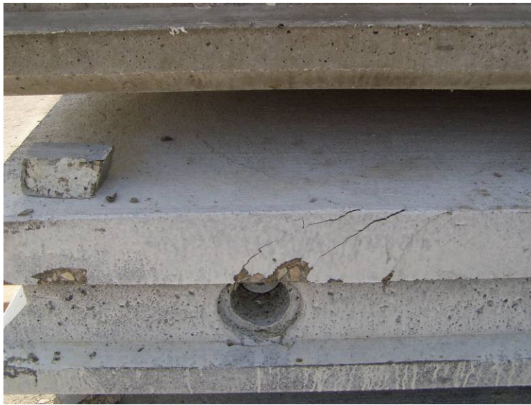
Figure 20. Damaged panel corner after trial assembly.
