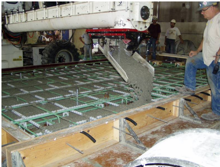
Figure 15. Placement of concrete for an abutment panel.
