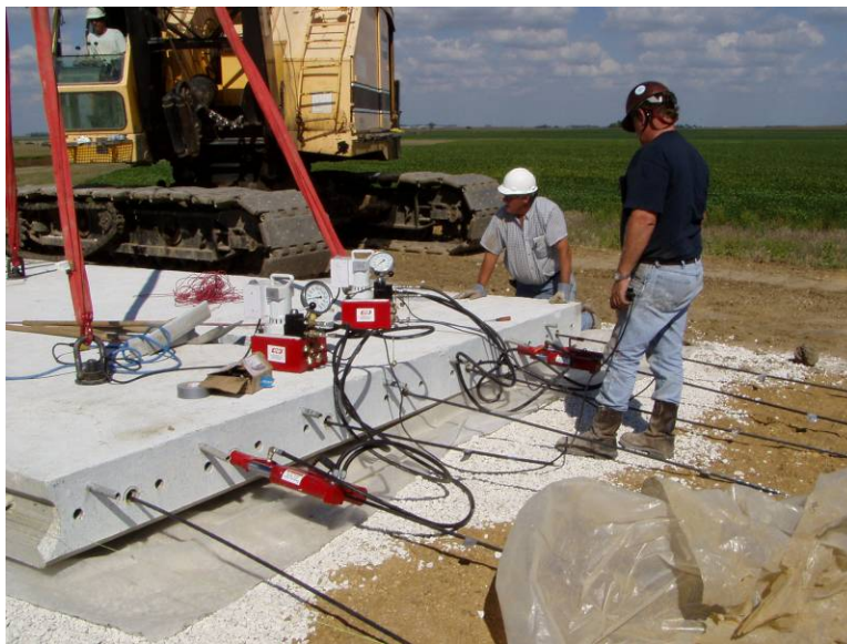
Figure 28. Temporary post-tensioning used to pull panels together.
