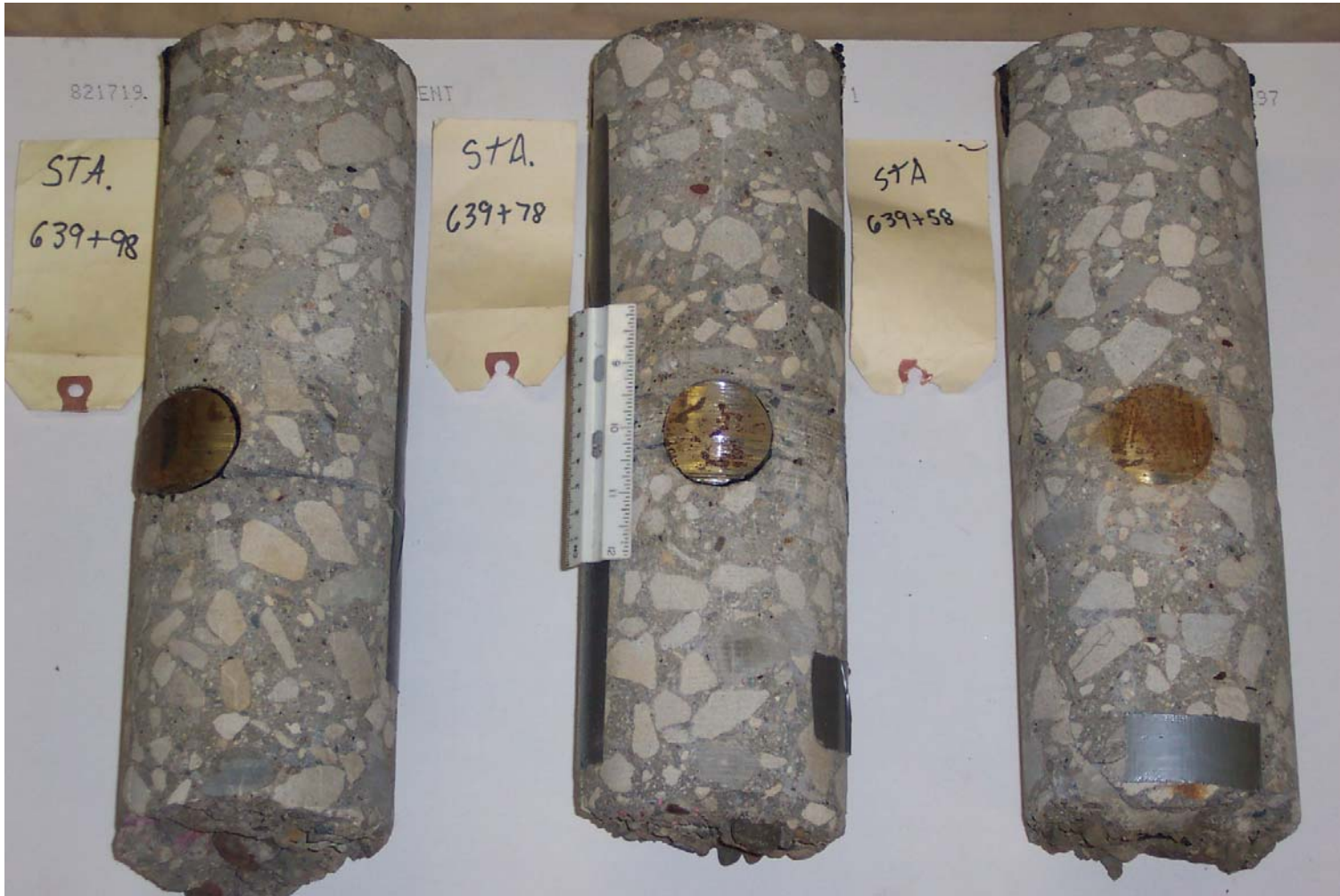
Figure D.3. Epoxy-Coated Steel Core Samples #s 1, 2, and 3 (left to right)
