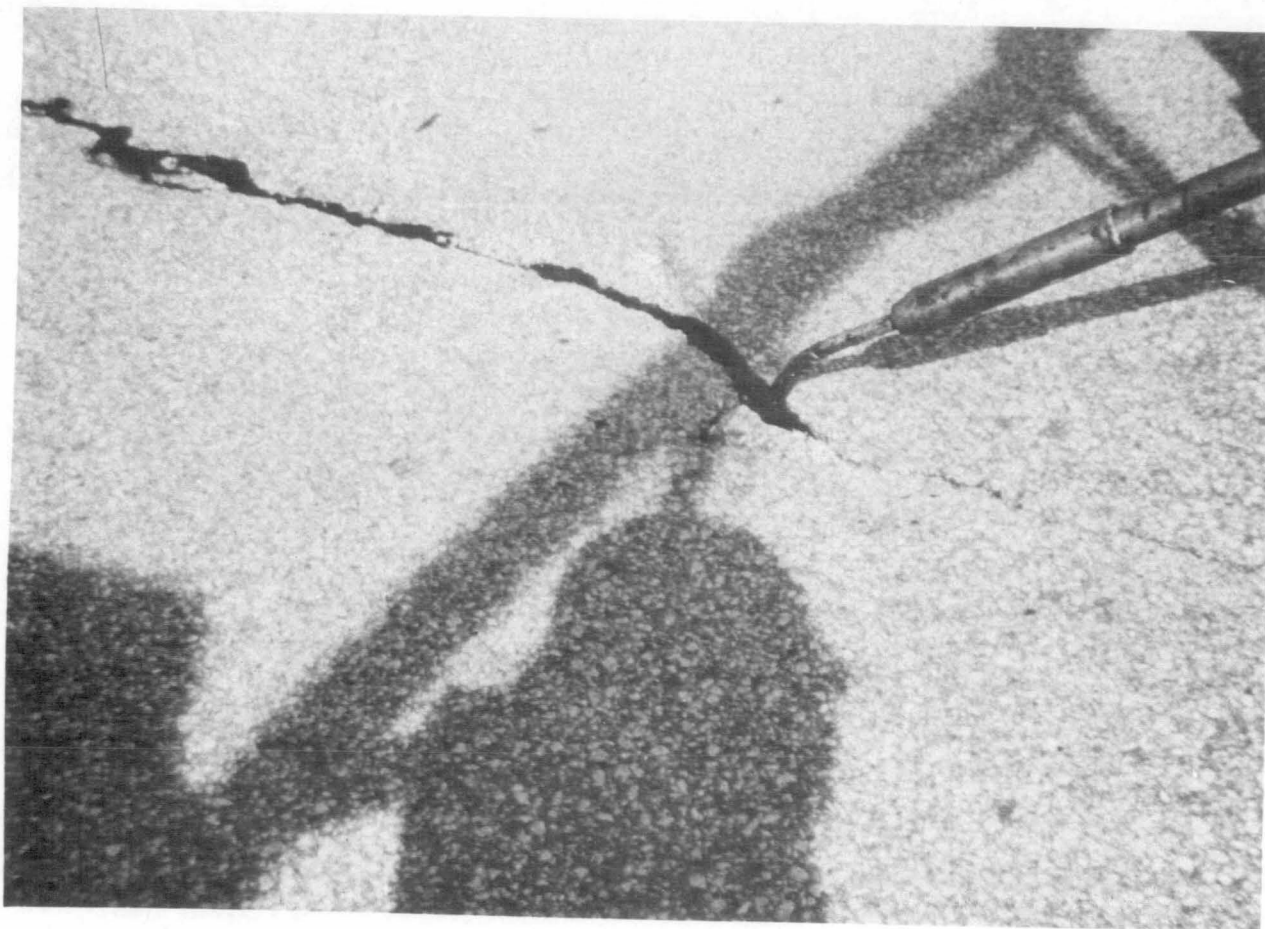
(Figure 3) Sealing of a crack.
