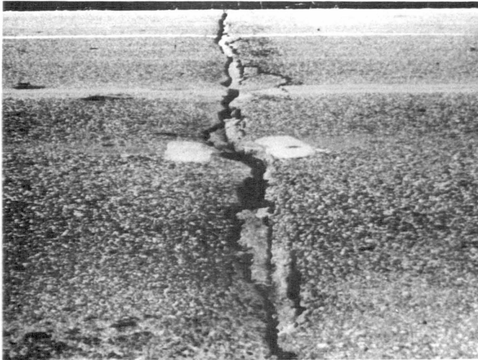
(Figure 1) Badly deteriorated transverse crack.
