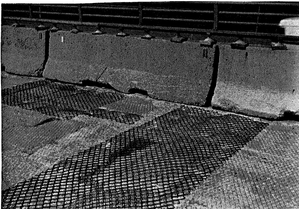
Figure 1 Anode Mat to Prevent Short Between Anode and Exposed Rebar
