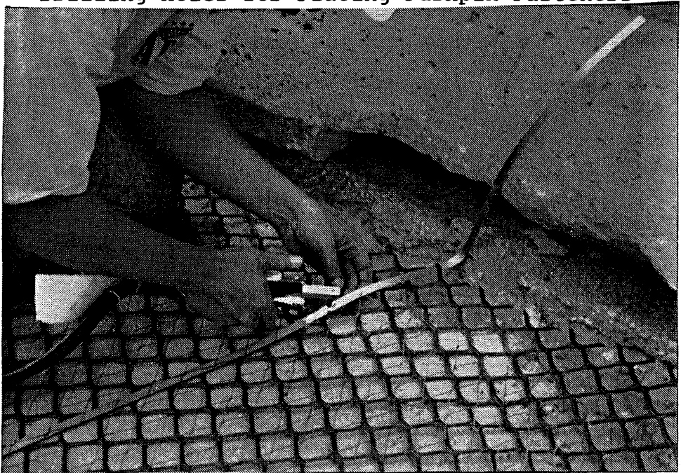
Figure 3 Welding Current Density Strip to Anode With Extra Length to Connect Both Sides of Zone
