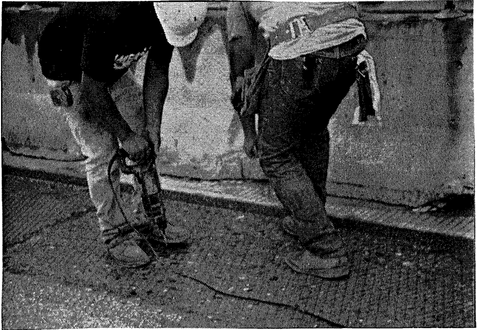
Figure 2 Drilling Holes for Placing Pushpin Fasteners
