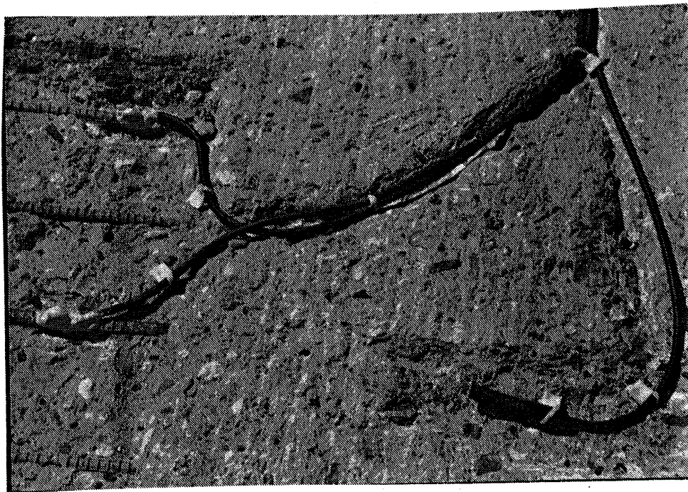
Figure 6 System Negatives and Graphite Reference Electrode
