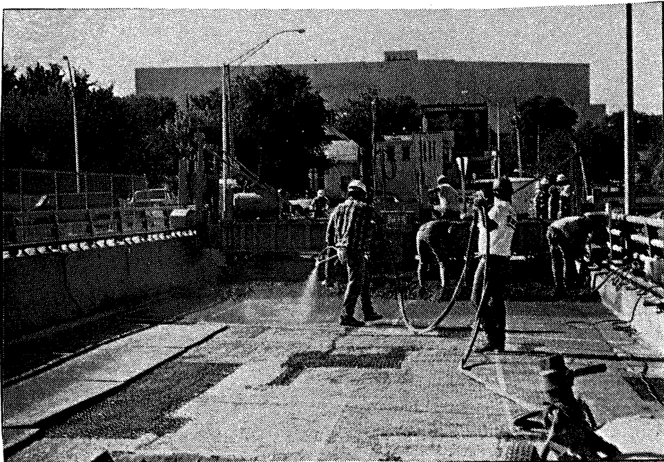
Figure 9 Placing Overlay, Spraying Grout, and Plywood Runway for Concrete Buggies
