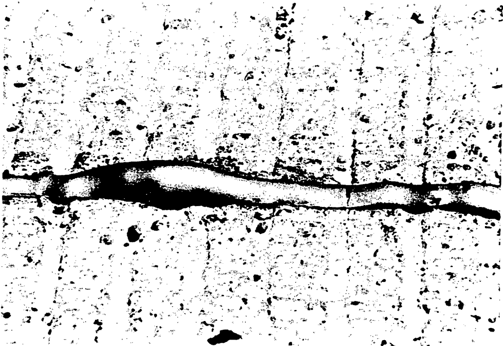
Figure 12 Nitrile Rubber Sealant "Bubbled" Out of the Joint
