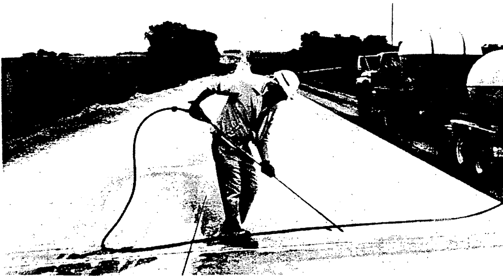
Figure 7 Special Joint Cleaning With High Pressure Water Blaster
