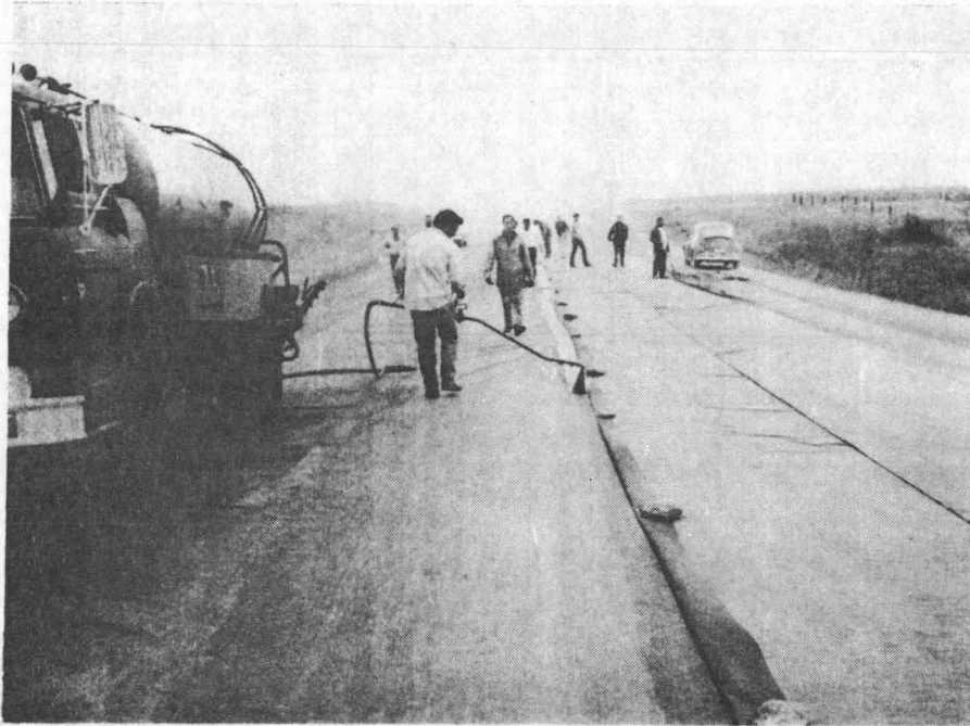
Figure 4: Sealing Lapped Fabric Joints
