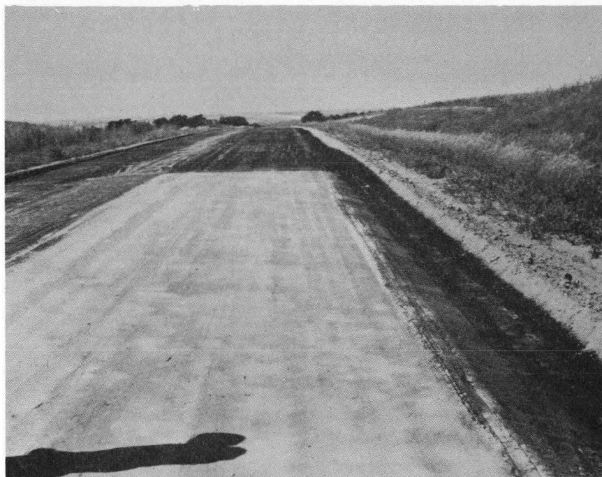
PHOTO 23: Completed base with RC-0 cure.
