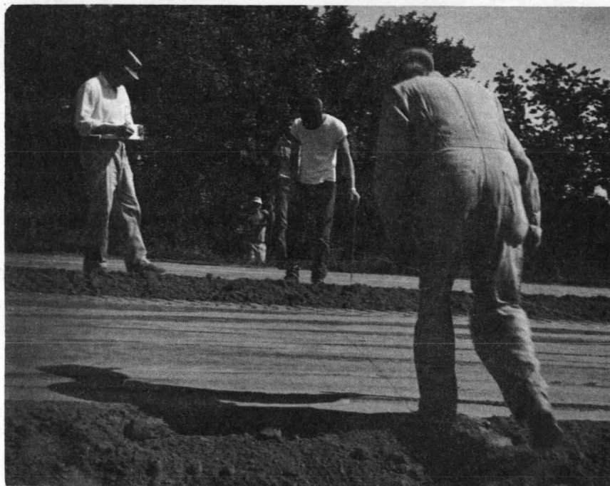
PHOTO 21: Checking crown during final shaping operation.
