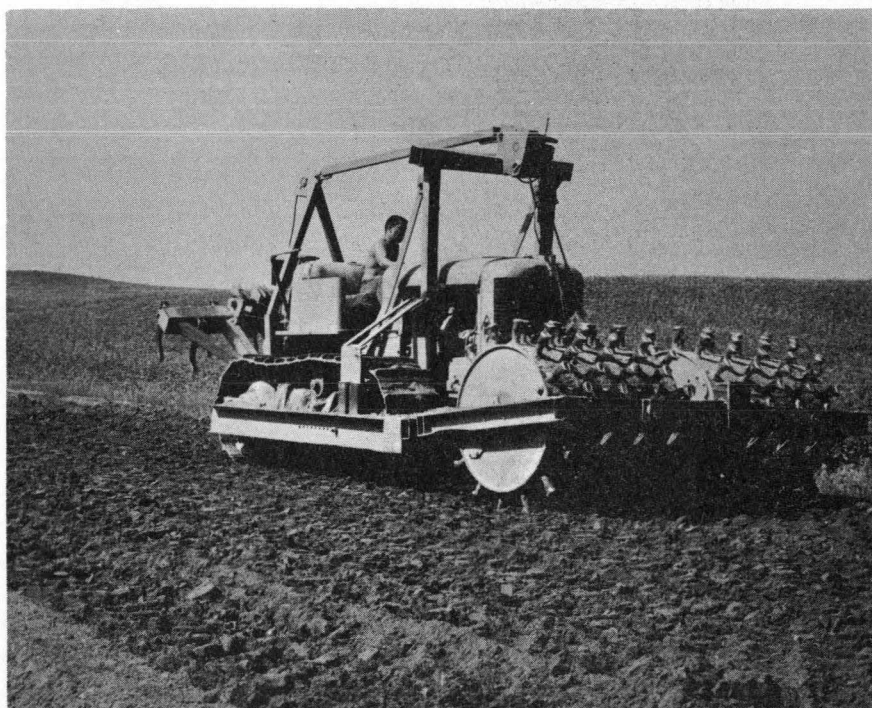
PHOTO 14: Sheepfoot roller making initial compaction.
