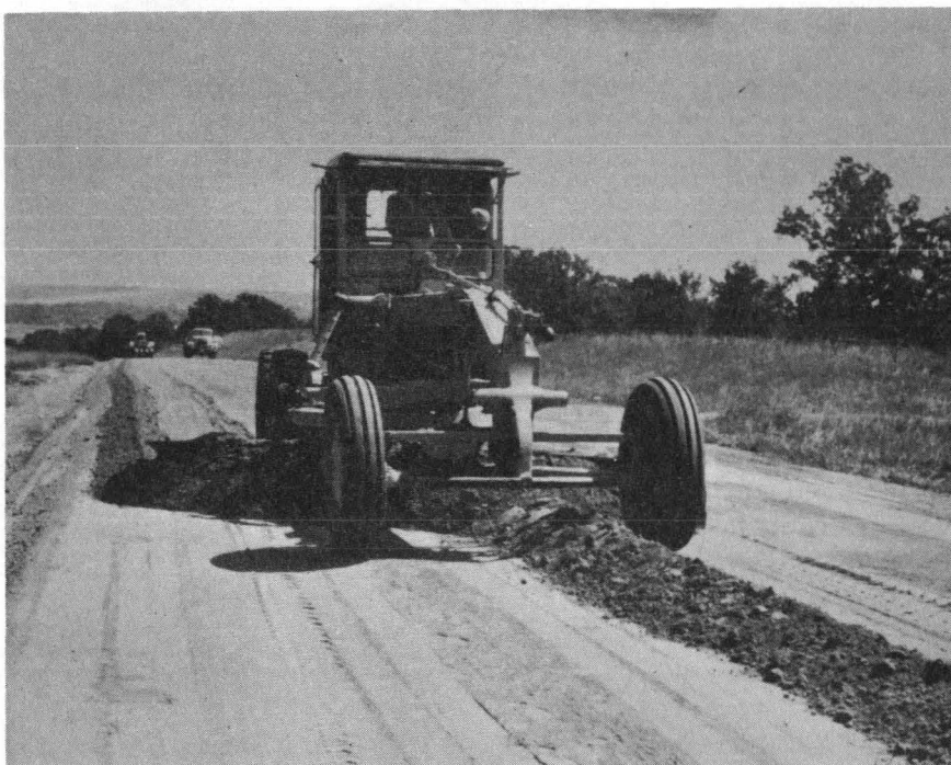
PHOTO 20: Motor grader shaping base prior to final compaction. Note large quantity of soil-cement carried by the blade. This material, which is approximately 2\frac{1}{2} hours old, had a tendency to separate from the rest of the base (See photo 24).
