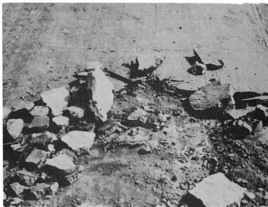
PHOTO 24: Separation of the top 3/4 inch of material from the rest of the base.
