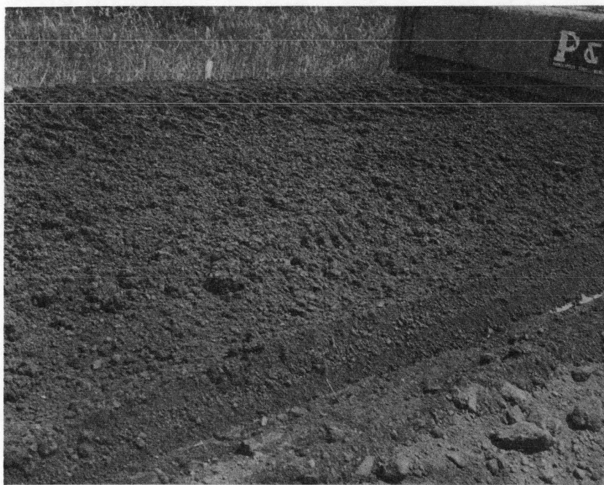
PHOTO 4: The arquad treated subbase after a single pass with the P & H machine.
