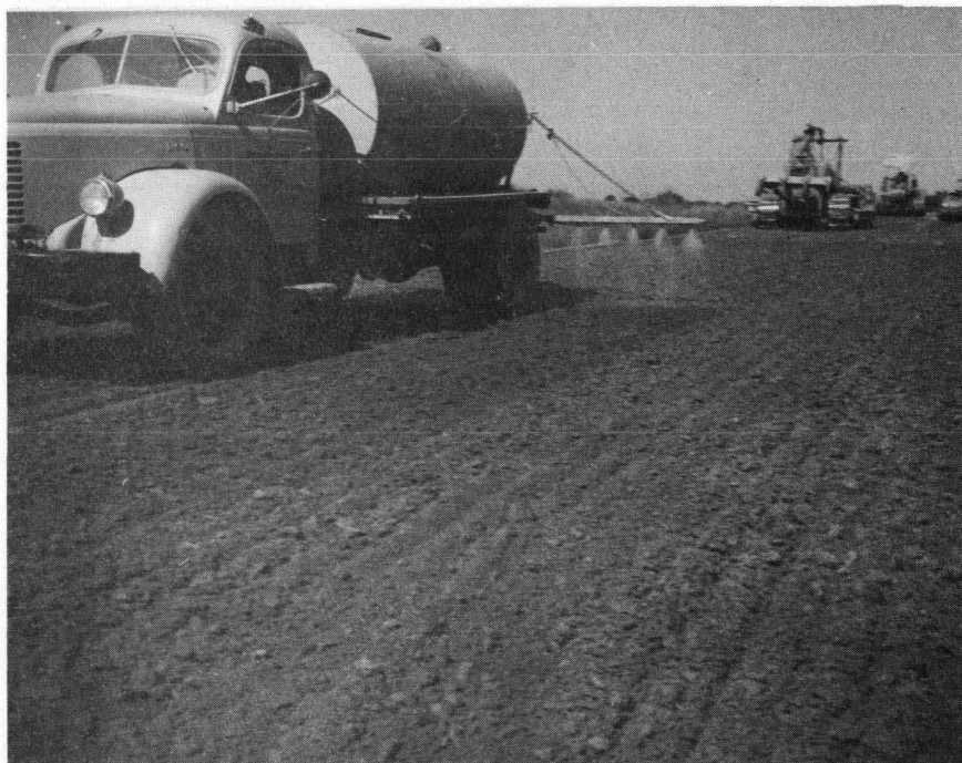
PHOTO 16: Applying water to the base following first coverage by the spike-drag.
