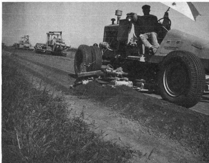
PHOTO 18: Lima Compactor compacting the edge.
