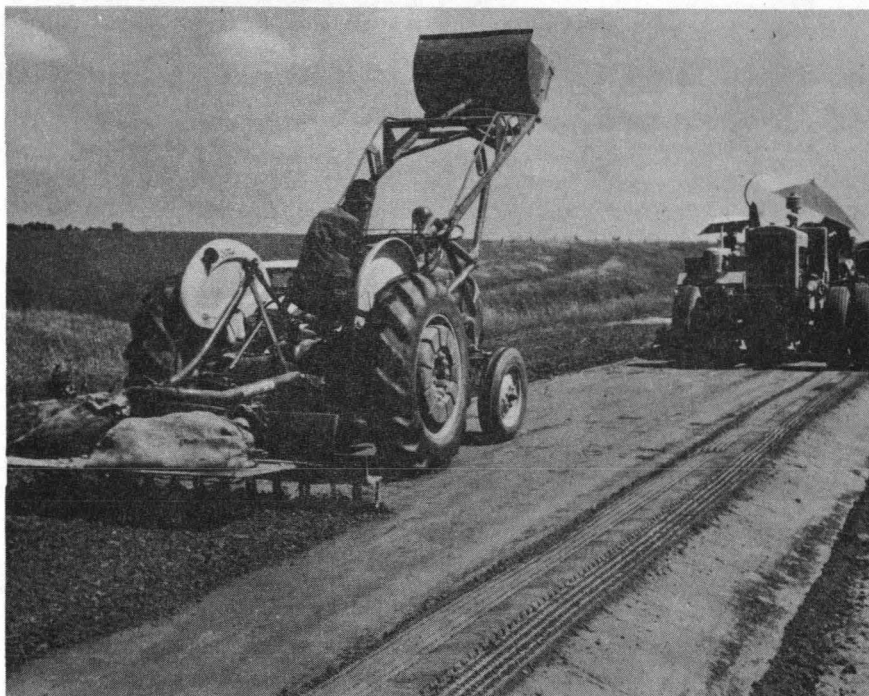
PHOTO 19: Second coverage by the spike-drag.
