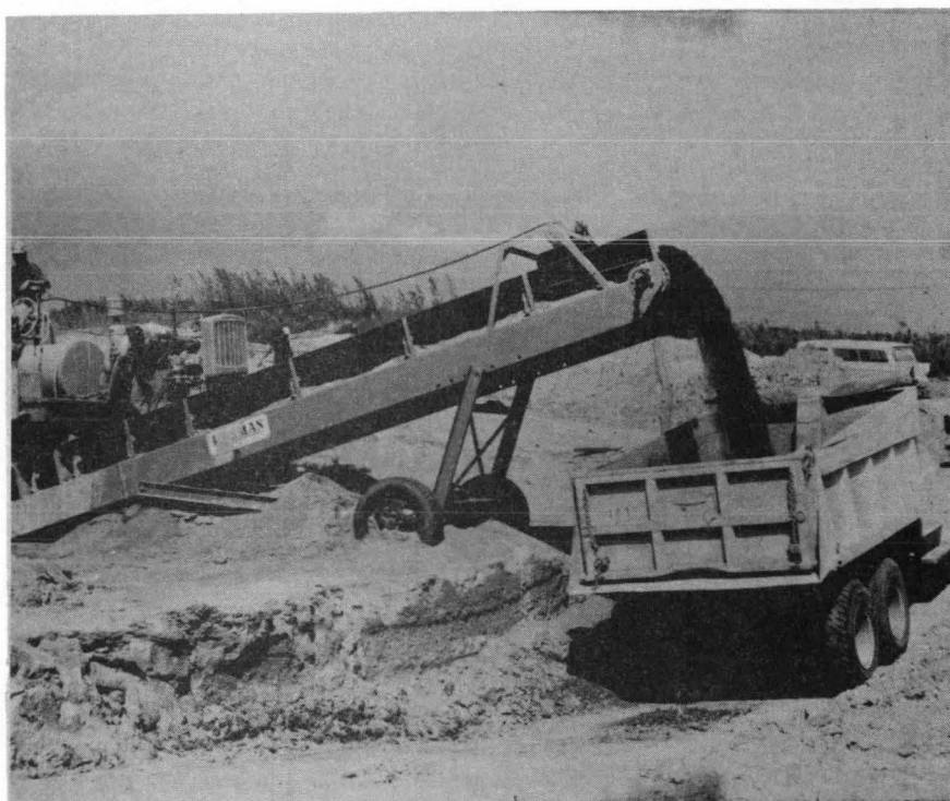
PHOTO 10: Loading soil-cement mixture.
