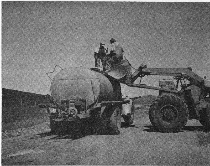
PHOTO 3: Adding Arquad 2HT to heated water. Circulation of the mixture was provided by the pump near the rear of tank.
