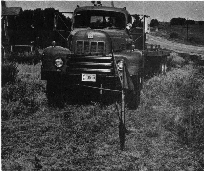
Photo 5: Test truck, showing tell tale guide for driver.
