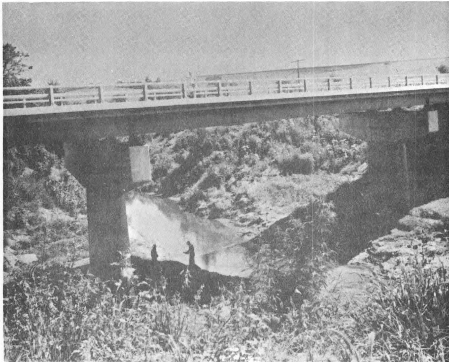
Photo 1: General view of the Silver Creek Bridge.
