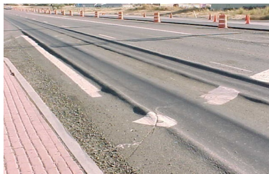
Figure 2.14. A Pictorial View of Rutting
