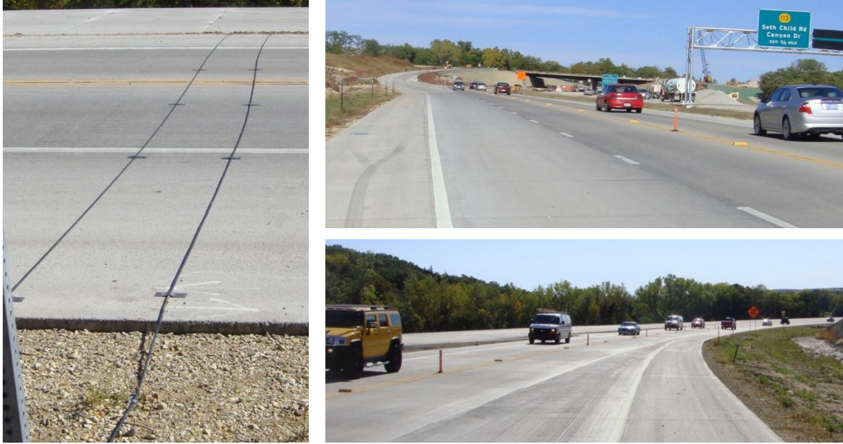
Figure 3.10. K-18 H-H EB and WB site setup photos
