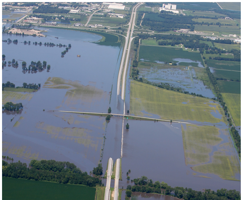
Closure of I-35 and US 30 for several days due to South Skunk River floods in and around Ames in 2010 (Image: ©James Moreland, retired from Iowa DOT Office of Motor Vehicle Enforcement)
