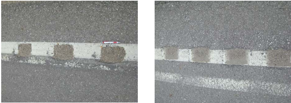
Figure 5-2. Rumble stripes filled with sand
