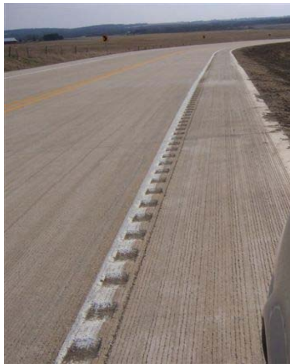
Figure 4-18. Rumble stripe installation on E-16
