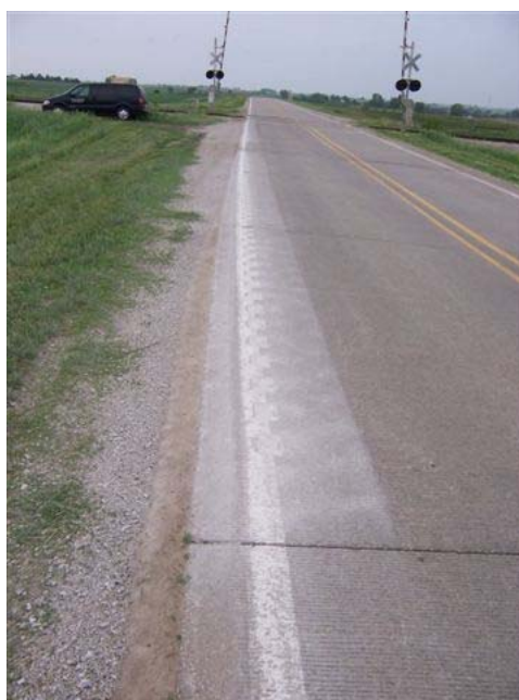
Figure 4-6. Rumble stripe installation on P-53
