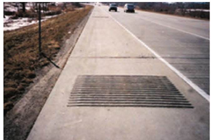
Figure 3.5. Formed-in shoulder rumble strips (Morena 2003)
