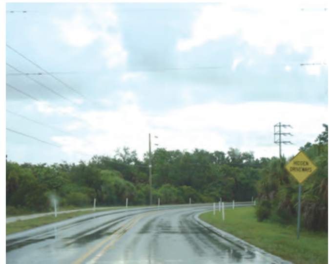
Figure 6.6. Post-mounted delineators in Captiva, Florida
