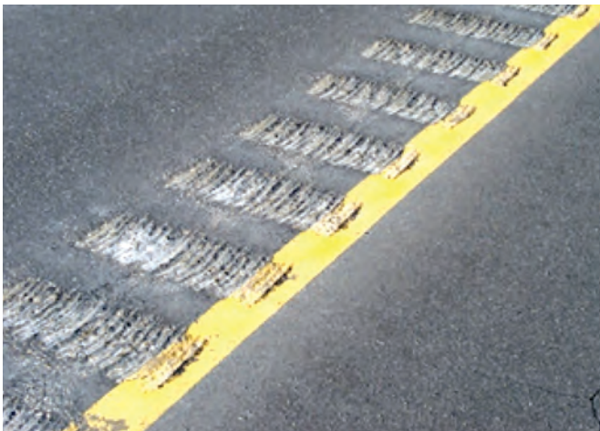
Figure 4.6. 18 inch CLRS in Iowa (Iowa DOT)
