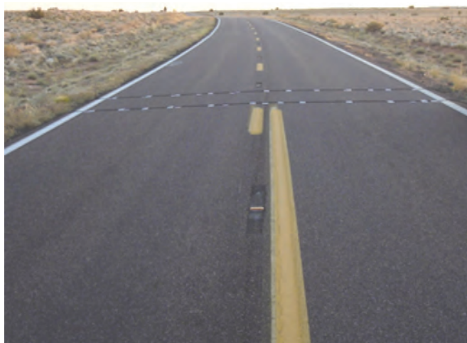
Figure 6.8. Raised pavement markers recessed into the pavement in rural Arizona
