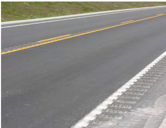
Figure 4.1. Continuous milled-in centerline rumble strips and edge line rumble strips on US Highway 34 near Creston, Iowa (Roche 2011)
