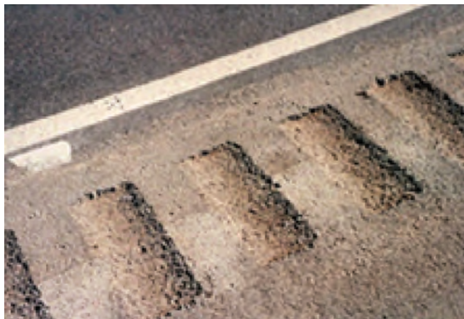
Figure 3.3. Milled-in shoulder rumble strips (Morena 2003)
