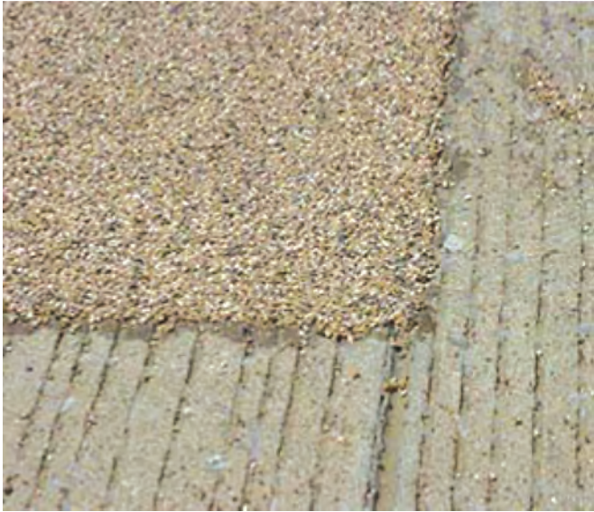
Figure 6.11. A high-friction surface treatment (Julian and Moler 2008)
