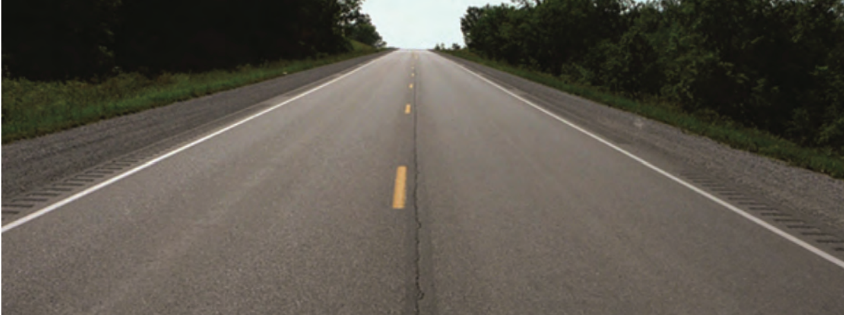
Figure 3.10. Continuous milled-in shoulder rumble strips on Iowa two-lane roadway with 2 foot paved shoulders
