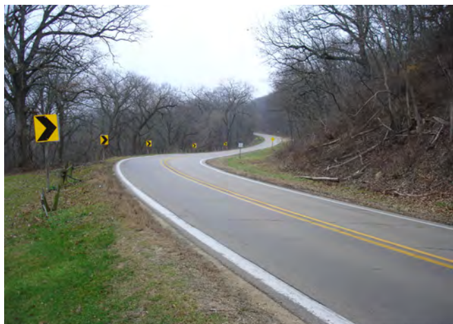
Figure 1.3. Typical earth unpaved shoulder
