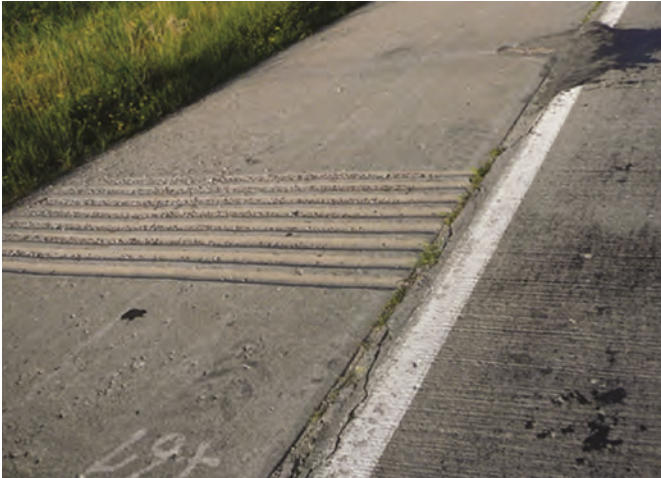
Figure 3.11. Formed-in PCC shoulder rumble strips on an Iowa highway
