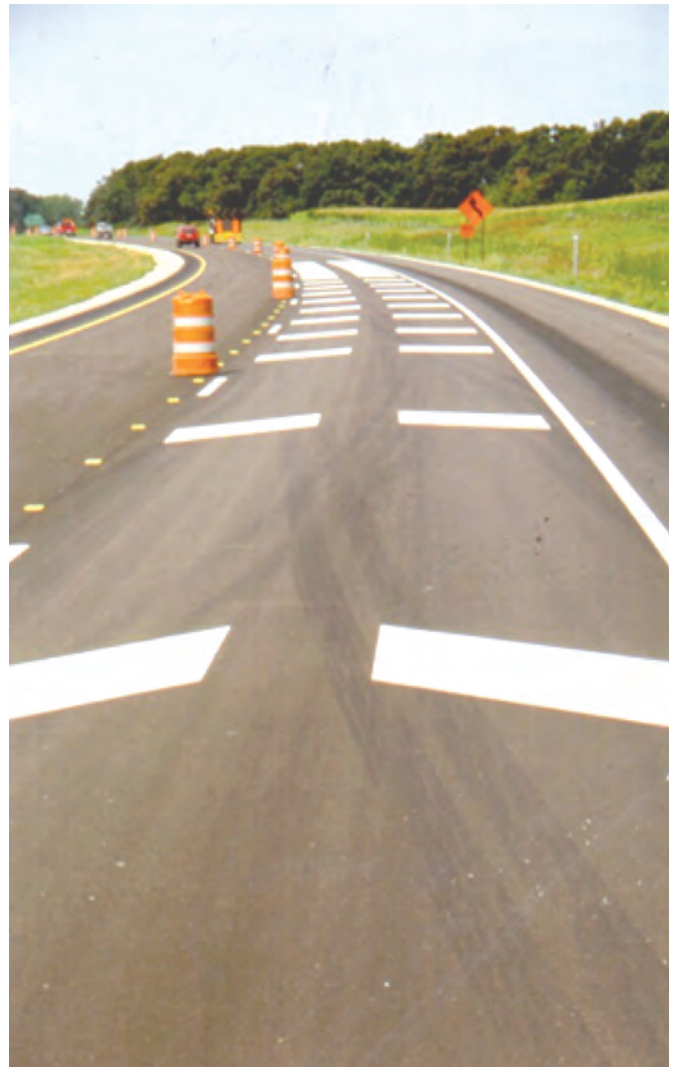
Figure 6.17. Mn/DOT "Tiger Tails" broken chevron pattern (Briese 2003)
