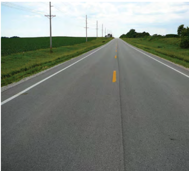
Figure 1.2. Two-lane highway with partially-paved shoulders
