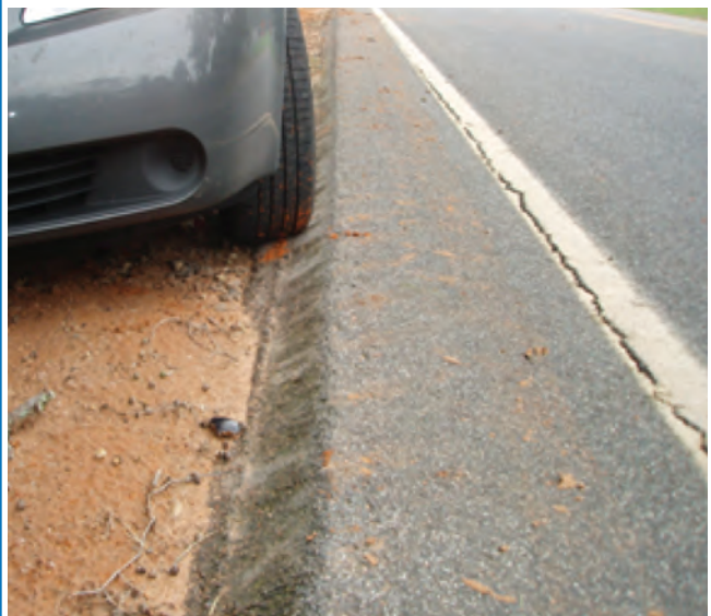
Pavement edge after resurfacing with Safety Edge
