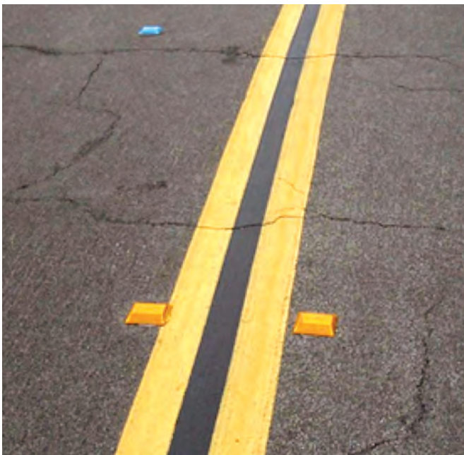
Figure 4.13. Raised centerline pavement markers (Intransition 2007)
