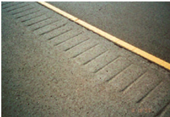
Figure 3.4. Rolled-in shoulder rumble strips (Morena 2003)
