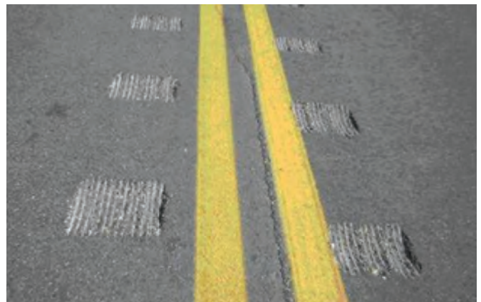
Figure 4.8. Continuous CLRS in Wisconsin on Highway 142 (Dulaski and Noyce 2006)
