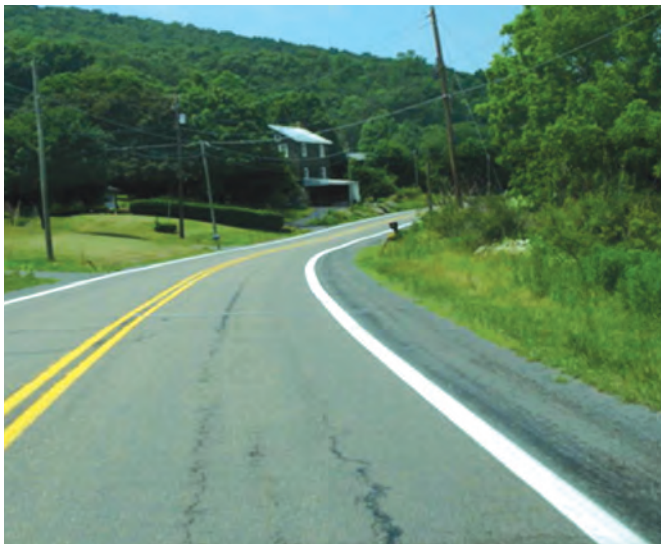
Figure 6.14. After 8 inch edge line treatment (Donnell 2006)
