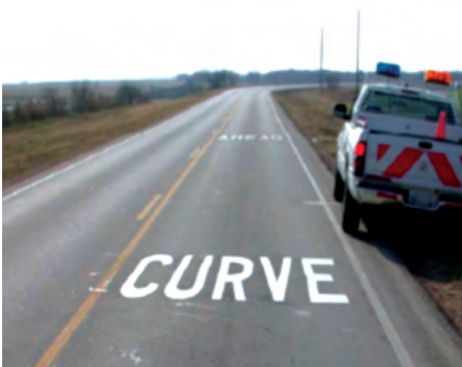
Figure 6.20. CURVE AHEAD in Texas (Chrysler and Schrock 2005)
