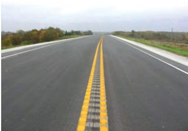
Figure 4.9. Continuous centerline rumble stripes (Stein and Neuman 2007)
