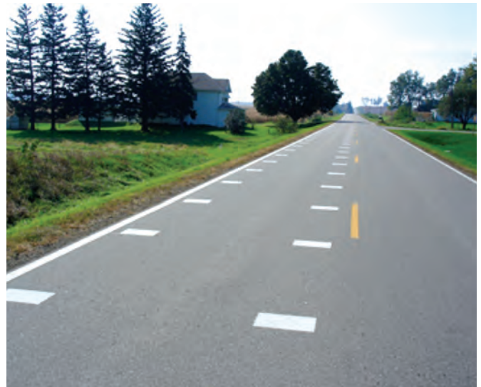
Figure 6.16. Transverse pavement markings as a rural gateway traffic calming treatment (Hallmark et al. 2007)
