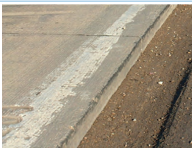
Typical vertical pavement edge on Portland cement concrete
