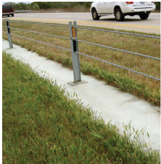
Figure 5.9. Mow strip for cable guardrails (WeedEnder®)
