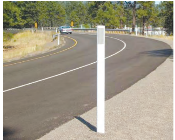
Figure 6.5. Flexi-Guide post-mounted delineators (Pexco)
