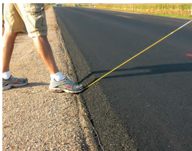
Figure 2.4. Pavement edge shape resulting from application of the Safety Edge
