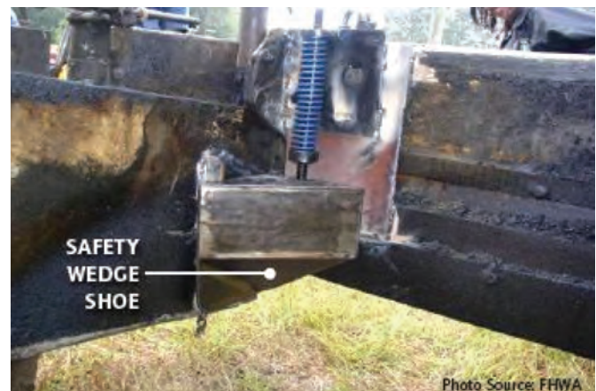
Figure 2.7. GDOT safety wedge hardware (FHWA 2009a)
