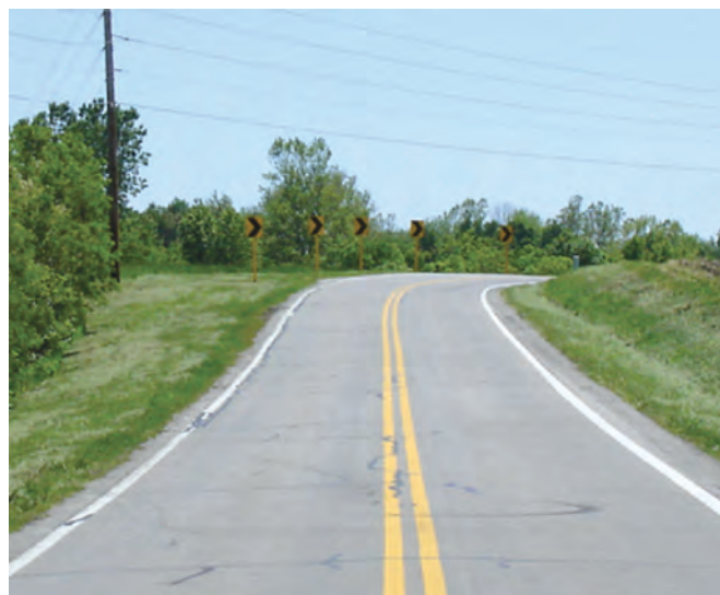
Figure 6.4. Chevrons with reflective post on a rural two-lane road in Ohio
