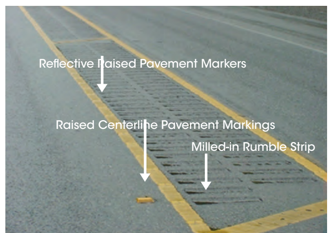
Figure 4.15. Painted median CLRS with raised thermoplastic edge line rumble strips and raised pavement marking lane guidance (Gray Notebook 2008)
