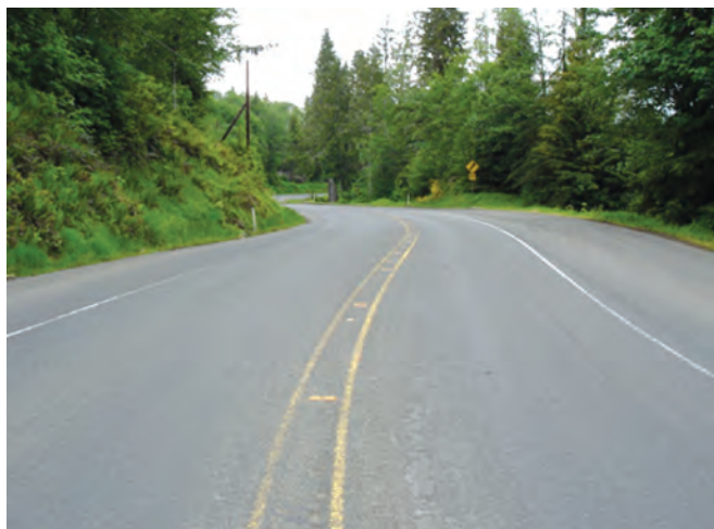
Figure 6.7. Typical raised pavement markers in the center of a curve in Washington
