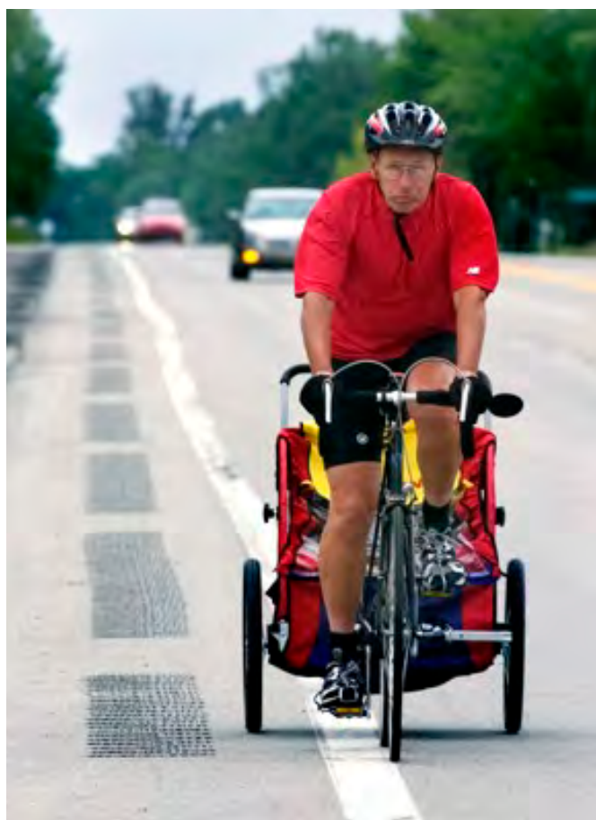
Figure 3.2 Bicyclist accommodation allows for travel between rumble strips without crossing over them (Cohn, Bay City Times ©2010 Michigan Live LLC)
