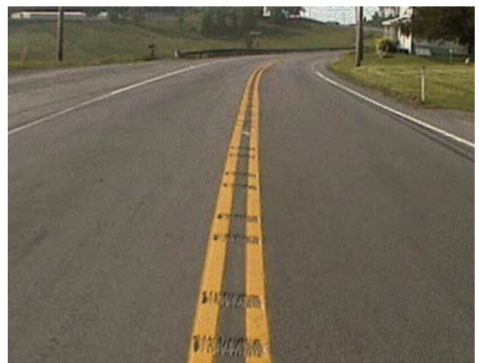
Figure 4.19. Gapped milled centerline rumble stripe pattern (Iowa DOT)
