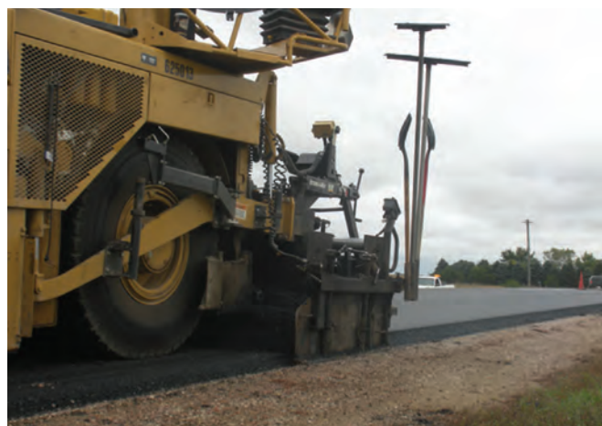
Figure 2.3. Application of the Safety Edge during resurfacing
