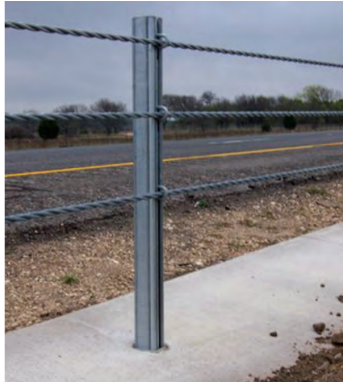
Figure 5.6. Gibraltar Cable Barrier Systems three cable system (Alberson 2006)
