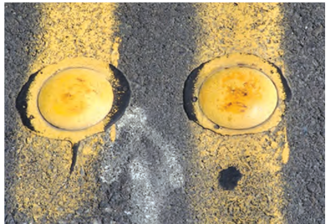
Figure 4.14. Caltrans raised pavement markers, "Botts' Dots"
