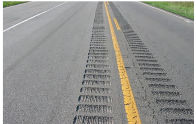
Figure 4.7. CLRS outside of pavement markings in North Carolina (Troy 2007)
