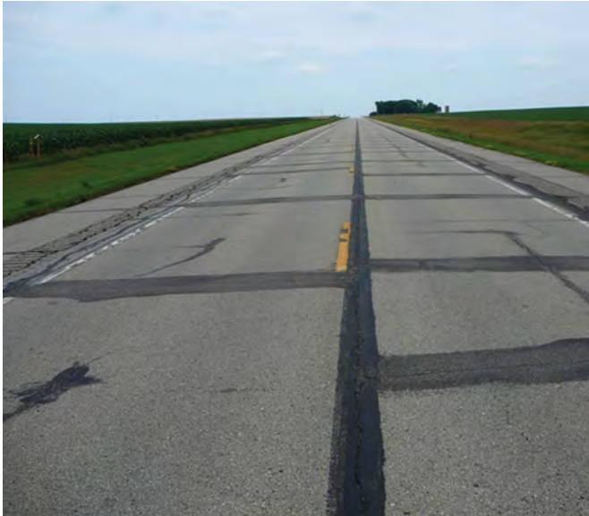
Figure 1.1. Two-lane highway with fully-paved shoulders
