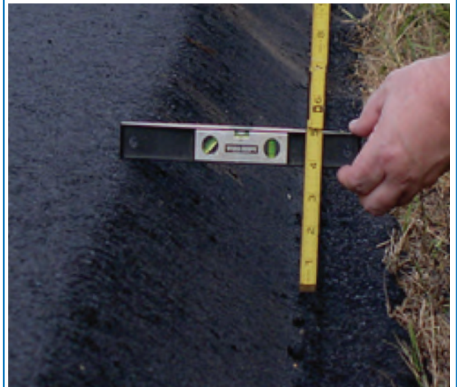
Pavement edge after resurfacing with Safety Edge
