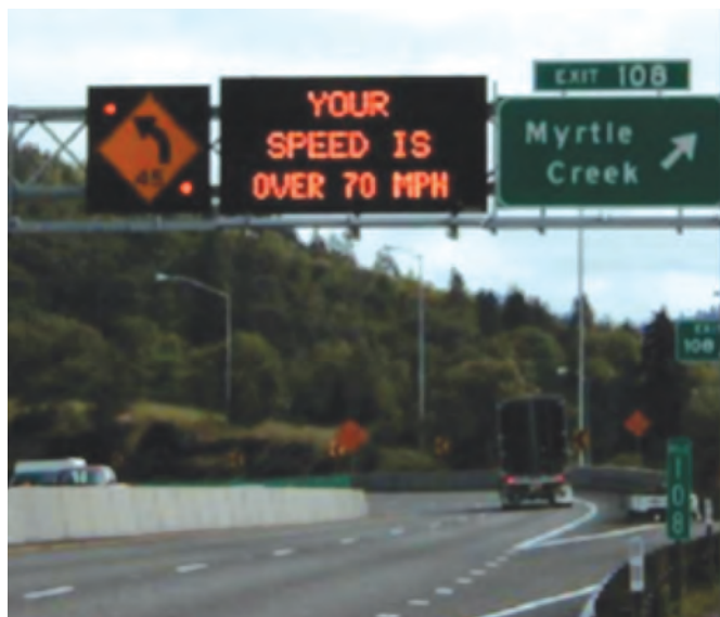
Figure 6.10. Overhead dynamic curve warning sign in Oregon (Bertini 2006)
