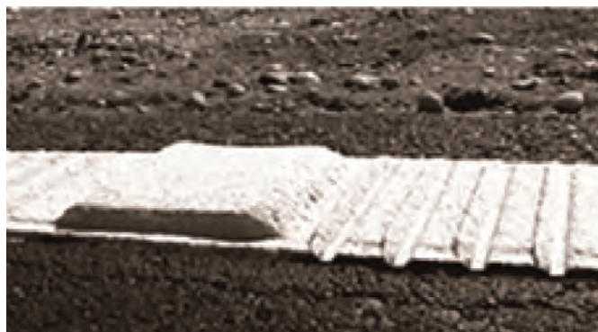
Figure 3.6. Caltrans raised (or inverted-profile) shoulder rumble strip made of thermoplastic (Neuman 2003)
