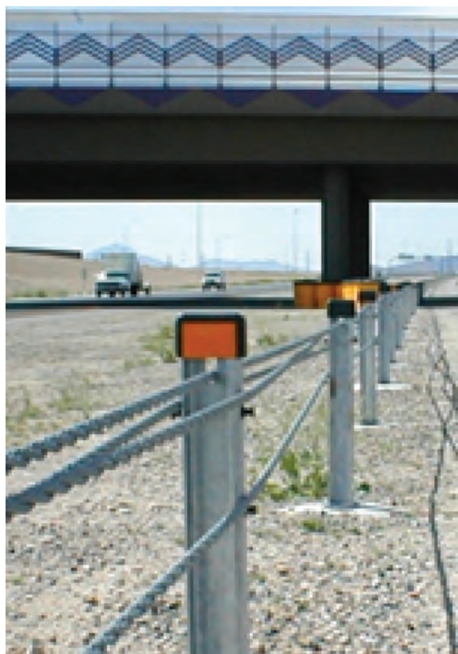
Figure 5.3. Brifen Wire Rope Safety Fence (WRSF) (Alberson 2006)
