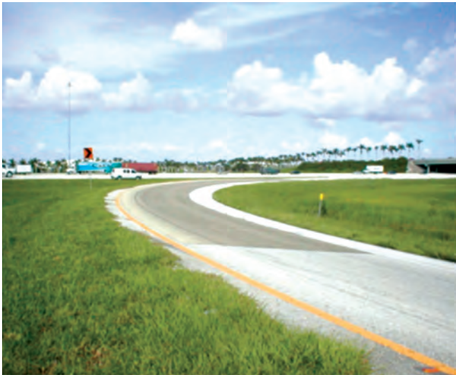
Figure 6.12: High-friction surface application area of I-75 northbound on-ramp from East Royal Palm Boulevard in Florida (Reddy et al. 2008)
