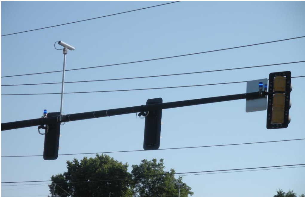
Figure 15. Confirmation Lights at University Avenue and Ansbrough Avenue in Waterloo, IA
