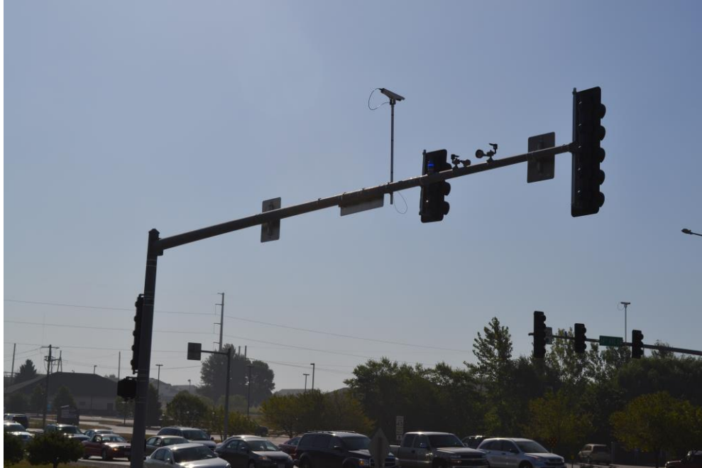
Figure 14. Confirmation Lights at 8 th Street and 34 th Street in Altoona, IA
