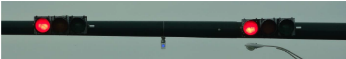
Blue Confirmation Light Mounted to a Mast Arm in Naples, Florida
