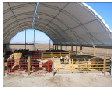
The prototype has three pens for cattle and a feed bunk that can be filled from outside.
