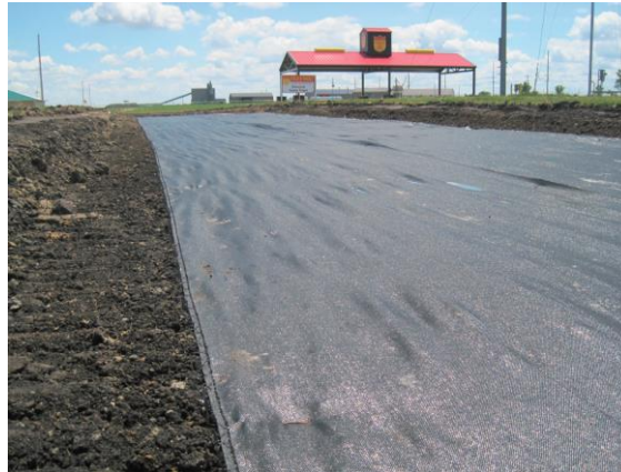
Figure 4. Woven geotextile placed in Boone County, Iowa (Boone County Expo research phase 1 – Granular road compaction and stabilization; InTrans project 12 – 433)
