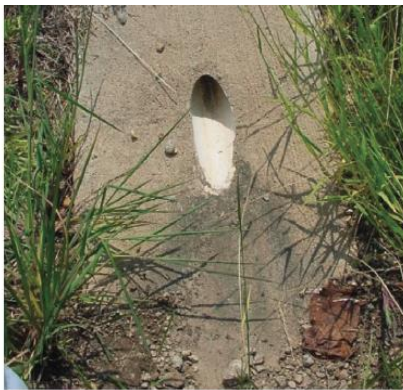
Figure 6. Rural subdrain outlet (Photo courtesy of Chapter 7, Concrete Pavement Preservation Guide, CP Tech Center)
