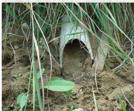
Figure 7. Clogged subdrain outlet (Photo courtesy of Chapter 7, Concrete Pavement Preservation Guide, CP Tech Center)
