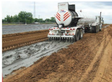
Figure 2. Cement slurry application (Photo courtesy of Guide to Integrated Pavement Solutions, CP Tech Center)
