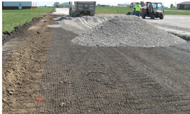
Figure 3. Rectangular geogrid placed in Boone County, Iowa (Boone County Expo research phase 1 – Granular road compaction and stabilization; InTrans project 12 – 433)
