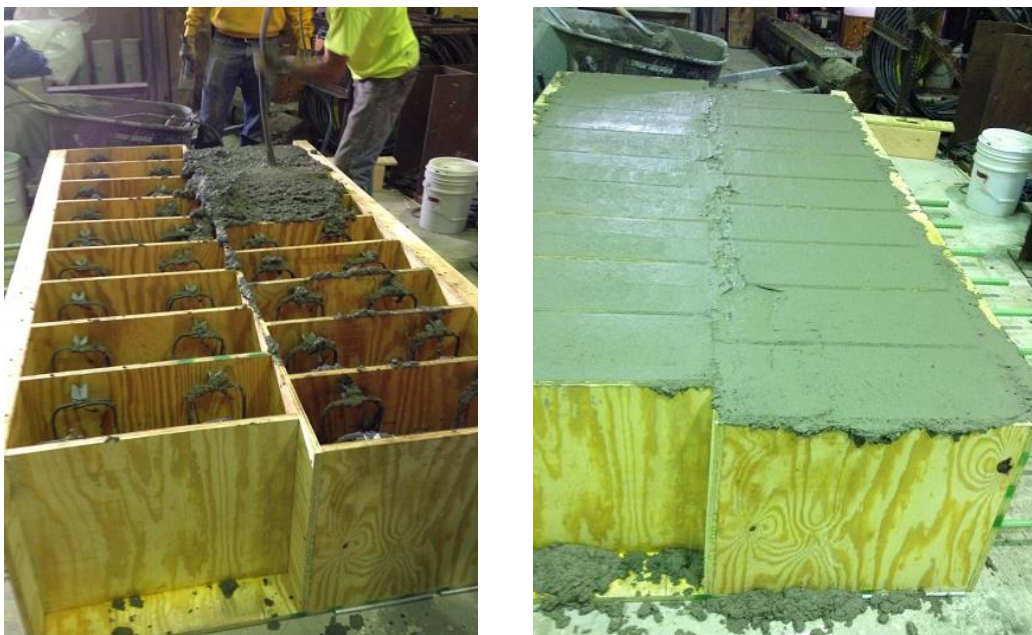
Figure 3-3. Concrete cast into the wooden forms
