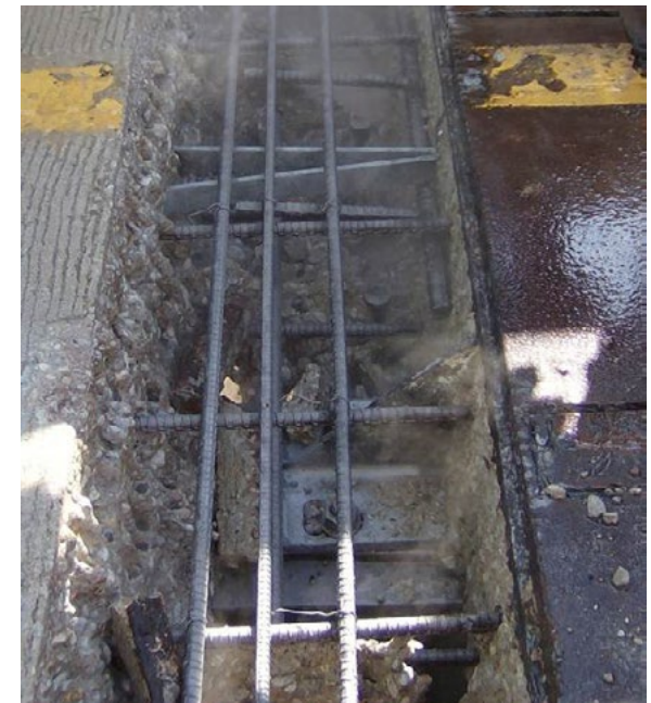
A sliding plate deck expansion joint being replaced using hydrodemolition technique.
