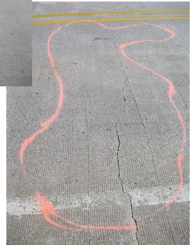
Photographic documentation of delamination is shown in these images.
