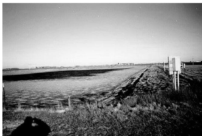
Geotextile cover with straw on Minnesota swine lagoon.
