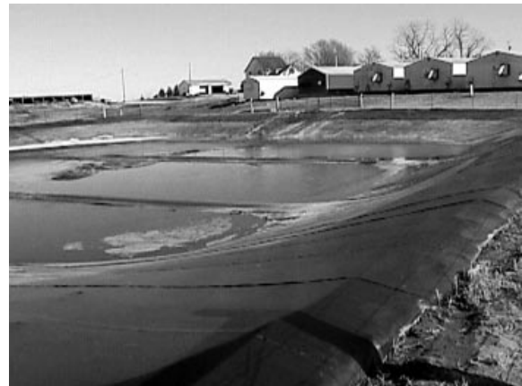
Figure 3. Floating plastic cover on earthen pit.
